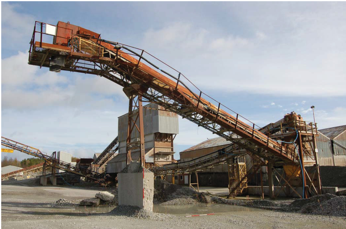
Plate 24: Stockpile Conveyor [18], NT SMR 54,217. View from south-west.
