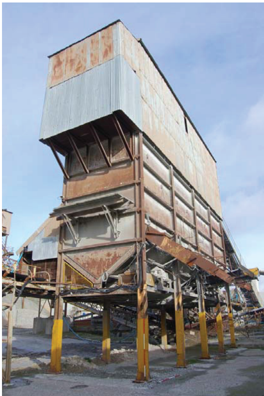
Plate 19: Grading Plant [13]. NT SMR 54,212, view from SW.
