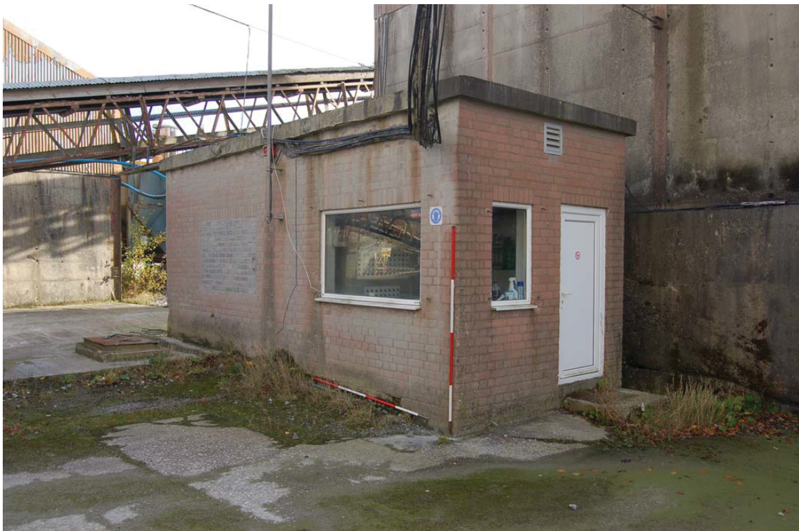
Plate 13: Building [8], 'Switch House B': NT SMR 53,207 . View from west.
