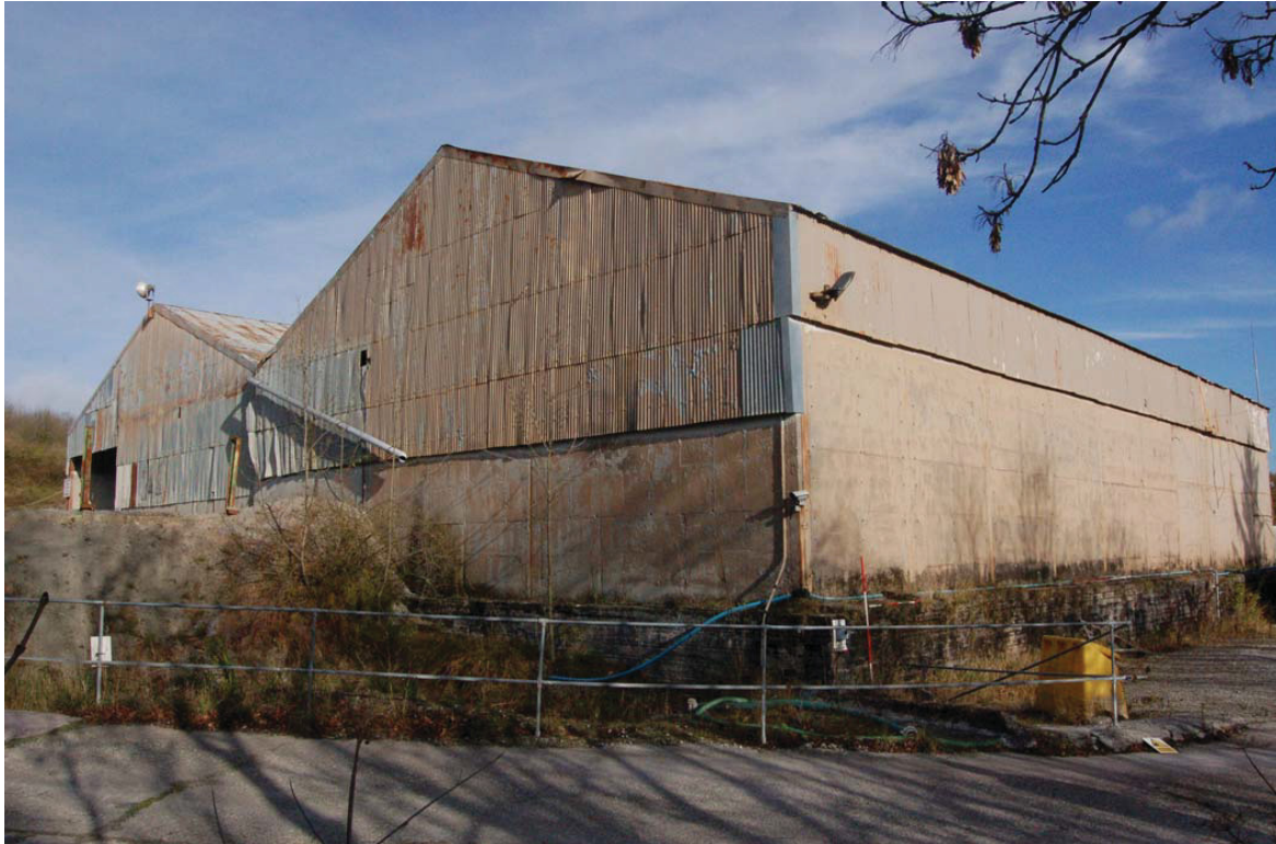
Plate 8: Building [5], 'Stock B Coating Plant': NT SMR 54,204 . View from south-west.
