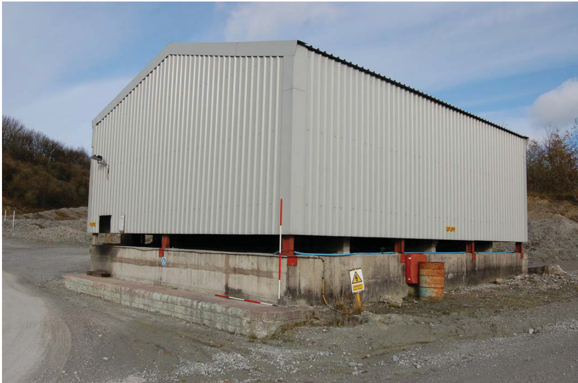
Plate 35: Oil Tank Store [26], NT SMR 54,225 . View from south-west.
