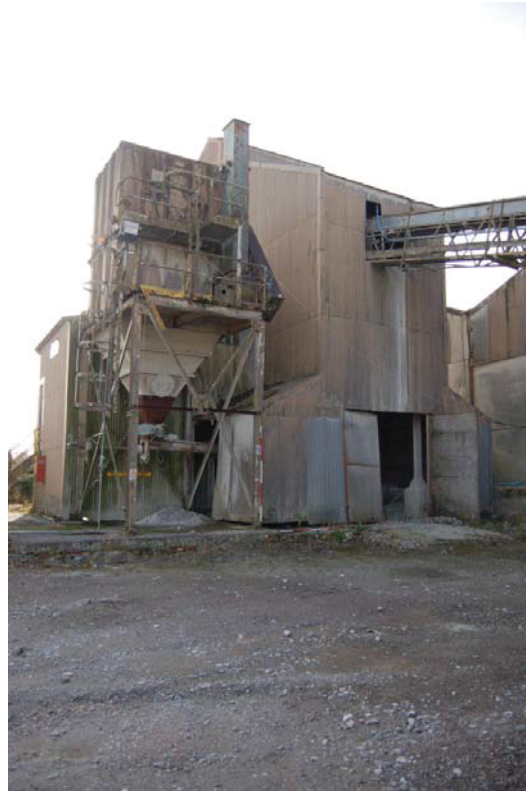
Plate 6: Building [4], 'Lanway 4 Crusher' NT SMR 54,203. View from NE.
