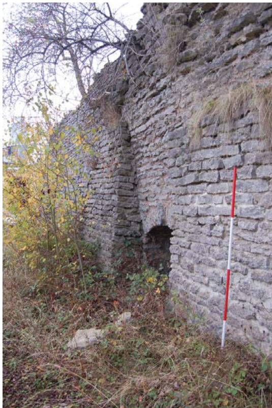
Plate 43: Detail of draw-hole and buttressing.
