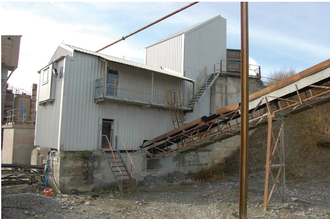
Plate 28: 'Primary Crusher' [22], NT SMR 54, 221 . View from east.
