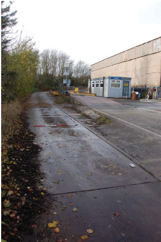
Plate 12: Building [7], Weighbridge. NT SMR 53,206 View from north-east.
