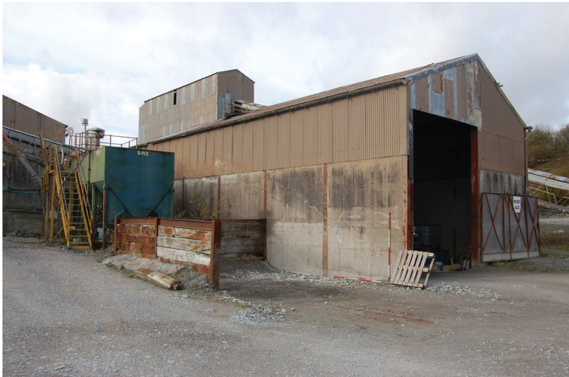
Plate 17: Building [12], 'Multicrete Balast Shed': NT SMR 53,211 . View from SE.
