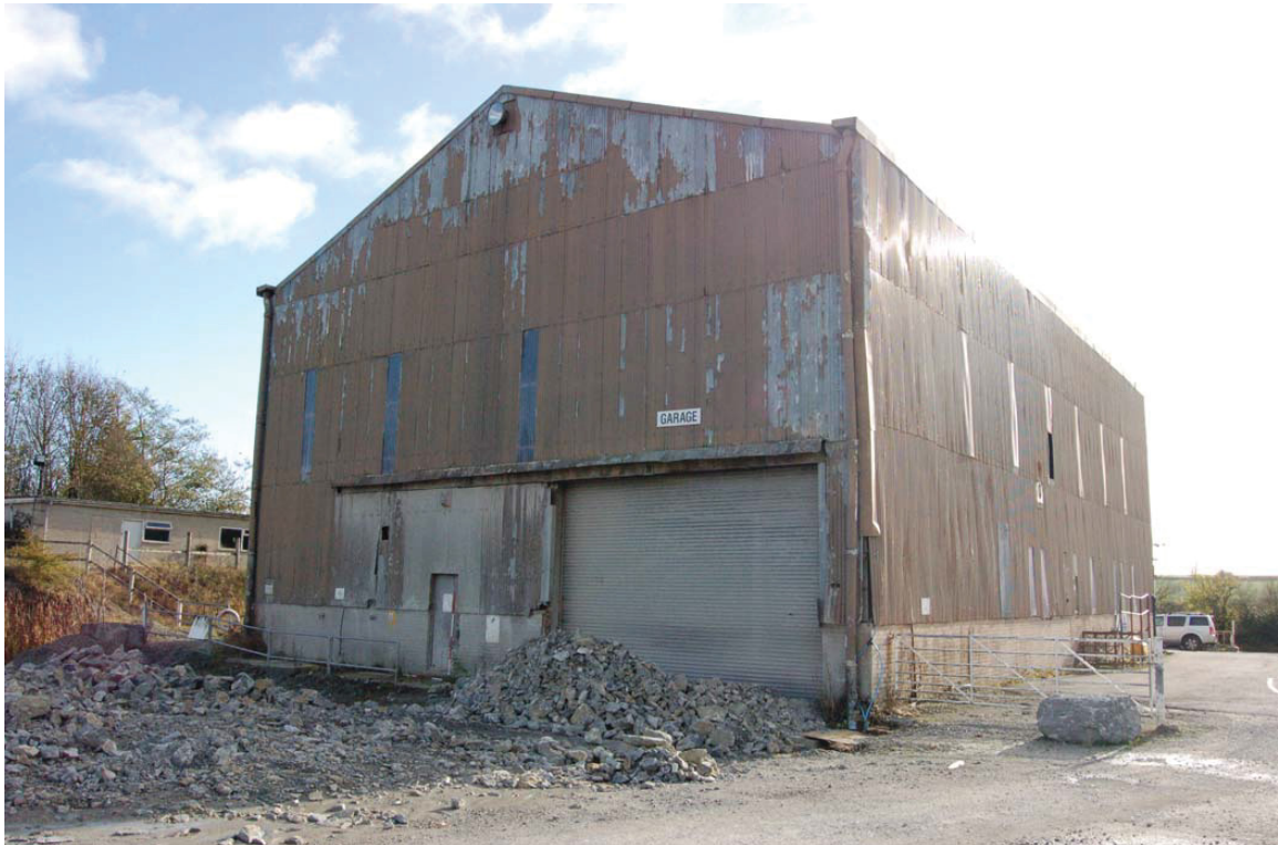
Plate 2: Garage [1]: NT SMR 54,200 . View from north-west.
