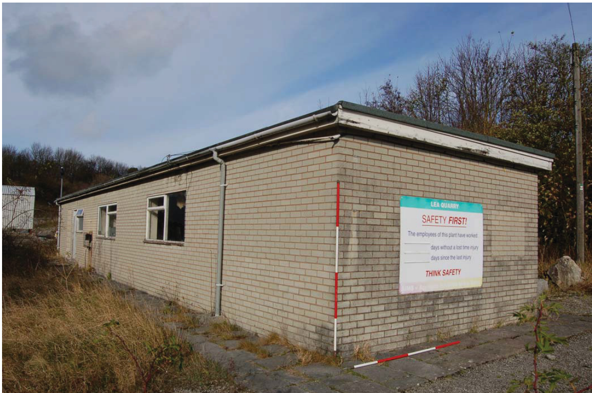
Plate 36: Toilet / Mess Room Block [27], NT SMR 54,226 . View from south.
