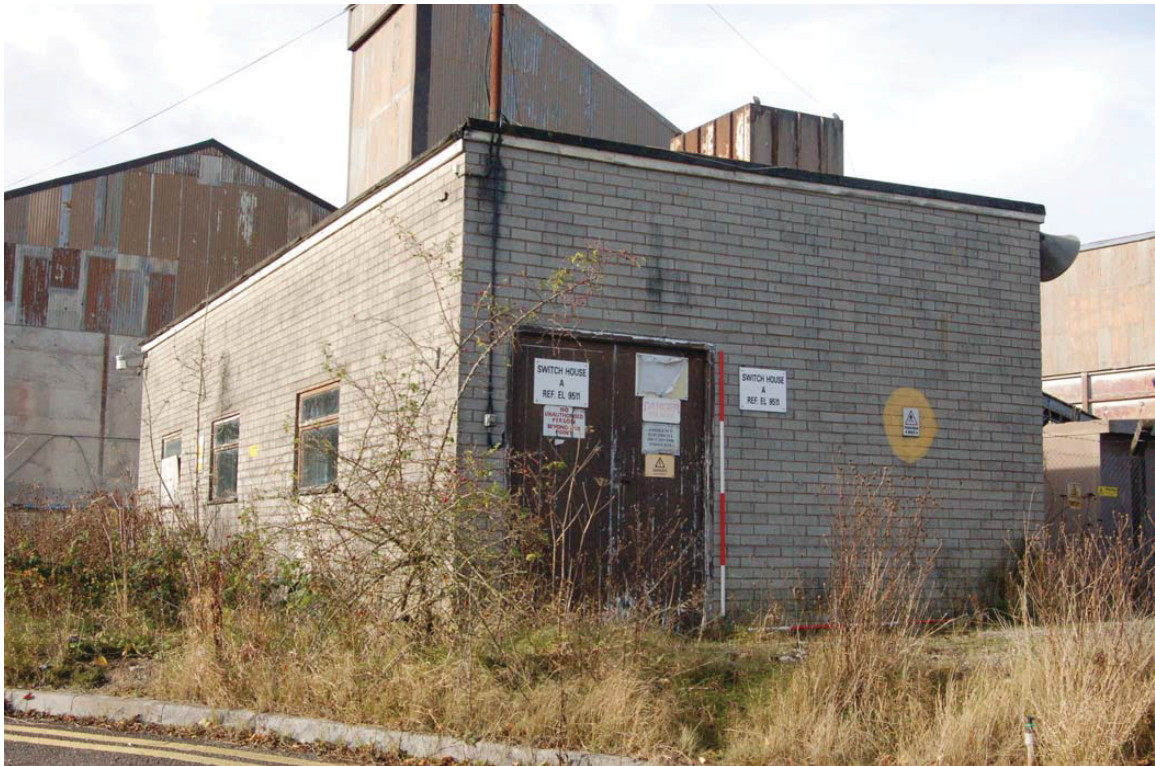
Plate 4: Building [3], 'Switch House A' : NT SMR 54,202 . View from east.
