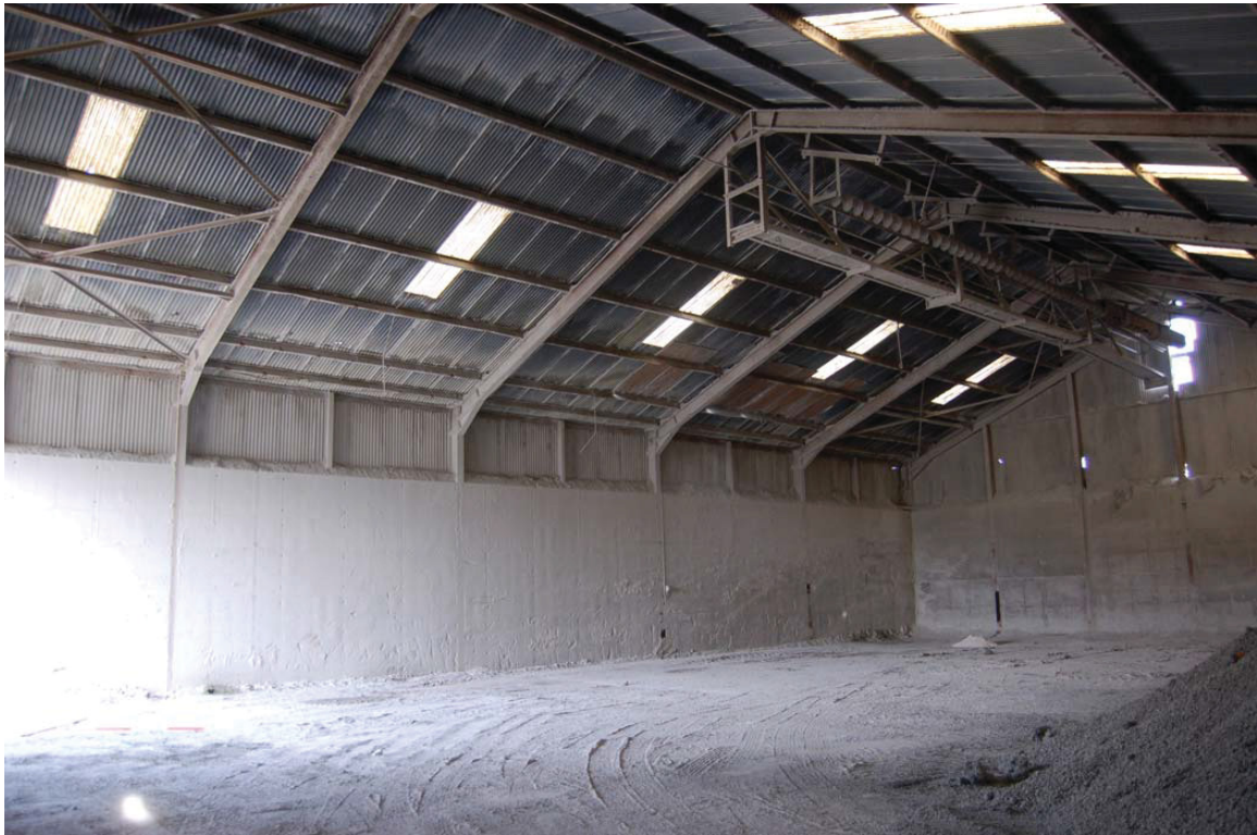
Plate 10: Building [5], 'Stock B Coating Plant': NT SMR 54,204 . Interior, north range.
