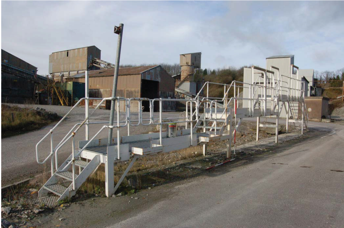
Plate 3: Raised walkway [2]: NT SMR 54,201 . View from south-east
