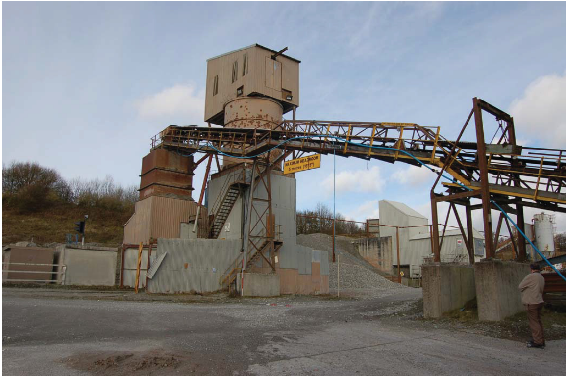
Plate 25: Long Conveyor [19] (NT SMR 54,218) to Brick Surge Bin [33] (NT SMR 54, 232).
