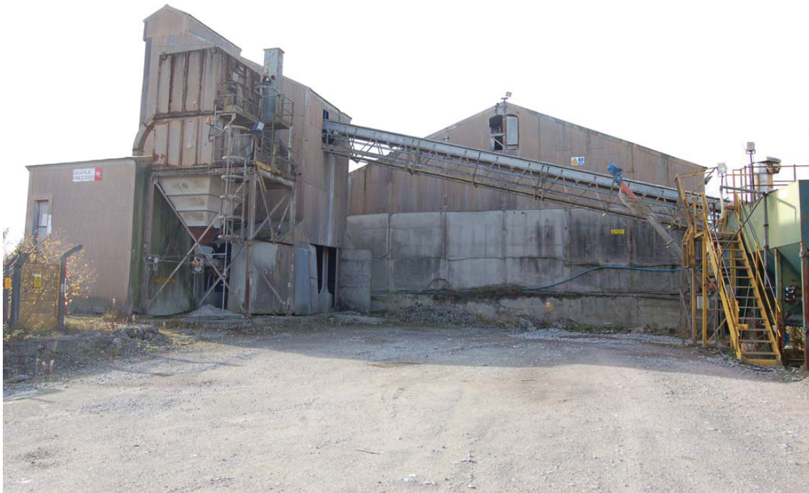
Plate 14: Building [9], 'Lime Plant Feeder No.2 Conveyor' ; NT SMR 54, 208 (centre), feeding into Lanway 4 Crusher (left), Coating Plant B to rear. View from north-east.
