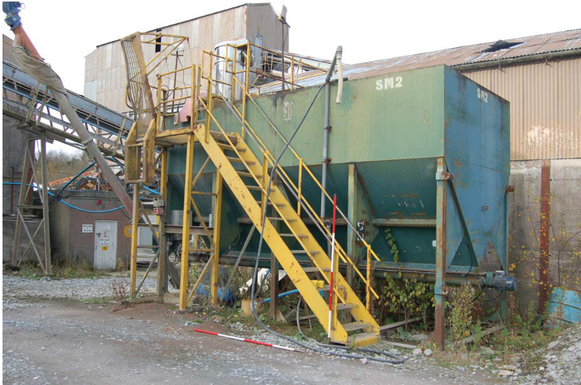
Plate 16: Cement Tank [11]: NT SMR 53,210 . View from south-east.
