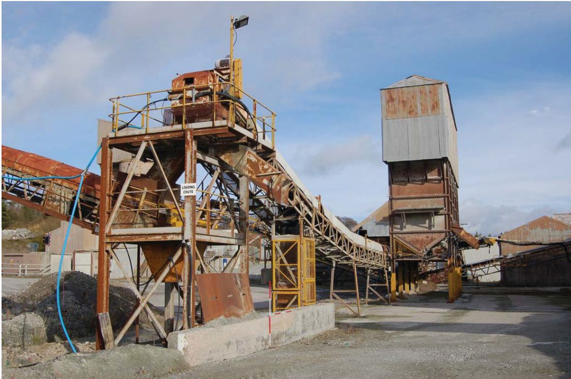
Plate 18: Grading Plant [13] (right), Batching Conveyor [16] and Loading Chute [17] (left), view from SW.
