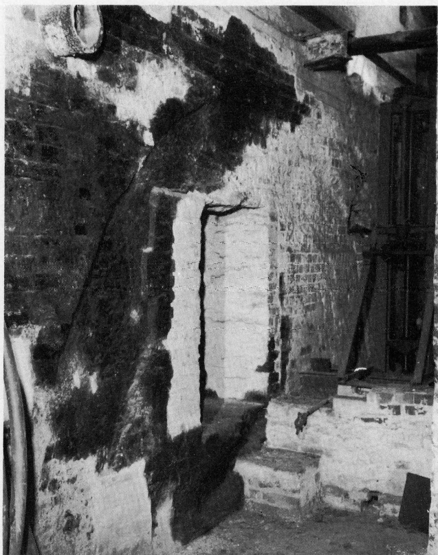
Plate 17 Scuff marks made on a wall by one of the water-wheels
