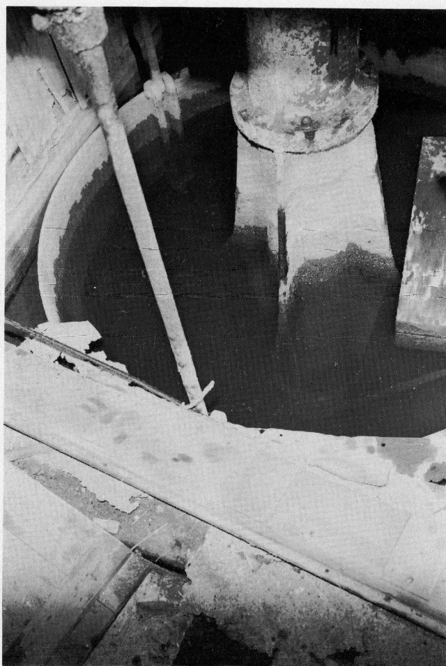
Plate 18 The Fourneyron-MacAdam water-turbine from above showing portions of the stator and the gate (see Fig. 21)
