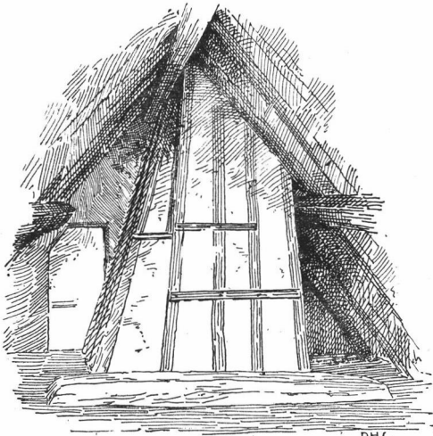
THE CHIMNEY IN THE ATTIC SOUTH SITCH
