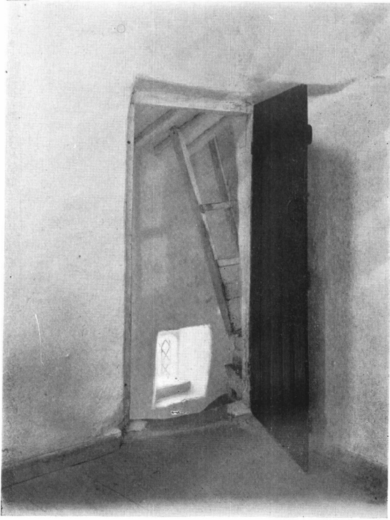
TOP OF STAIR IN UNDIVIDED HOUSE.
