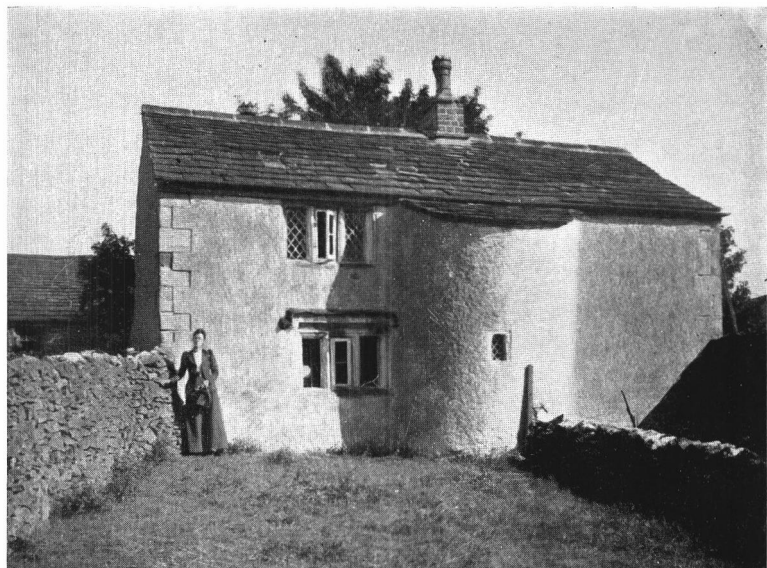
THE UNDIVIDED HOUSE (FROM THE SOUTH).
