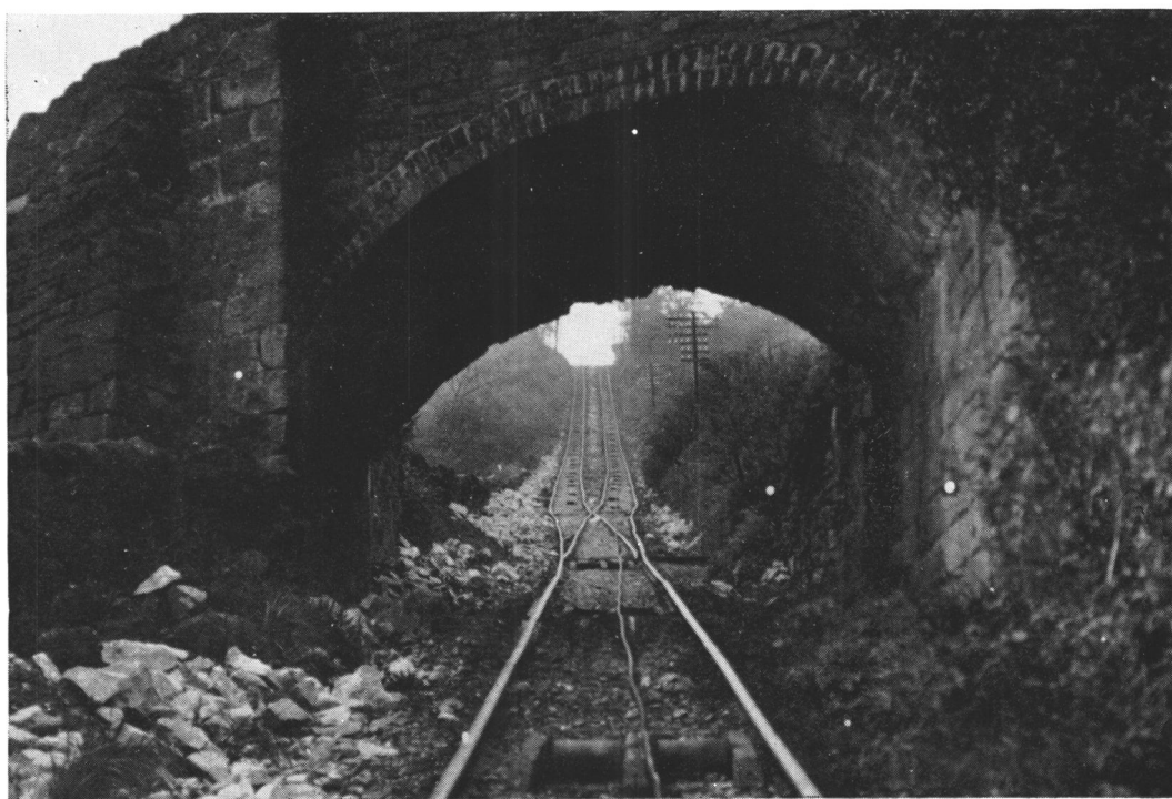
b. George Stephenson's gravity operated incline for limestone wagons, Bull Bridge.
