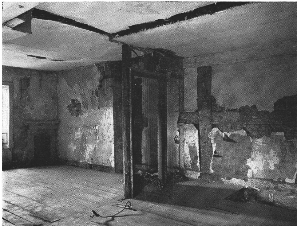
a. Upper part of the medieval stud partition during restoration.
