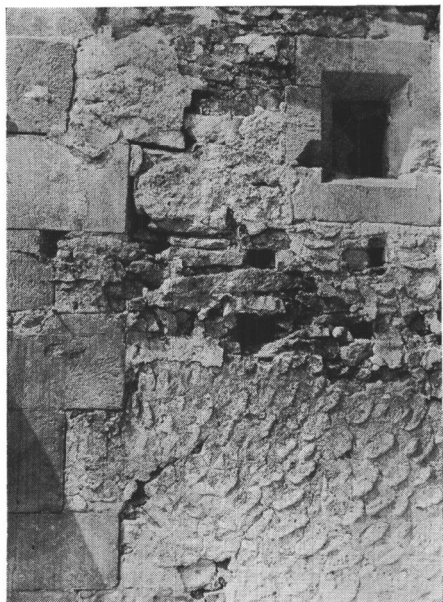
a. Small medieval window and oyster shell pargetting.
