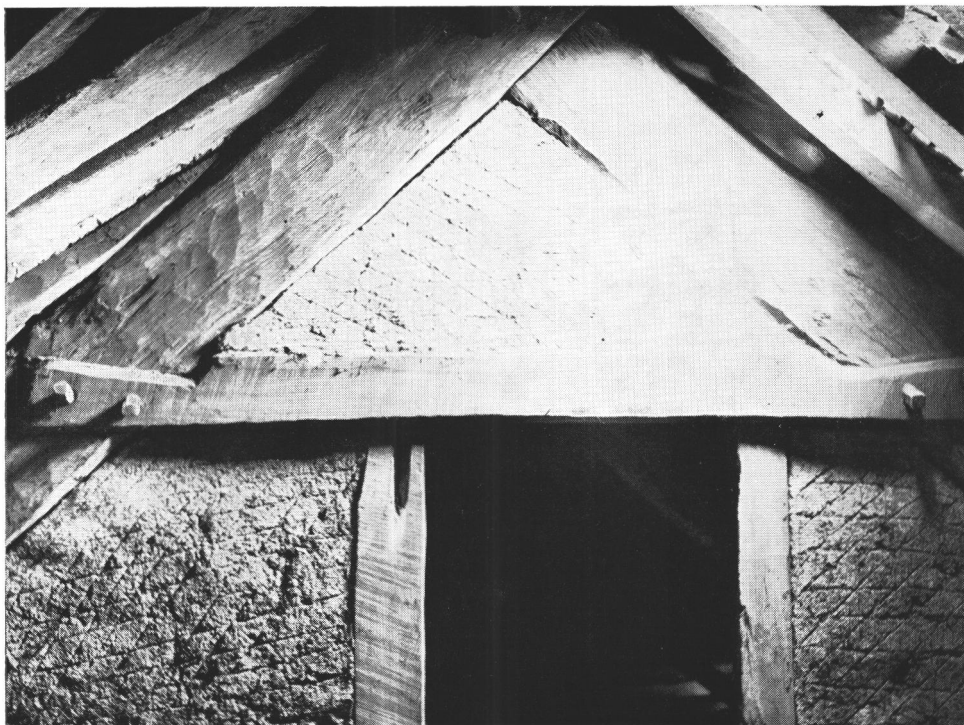
a. Hatch to the roof chamber over the buttery.
