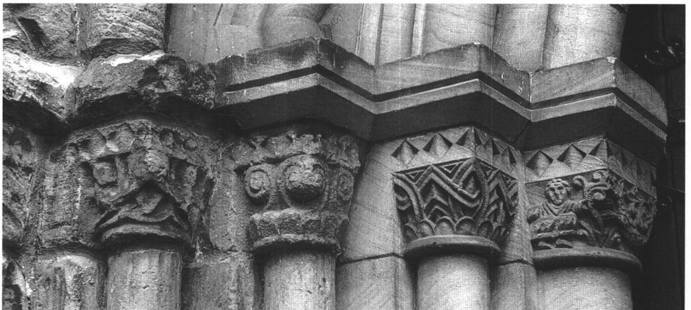
Plate 27: Capitals of the west doorway, left side.
