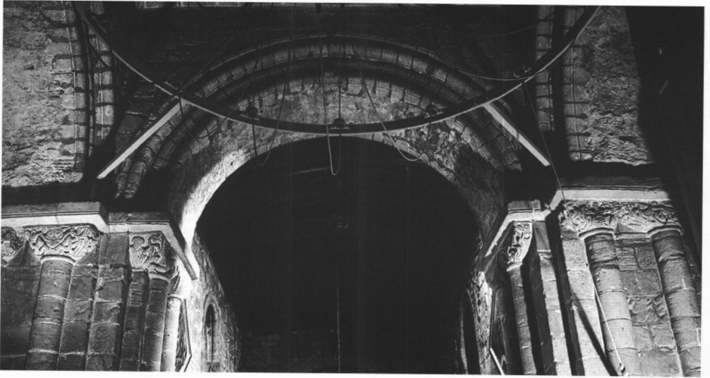
Plate 29: View of the main scheme from the crossing.
