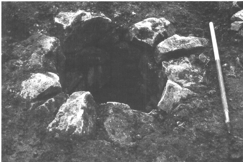
Plate 1: Dry-stone lined (ginged) shaft at Dene Quarry, Cromford. Photo by Duncan Alexander. ©ARCUS
