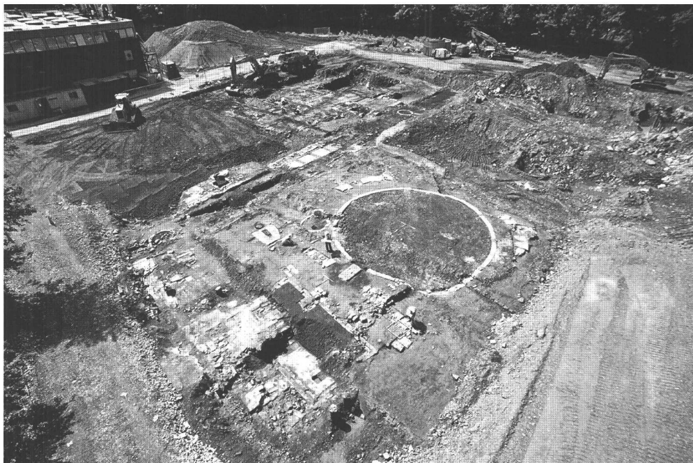
Plate 5: Excavations at Milford Foundry, Milford. The remains of the retort house and gas holder of the gas works are in the foreground. Photo by Aerial Close-Ups. ©ARCUS.
