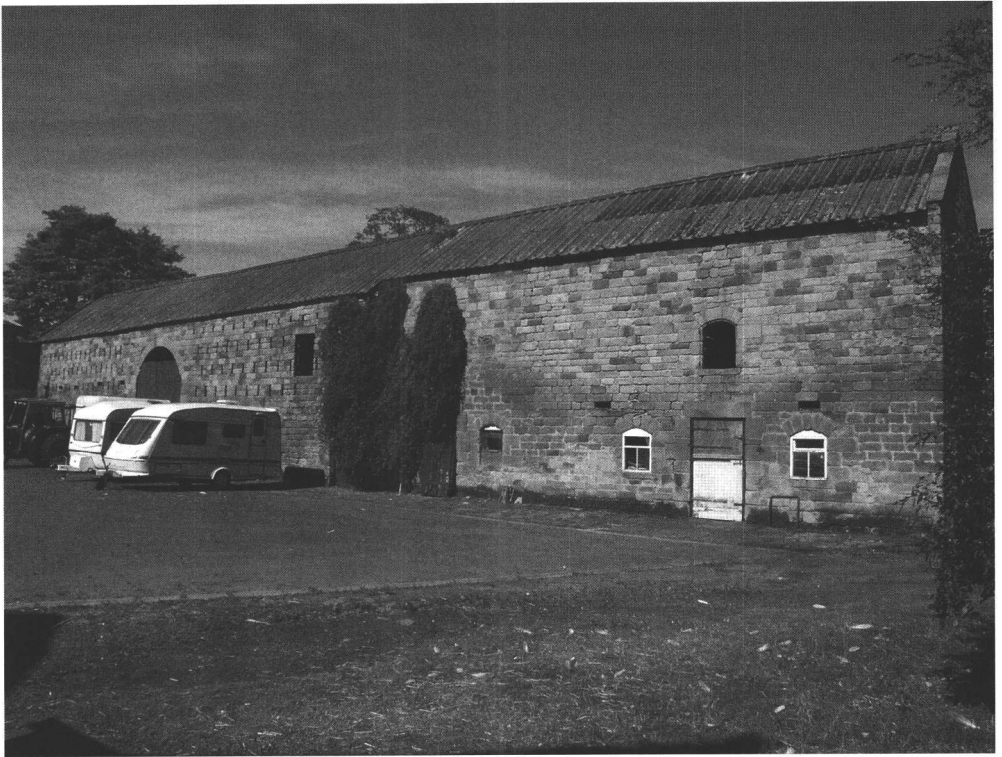
Plate 7: Elms Farm, Little Eaton: west frontage of the barn range, with the barn to left and the added stable to right.
