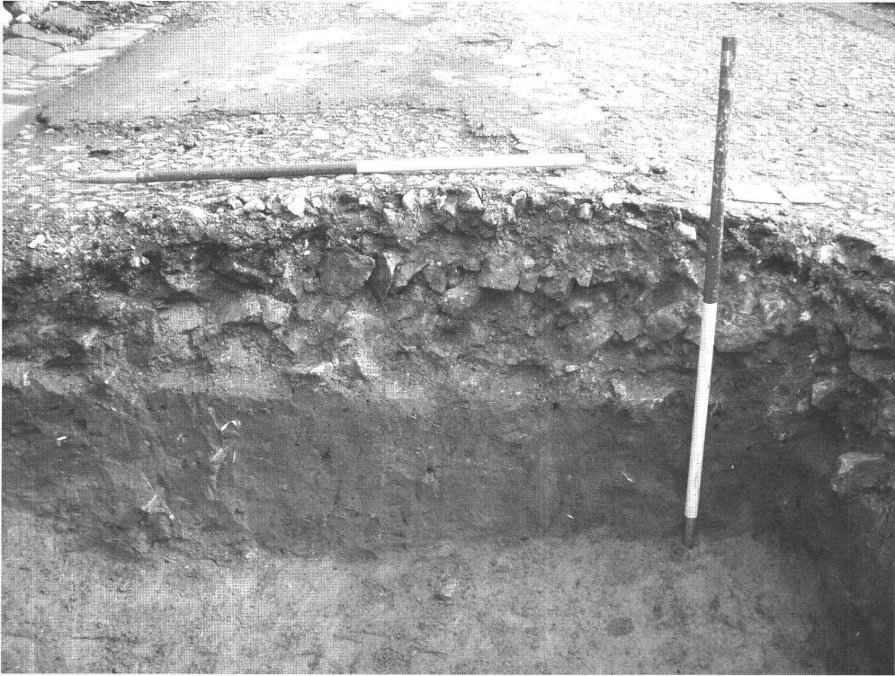
Plate 1: Belper: section showing the make-up of the 19th century road surface in George Street. Photograph by D. Walker.
