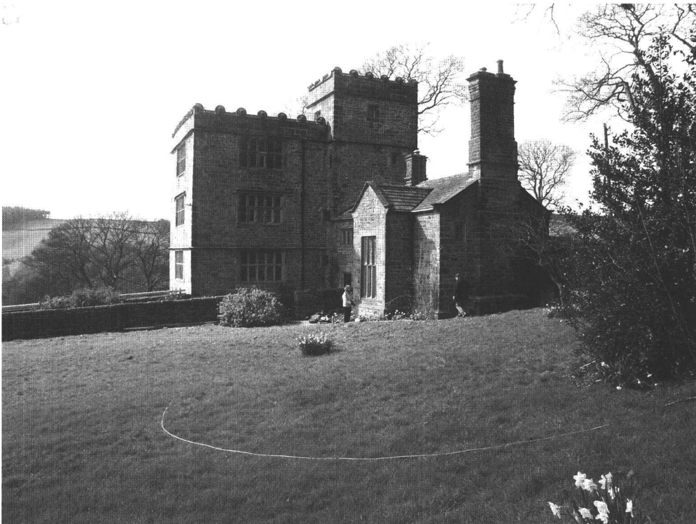
Plate 8: North Lees Hall: the 16th century hall, its later wing and, in the foreground, the grassed area where geophysical survey has revealed the outline of another structure.
