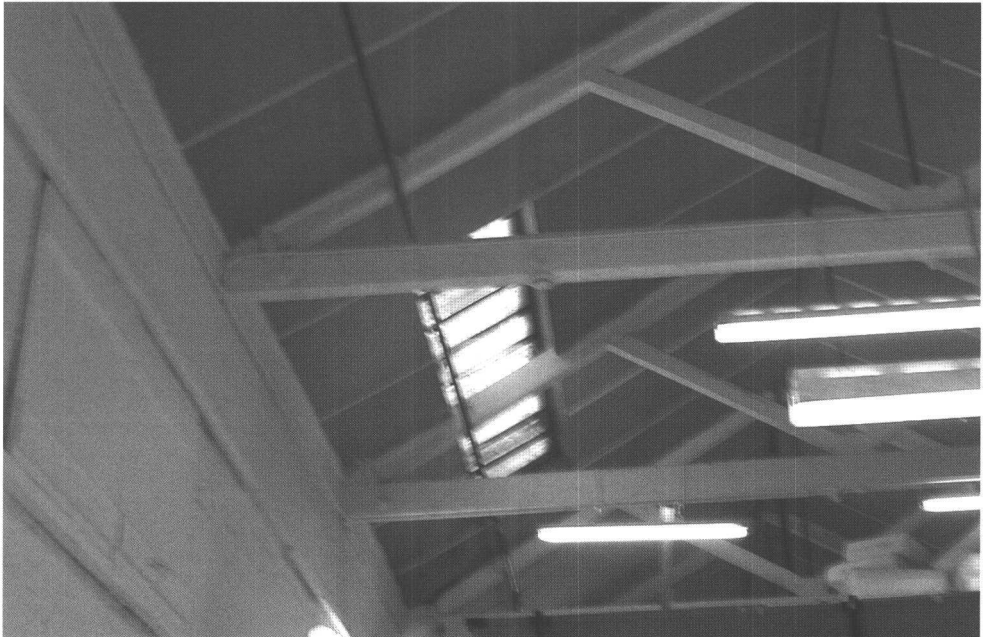
Plate 10: Coke Store — interior and roof structure.
