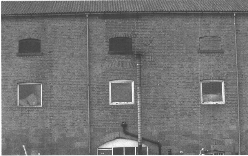
Plate 7: Coke Store north elevation — infilling in wall above arched entrance to canal.
