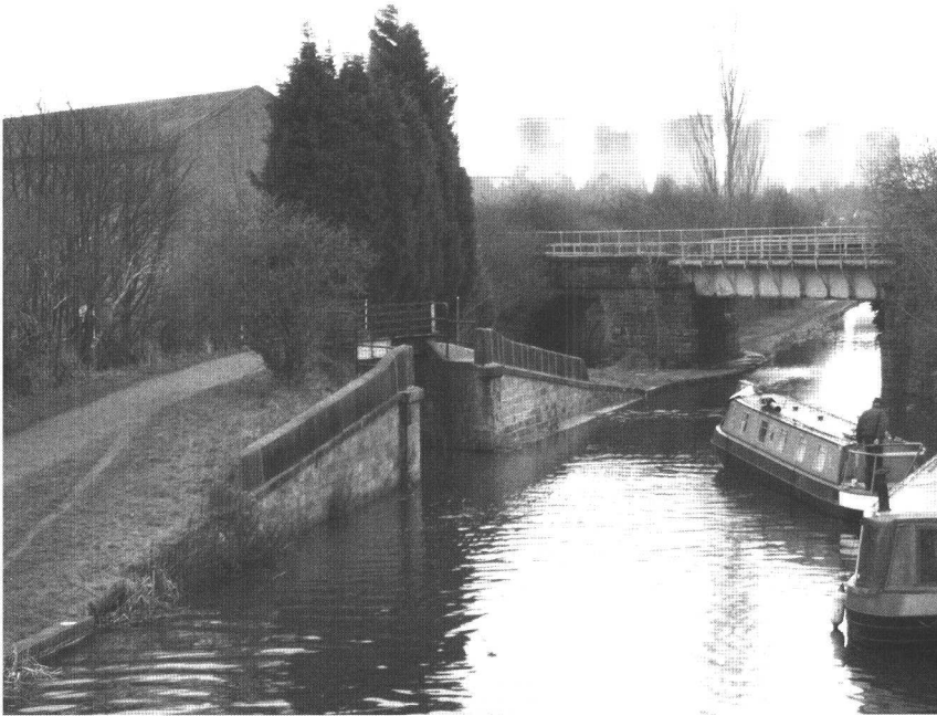
Plate 1: Entrance to basin from Erewash Canal.
