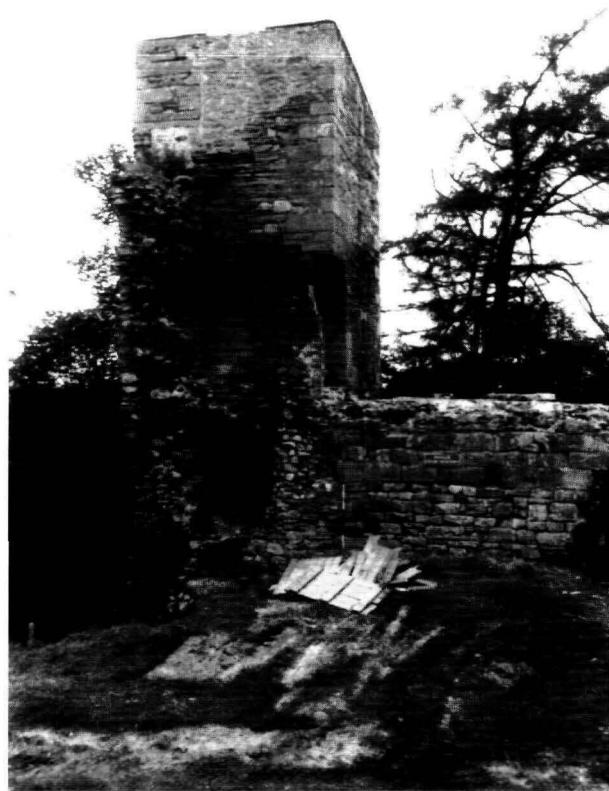
illus 33 The north-west tower, viewed from the south. Note the stump of the demolished west curtain wall projecting from its south face.
