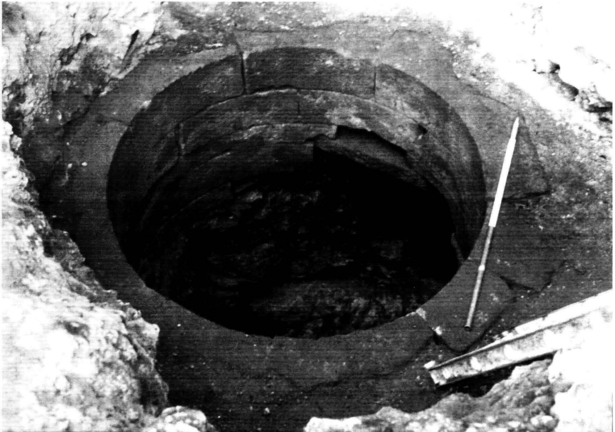
illus 59 View of the top of the well, showing the lintel supporting the well's ashlar lining, of which three to four courses remain. Below the lintel, the sides of the well comprise bedrock.
