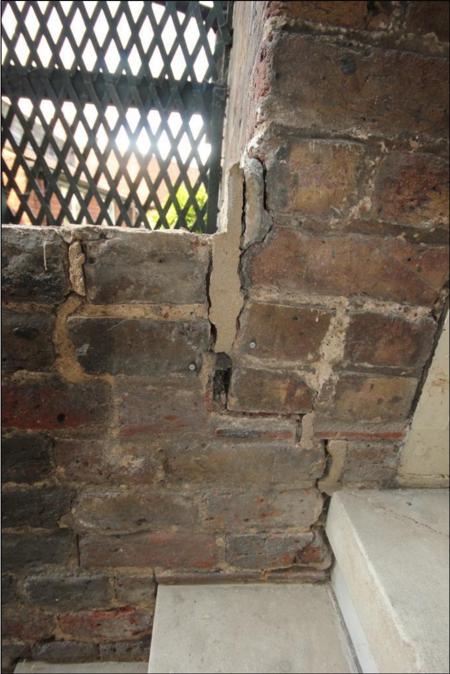
Figure 6: Crude mortar repairs where wall 1 meets the south face of the shed wall
