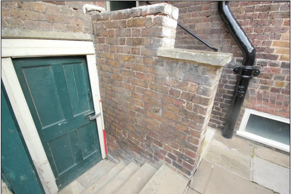
Figure 4: West-facing elevation of wall 1
