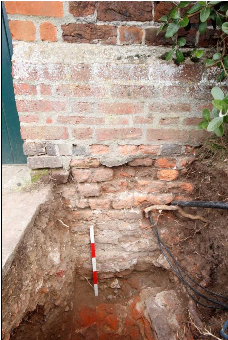
Figure 10: The boundary wall and its Tudor foundation, context 17
