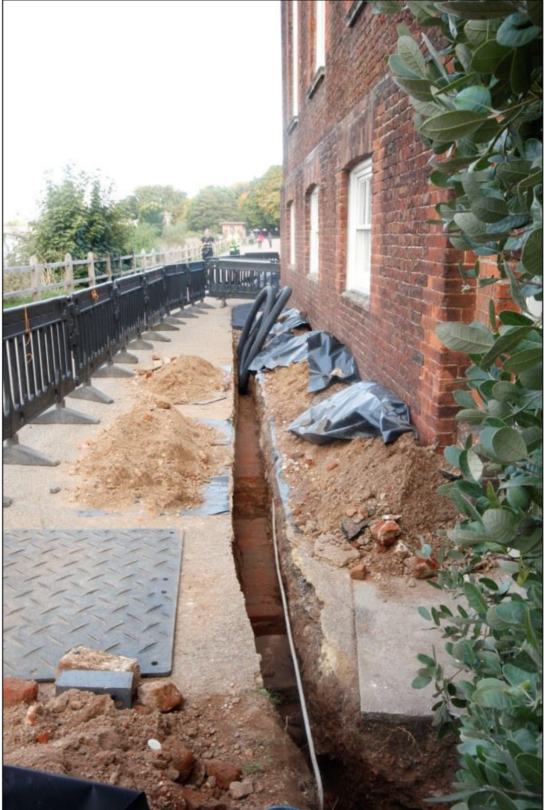
Figure 4: General view of the trench looking towards the west
