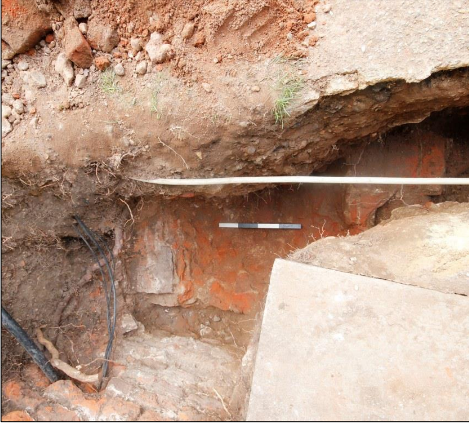
Figure 11: Tudor brick tubular drain seen from above truncated by context 17
