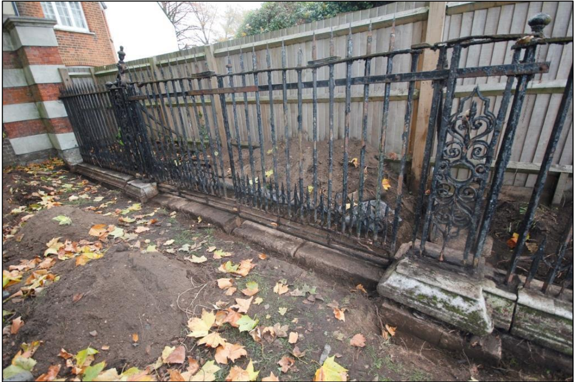
Figure 2: General view of Groom's House Gate after soil clearance viewed from the south-west
