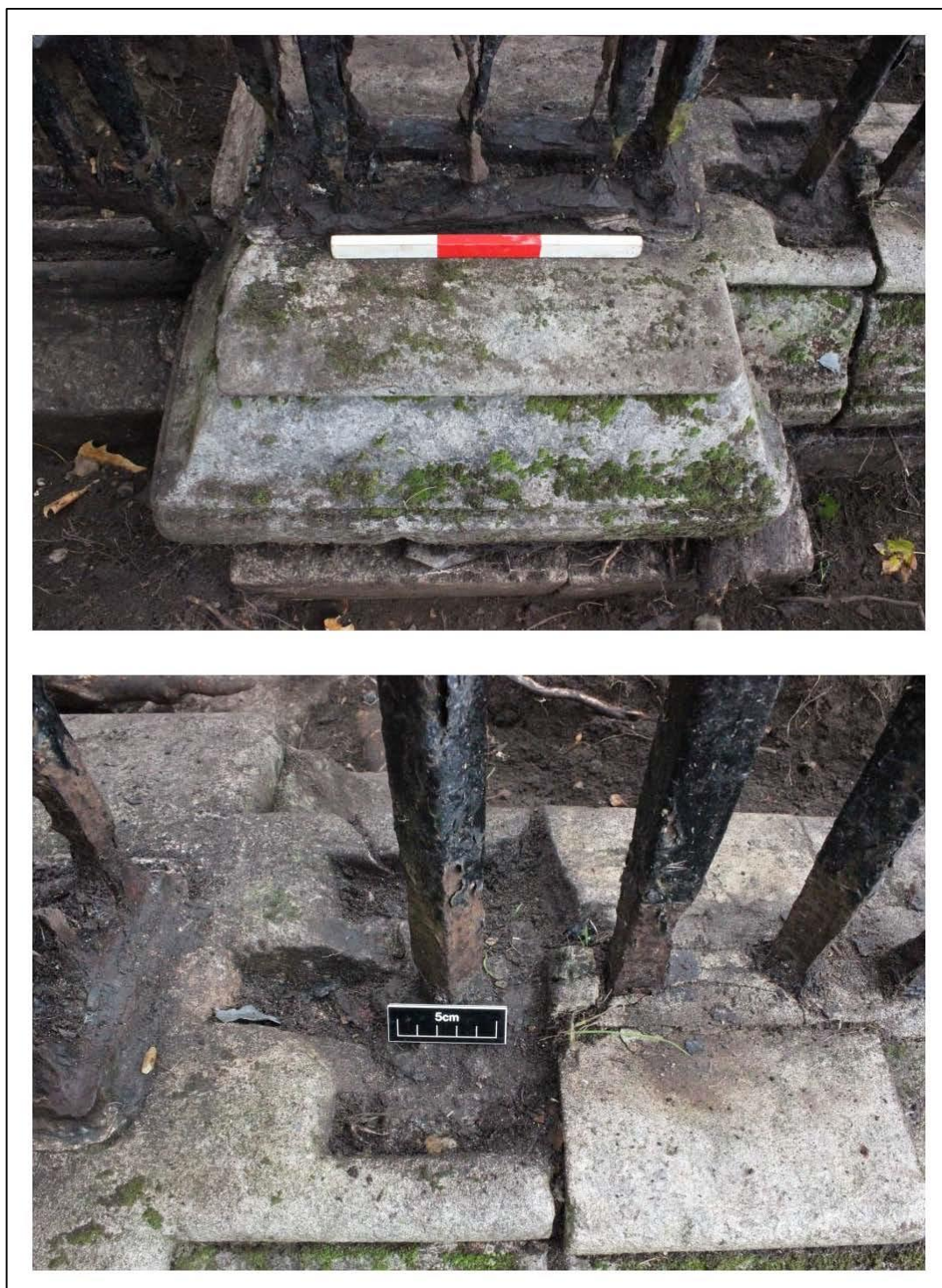
Figure 5: Top - Detail at the base of the southern box pier (1010). Bottom – recess cut into the southern plinth stone (1008)
