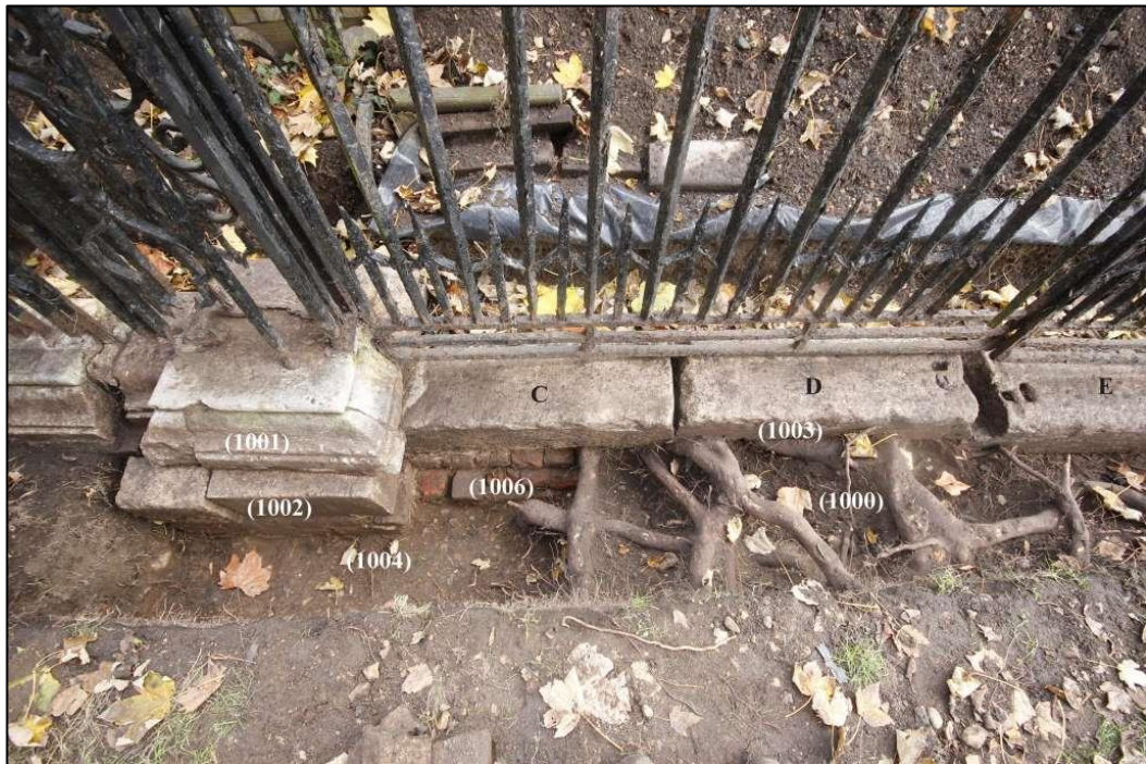
Figure 9: View of the damage caused to the threshold by the Plane Tree roots
