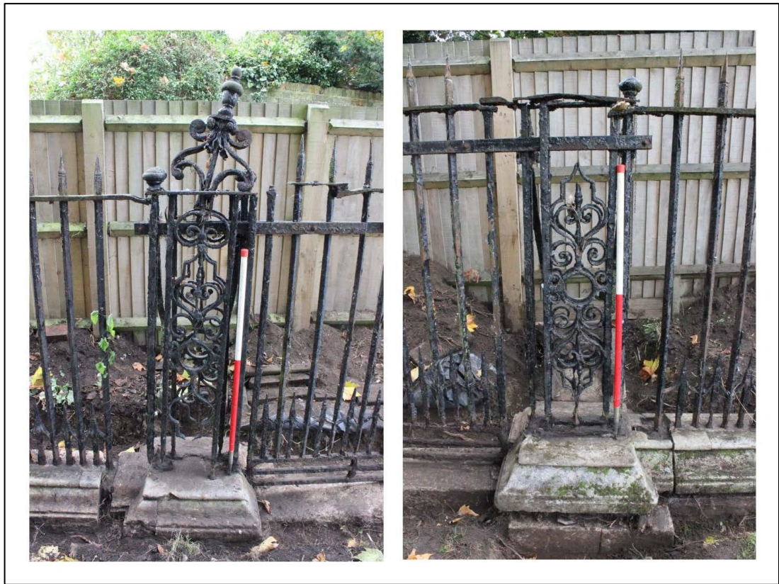
Figure 3: Groom's House Gate box-piers, (1009) and (1010)
