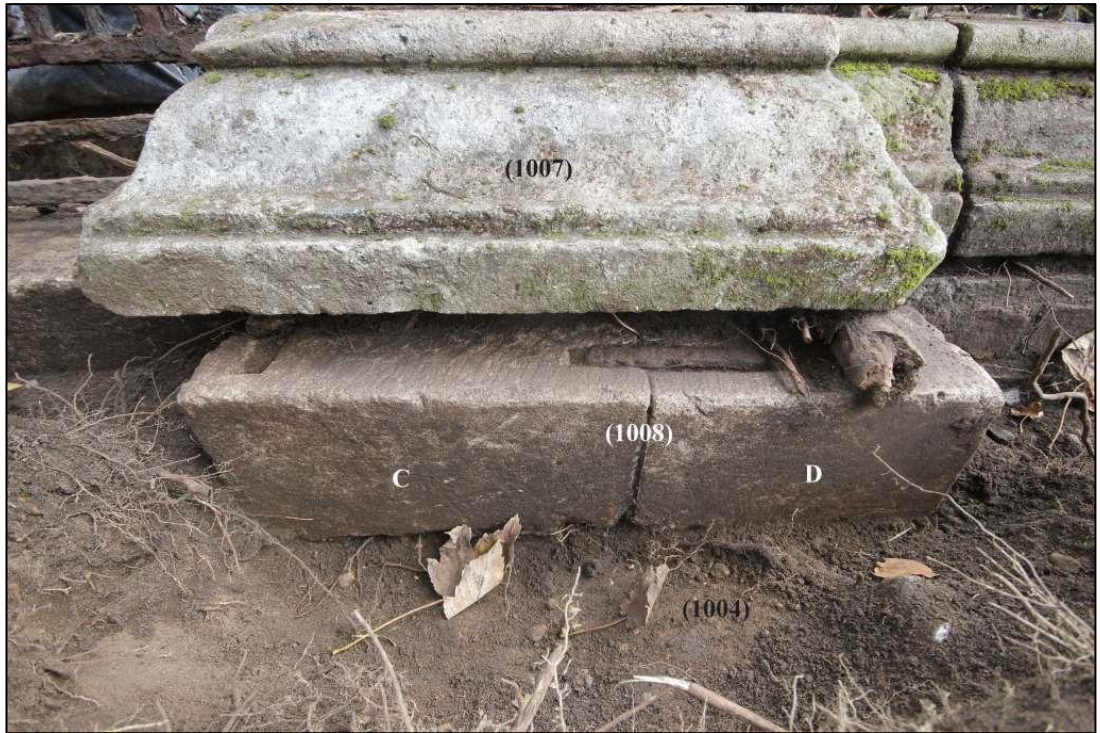
Figure 6: Northern plinth stone base and cap showing the recess and iron fixture in blocks C and D
