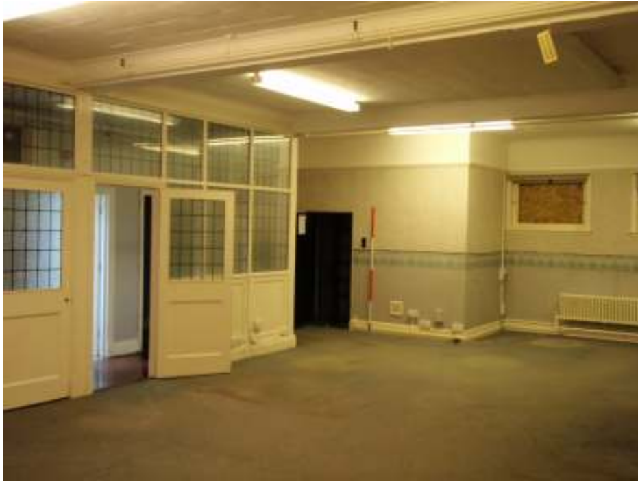
Plate 11: Ground floor room 2 looking south east, walk-in safe in corner, ceiling joists marking removed partitions visible
