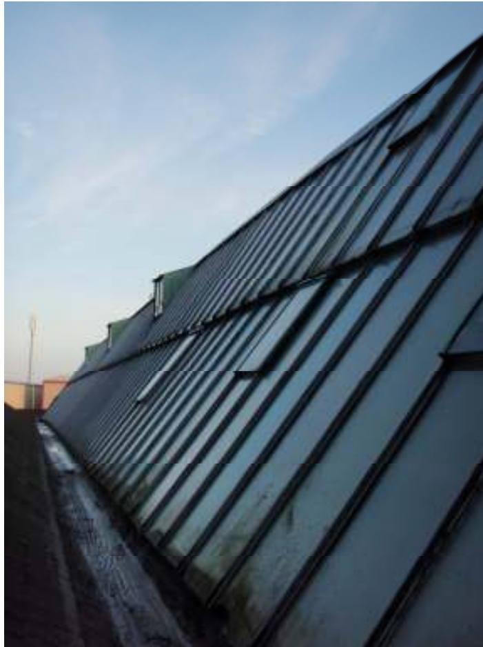
Plate 7: View of southern north light bay glazing from first floor rear window showing small ventilation dormers
