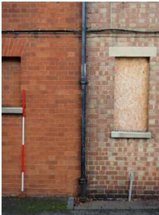
Plate 4: Detail of south elevation showing join between office and factory range
