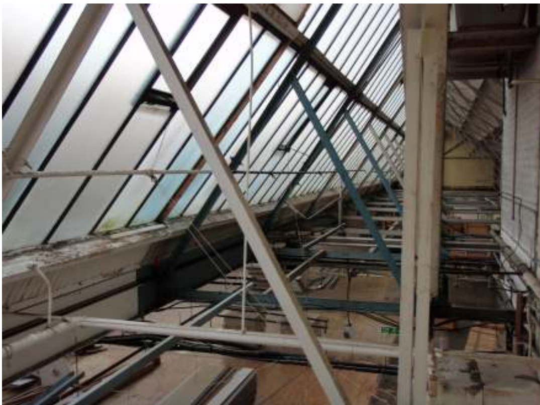
Plate 18: Factory range interior from first floor office range showing deep valley beam
