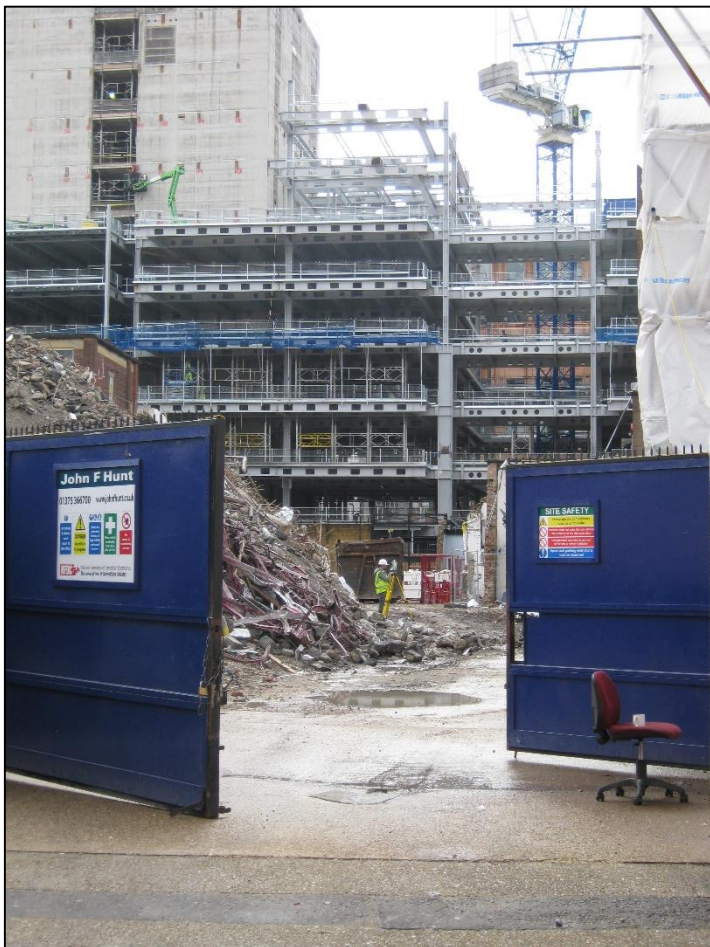
Looking south from Hewett Street into The Stage development site
