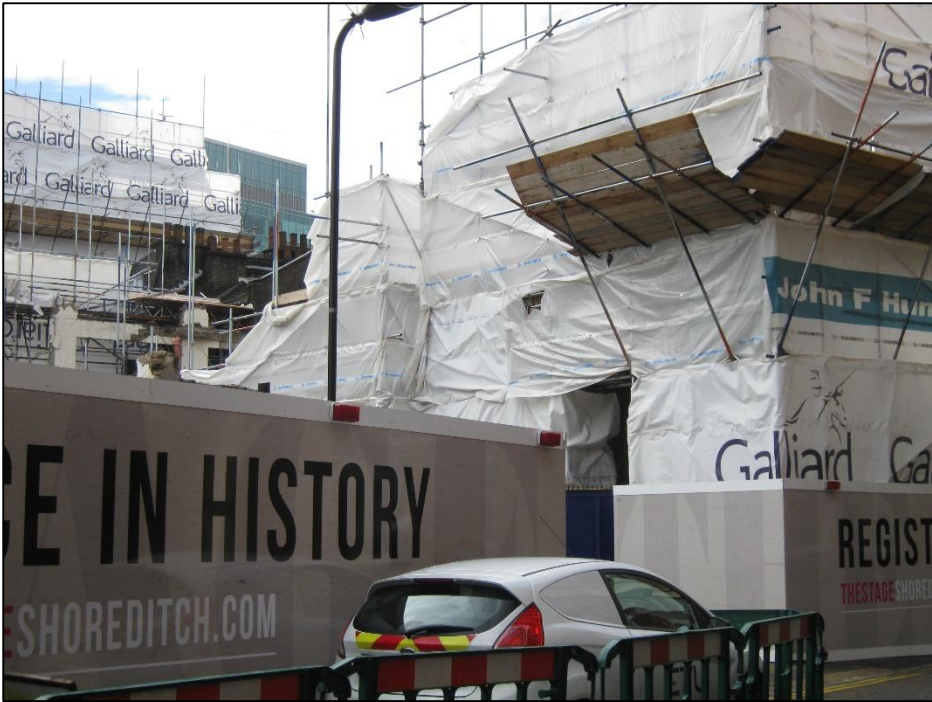
Looking south from Hewett Street towards the rear of 30 - 36 Curtain Road
