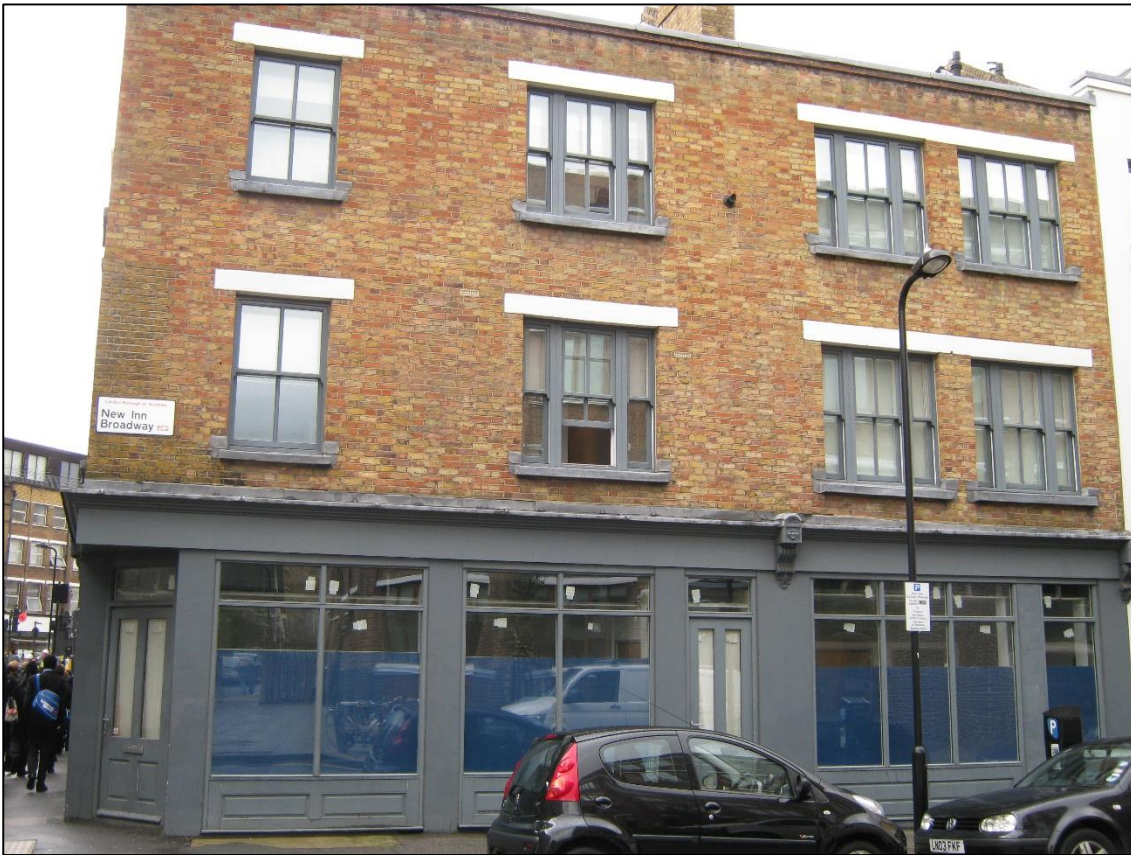
15 New Inn Yard and 3 New Inn Broadway, looking west
