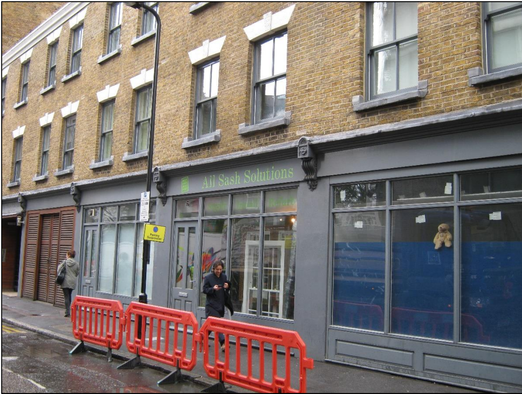
11 - 15 New Inn Yard, looking west
