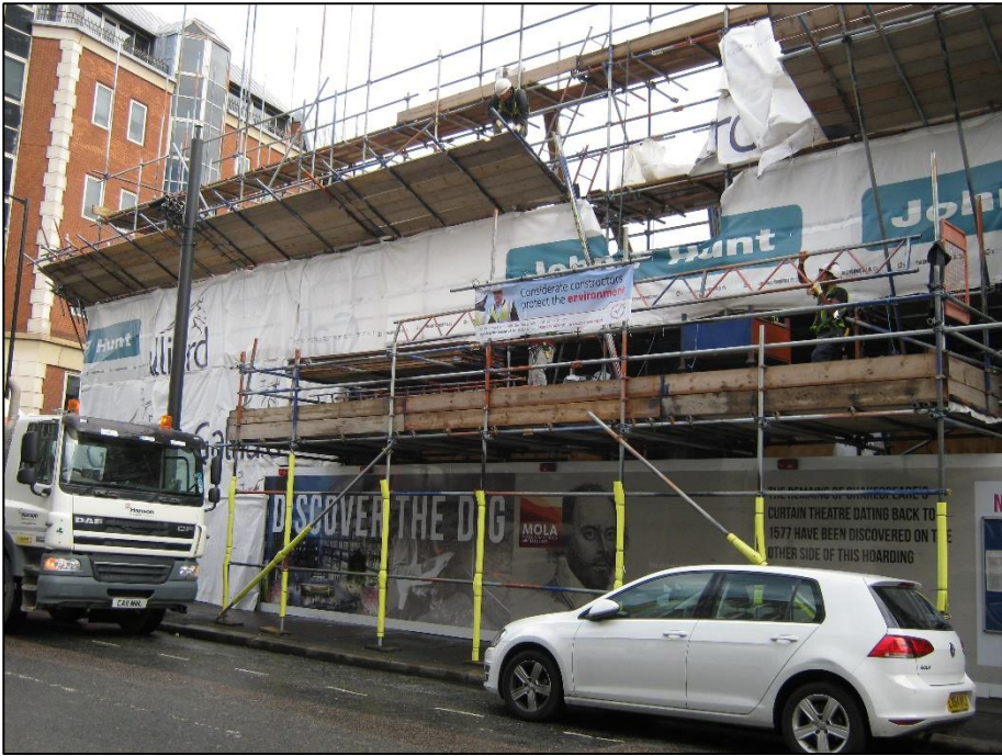
30 - 36 Curtain Road, looking east
