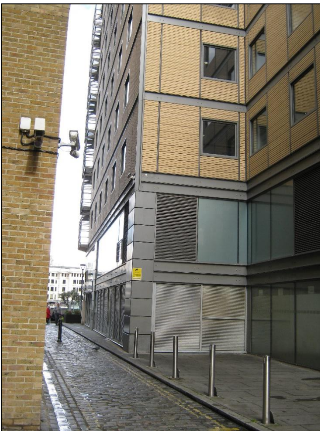
Rear of Riverside House, looking north on Bear Gardens
