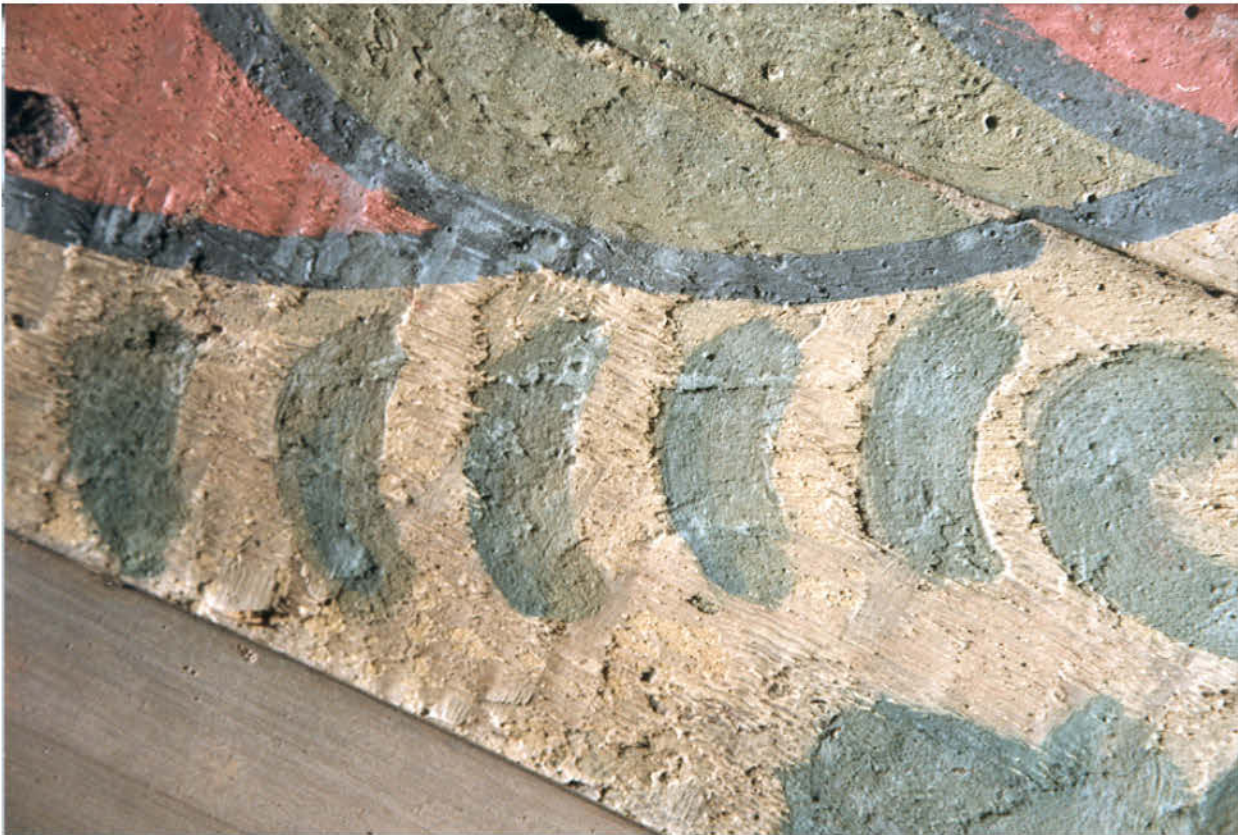
Figure 15. St Albans Cathedral, C15th Choir Ceiling: Detail showing the apparently receded wood surface where original background paint had been lost. The same phenomenon has occurred on the nave ceiling at Peterborough Cathedral.
