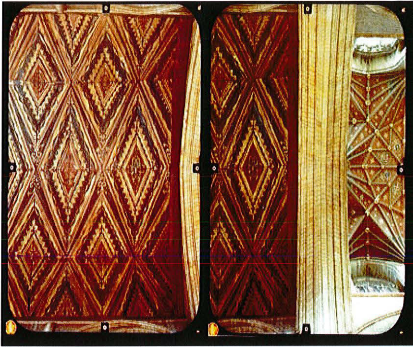
Figure 4. Stereo pair taken with Zeiss UMK 30/1318 metric camera of eastern most bay
