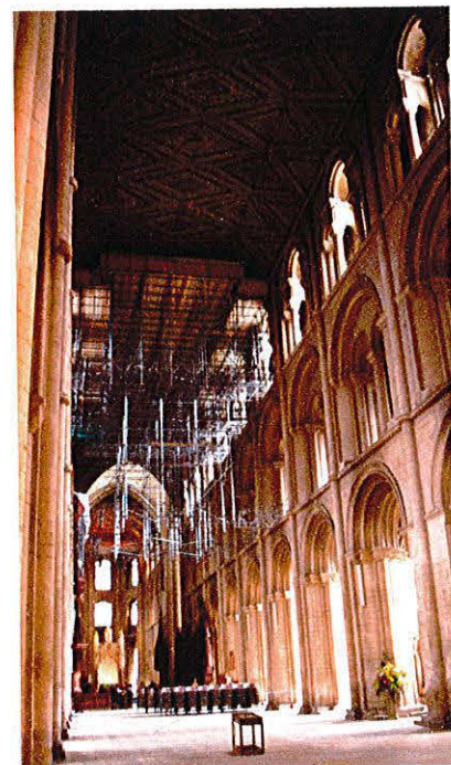
Figure 1. View of the nave, facing east. (Photo: TCA 2000)
