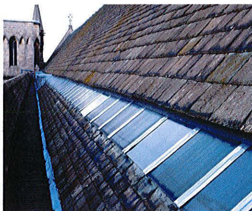
Figure 9. Windows on the south side of the nave roof. (Photo: TCA 2000)
