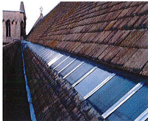
Figure 4. Windows on the south side of the nave roof. (Photo: TCA 2000)
