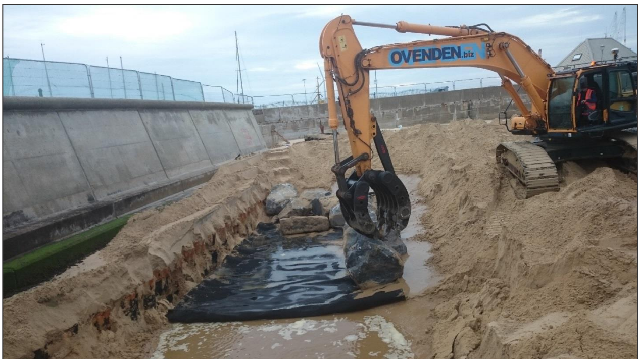
Plate 6: Shallow excavations in advance of Knuckle rock placement
