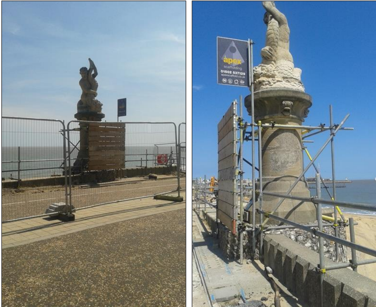
Plate 3: Protection installed around Grade II Listed Statue of Triton (3)
