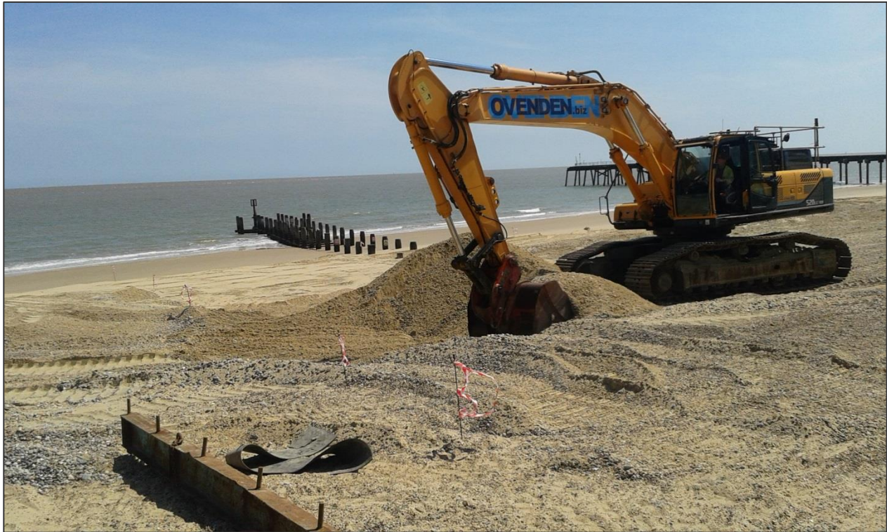
Plate 7: Borrowing of beach material from the causeway donor area, on the north side of Claremont Pier
