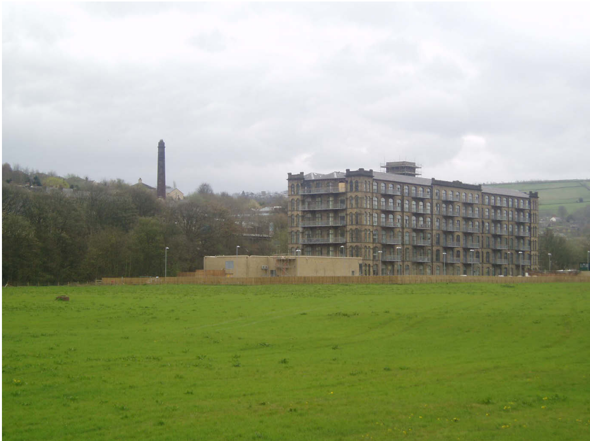
Figure 276. Titanic Mills. Linthwaite. 2002. Mill conversion to flats and a spa
