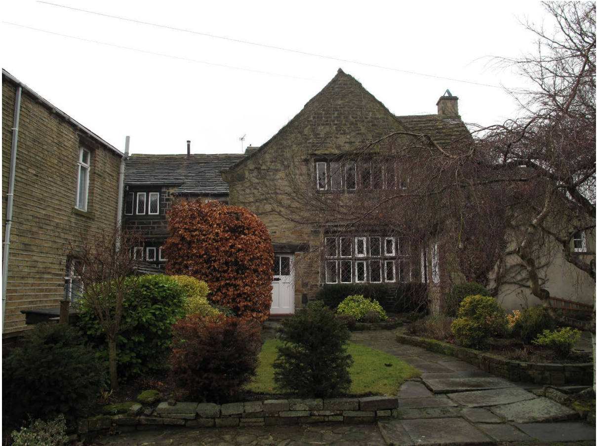
Figure 311. Quarmby Old Hall, Quarmby. 2010
