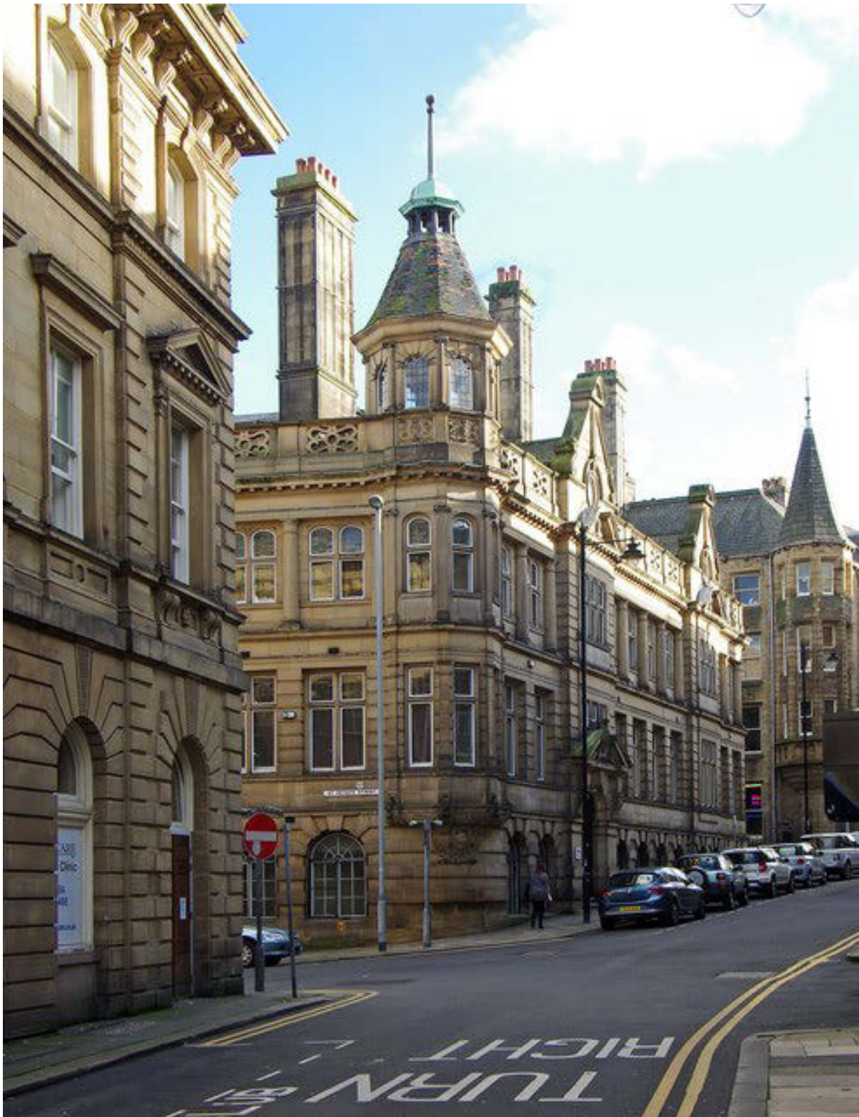
Figure 419. Station Street Buildings, Huddersfield © Copyright Julian Osley and licensed for reuse under this Creative Commons Licence. www.geograph.org.uk/photo/4209932
