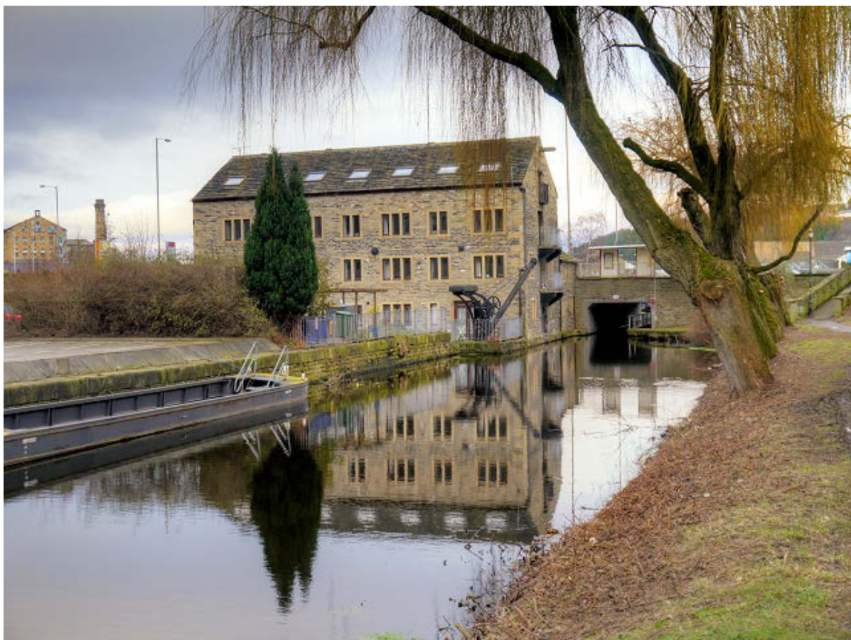
Figure 396. John Ramsden Court, Huddersfield Broad Canal. It was erected c.1776 by Sir John Ramsden for storing wool. There are taking-in doors on four levels and the remains of a winch system on the top floor. The right hand wing was added between 1780 and 1825; it was originally longer but was truncated when the Wakefield Road was widened in the 1960's. The warehouse is a Grade II* listed building. © Copyright David Dixon and licensed for reuse under this Creative Commons Licence. www.geograph.org.uk/photo/4304494
