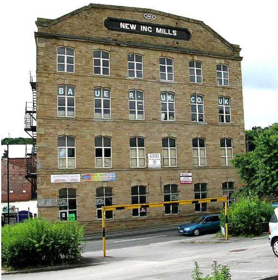
Figure 370. New Ings Mill. Four storey weaving shed dated to 1863. © Copyright Betty Longbottom and licensed for reuse under this Creative Commons Licence. www.geograph.org.uk/photo/487193
