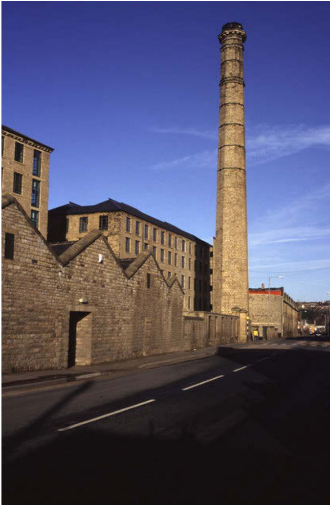
Figure 406. Firth Street Mills and Larchfield Mills, Huddersfield. To the left of the chimney is the 6 storey Firth Street Mills, originally built as a cotton mill but later used by Fred Lawton & Sons Ltd for carpet yarn spinning. To the right is the 5 storey Larchfield Mills, built as a woollen mill. Both mills are now part of Huddersfield University. There was a second square chimney alongside the octagonal stone one but this was dismantled piecemeal. Photograph taken in 1998 prior to conversion. © Copyright Chris Allen and licensed for reuse under this Creative Commons Licence.
