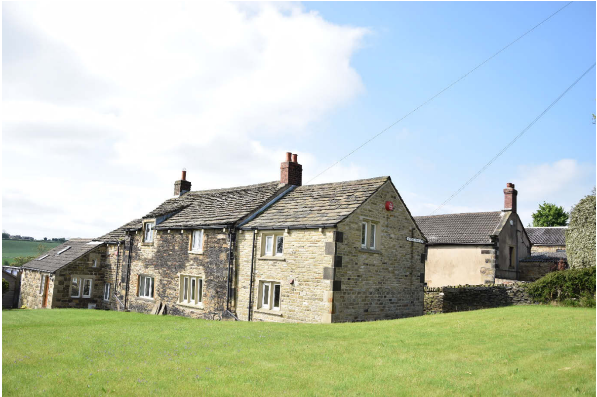
Figure 207. Westfield Cottage. Barnsley Road. Flockton. 2016
