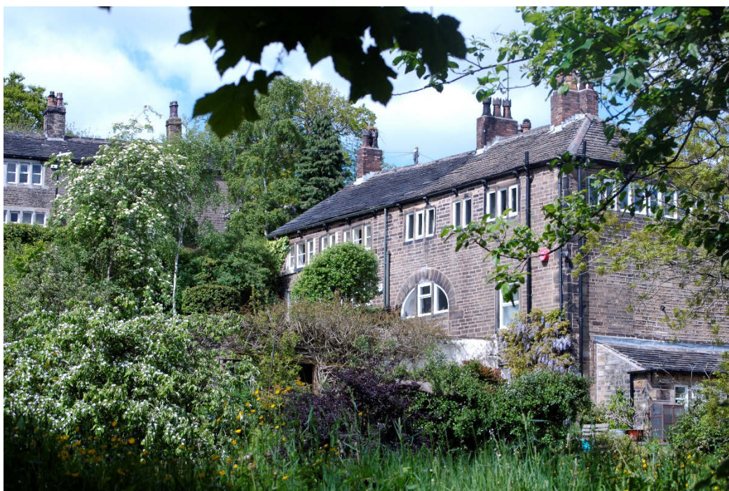
Figure 252. Upper Steps Mill. Steps. Meltham. 2013
