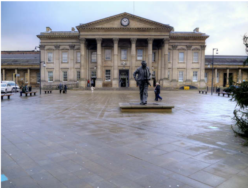
Figure 411. Huddersfield Railway Station ©
