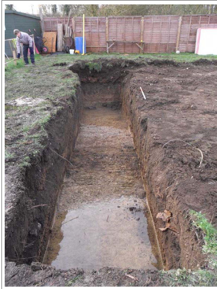
Plate 1: View along Trench 1, looking west Scale 1x1m
