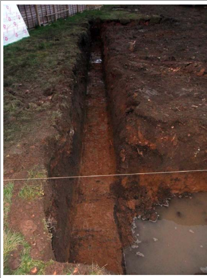
Plate 5: View along western foundation trench from end of trench 2
