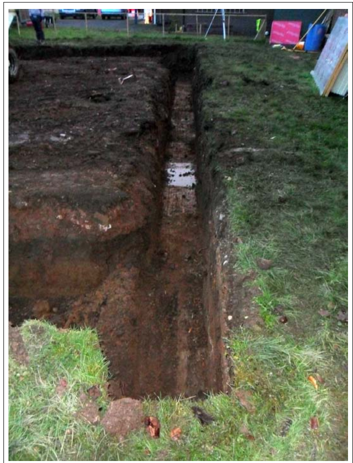
Plate 6: View along western foundation trench from end of trench 2
