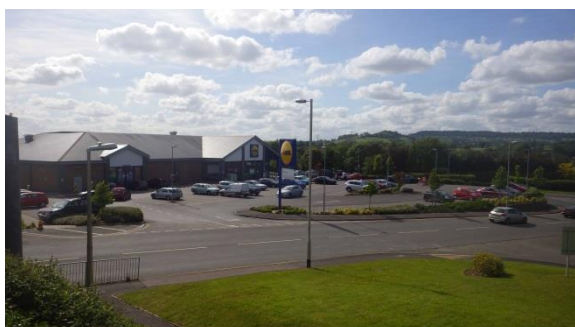
PL.155 Industrial estate. View to NW.
