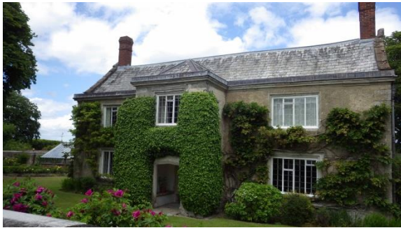
PL.118 Marwood House. View to NW.
