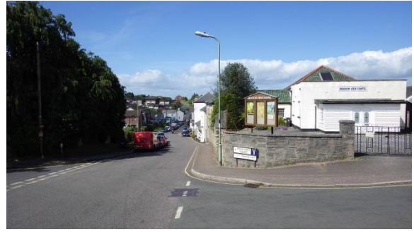
PL.45 HUCA 1 and HUCA 5. Along King Street back lane. View to WSW.
