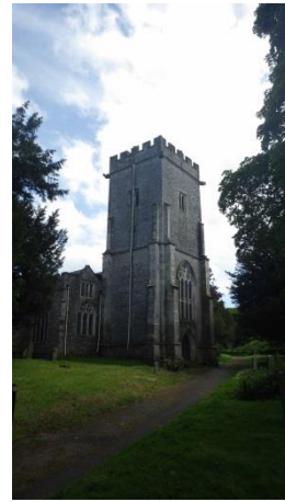
PL.146 Church of St Michael. View to SSW.
