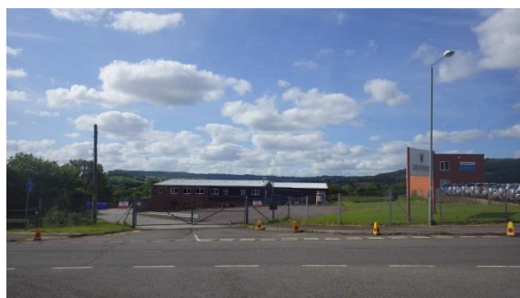
PL.158 Industrial estate. View to NNW.
