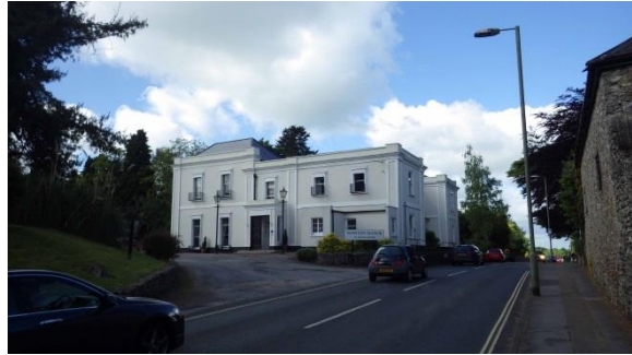
PL.29 Honiton Manor. View to SW.
