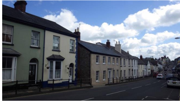
PL.22 Low houses and Shop units. View to NE.
