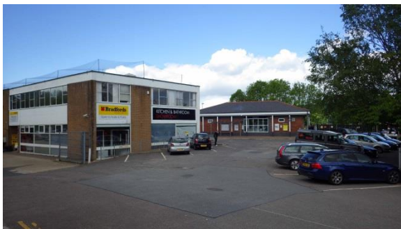
PL.72 Station and curtilage. View to NW.
