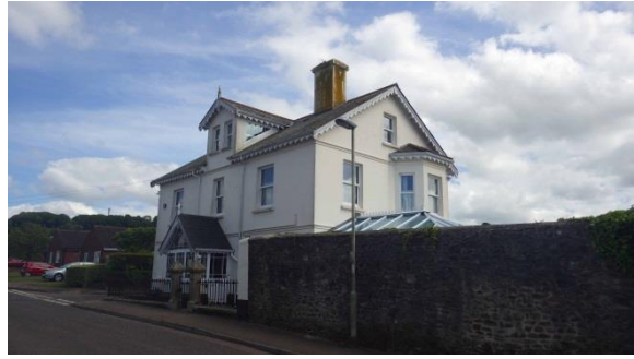
PL.104 Pine Park House. View to SE.
