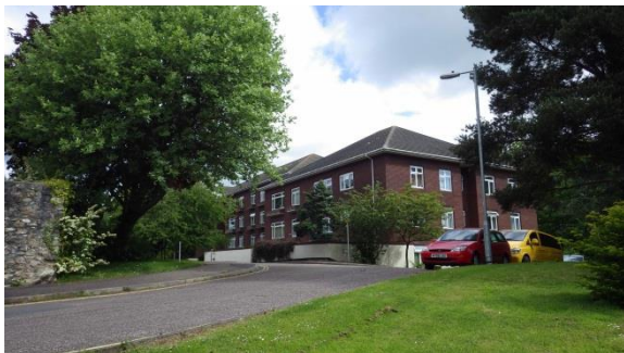
PL.37 20 th century mixed development on site of the former Rectory. View to NW.
