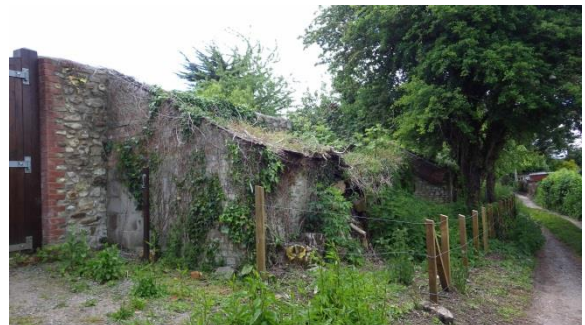
PL.87 Outbuildings to the rear of HUCA 10 on the back lane. View to WNW.
