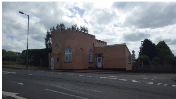
PL.101 Copper Castle Gate on Kings Road. View to SW.
