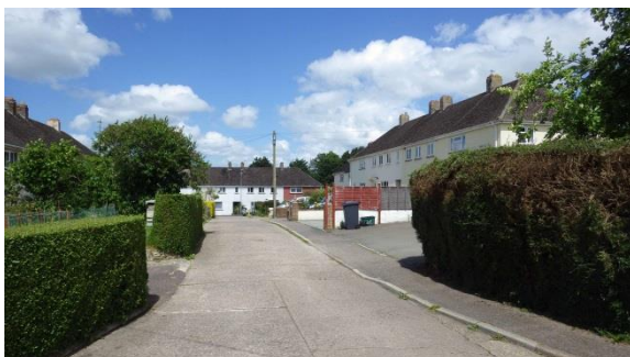
PL.131 Minifie Road. View to NE.
