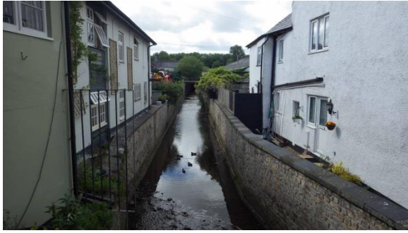
PL.21 Canalised River Gissage. View to SSW.
