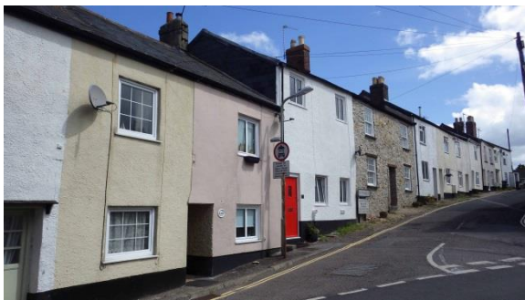
PL.68 View from Queen Street to Orchard Way. View to N.
