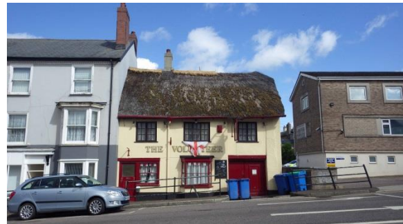
PL.18 The Volunteer Inn. Modern police station to the right. View to NNW.
