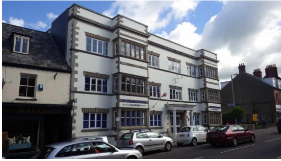
PL.7 Manor House. View to NNE.
