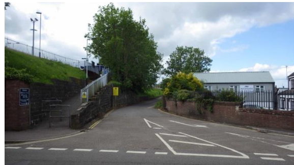
PL.71 Station and curtilage. View to SW.
