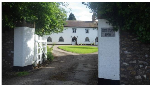
PL.56 Littletown House. View to SW.
