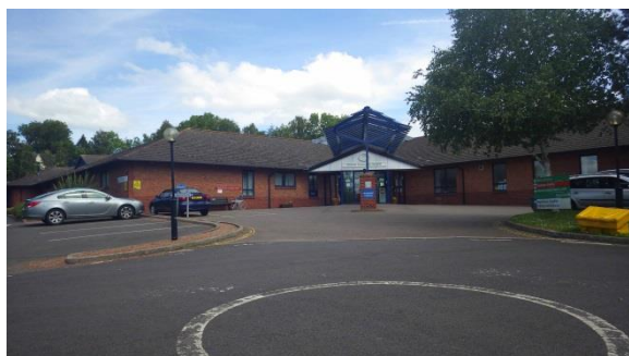
PL.77 Honiton Community Hospital. View to S.
