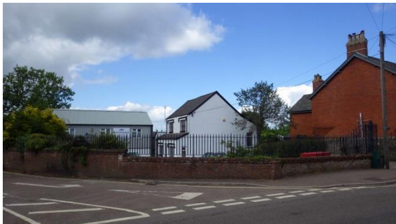
PL.70 Station and curtilage. View to W.
