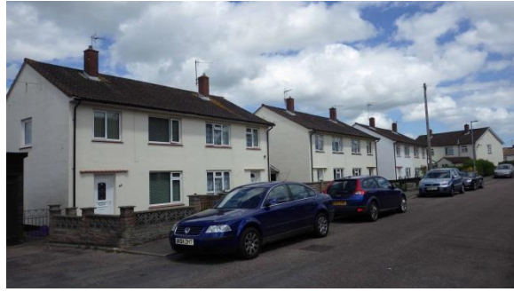
PL.111 Langford Avenue. Post-War residential buildings. View to NE.
