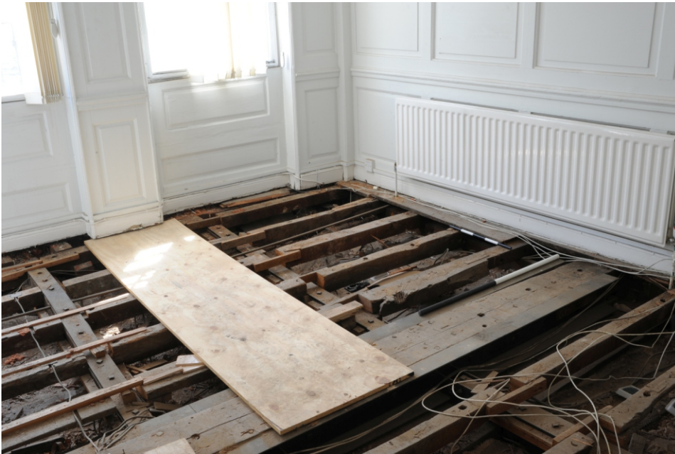
Appendix 3.24: Room F2 after removal of floor boards revealing primary floor beam with steel reinforcement, altered floor joists. SE
