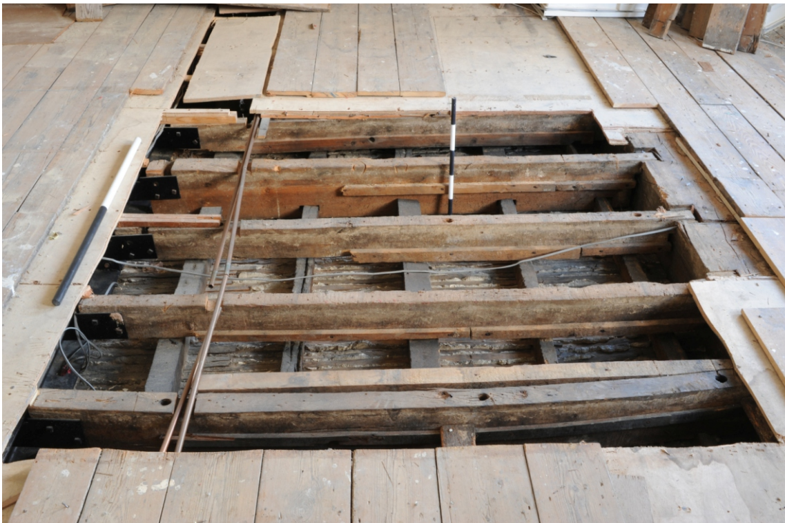
Appendix 3.23: Room S5, Area C. note perpendicular floor and ceiling joists, extant lath and plaster, steel cradles for floor joists on left hand side, surviving historic joints on right hand side into beam at the front of the rear bay. S
