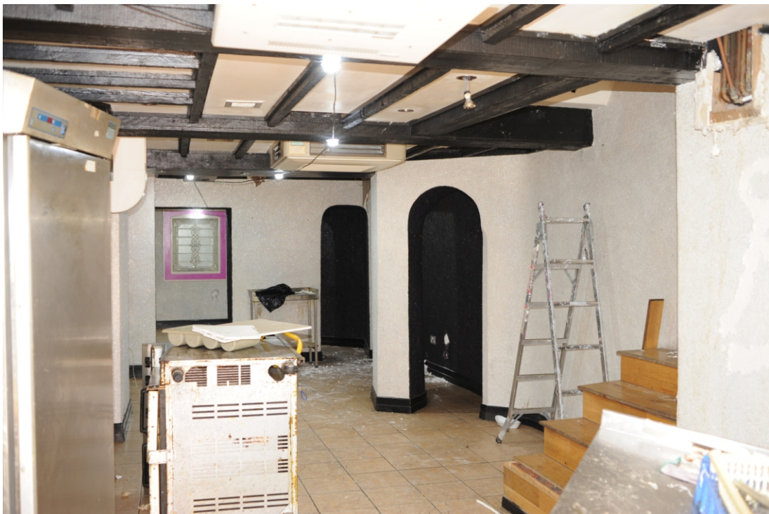
Appendix 3.3 (below): Basement/Lower ground room 1 looking towards the street, arched opening on right of image is in former angled stack and suggests a possible early partition. E
