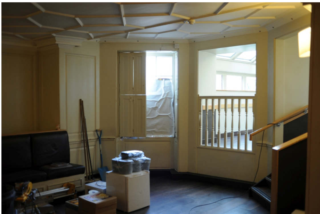
Appendix 3.8: Room G1 looking towards rear bay with extant shutters. SW
