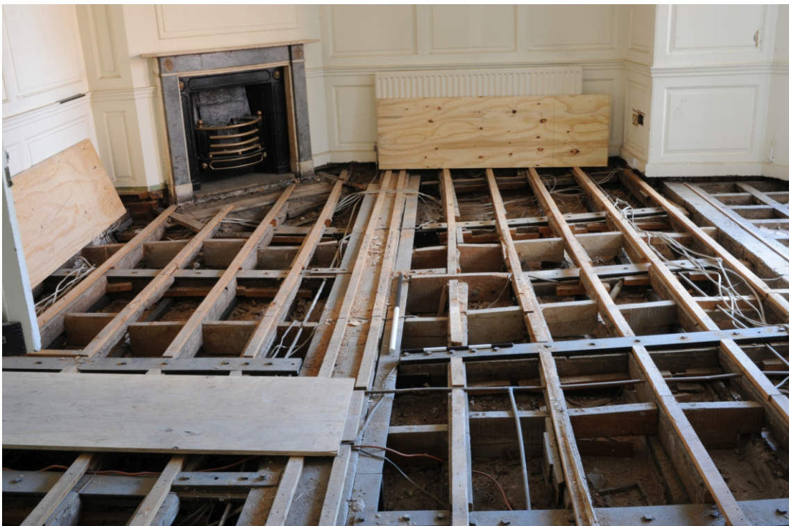
Appendix 3.28: Room F5 after removal of floor boards, looking towards the southern part of the room. S
