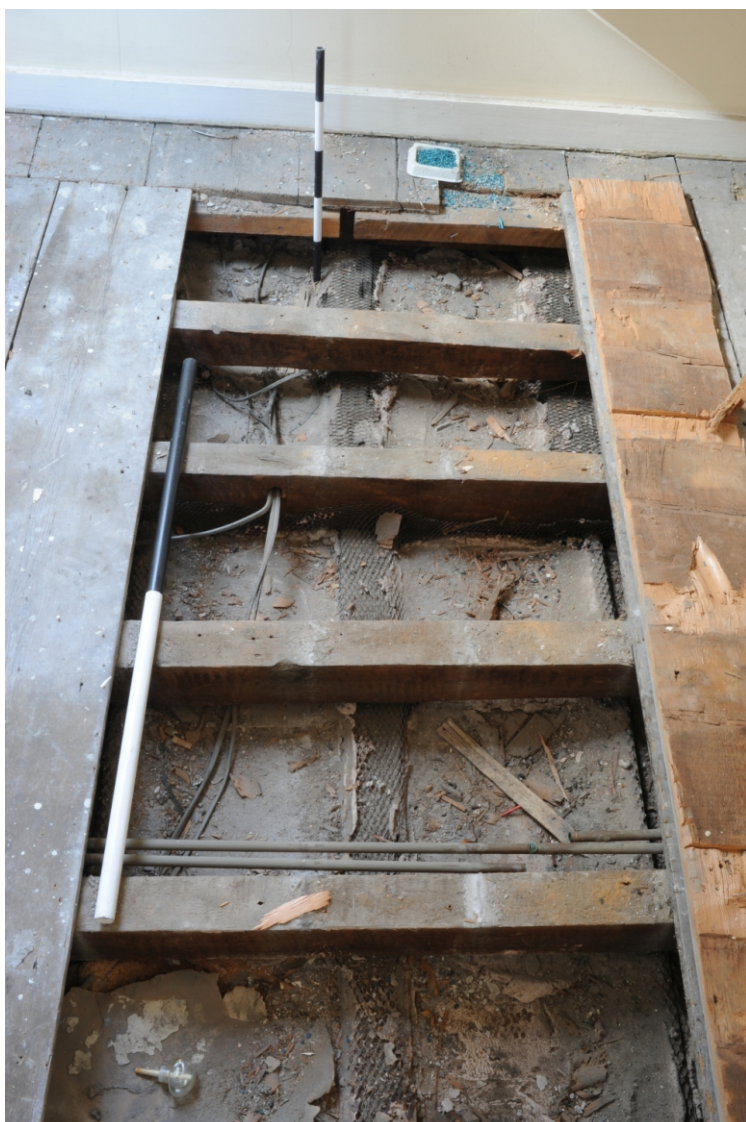
Appendix 3.19: Room Th4, Area A. Note perpendicular ceiling joists obscured by expanded steel mesh and ceiling plaster reinforcement. S
