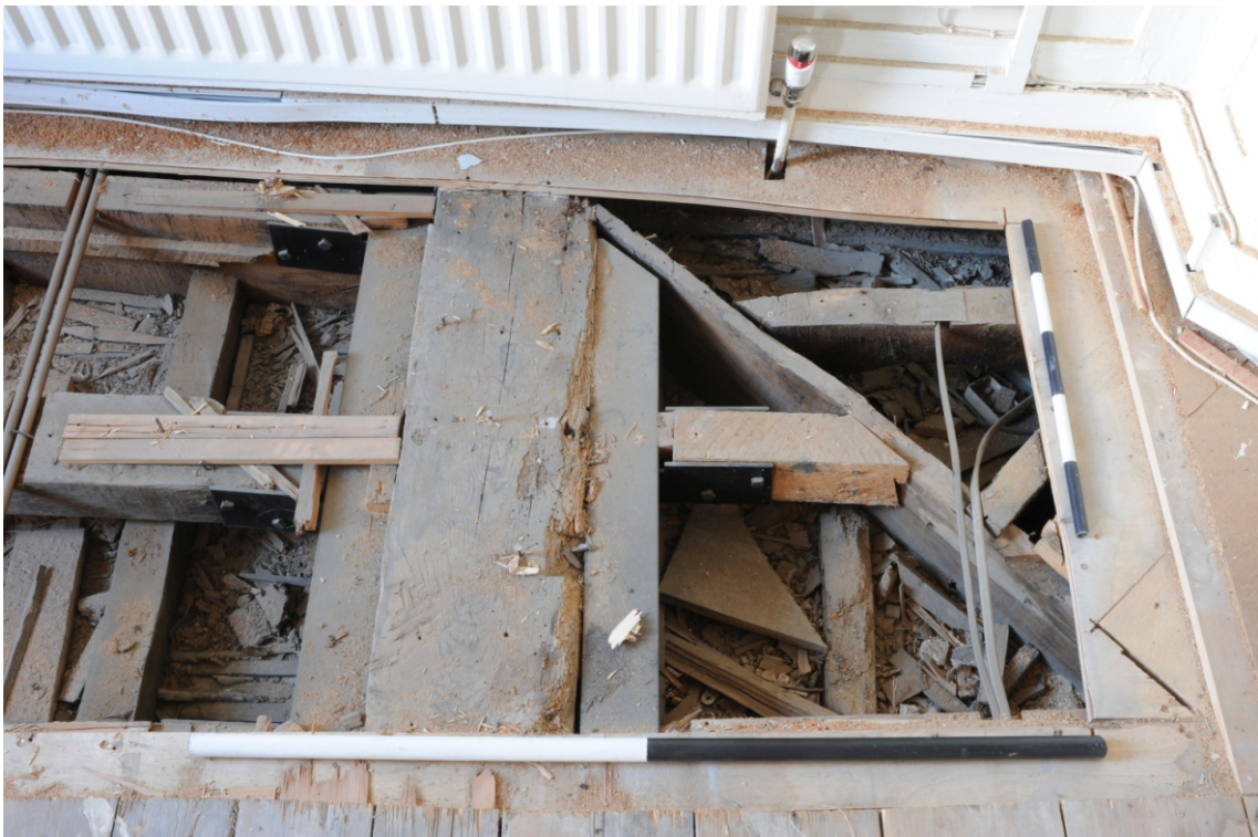
Appendix 3.21: Room S5, Area B, eastern end of open area showing principal floor beam, angled trimmer for the fireplace and steel reinforcements to main beam and joist on left hand side. N
