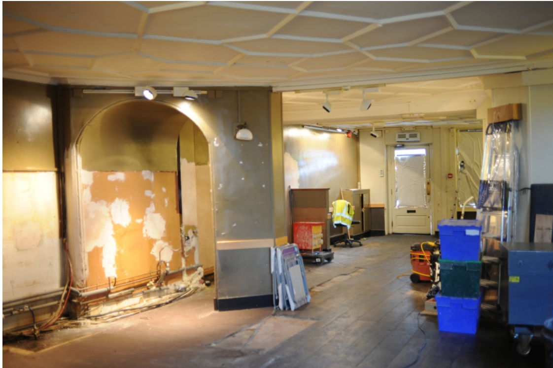
Appendix 3.7: Room G1 looking towards the front of the building. Arch on left in former angled stack, note decorated ceiling. E
