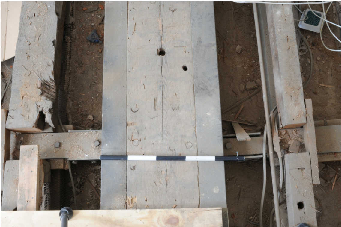
Appendix 3.30: Room F2 detail of main spine beam showing the steel cradles each side of the beam and smaller steels supporting floor joists, cut ends of secondary floor joists and peg holes within the main beam indicating original location of joists. S
