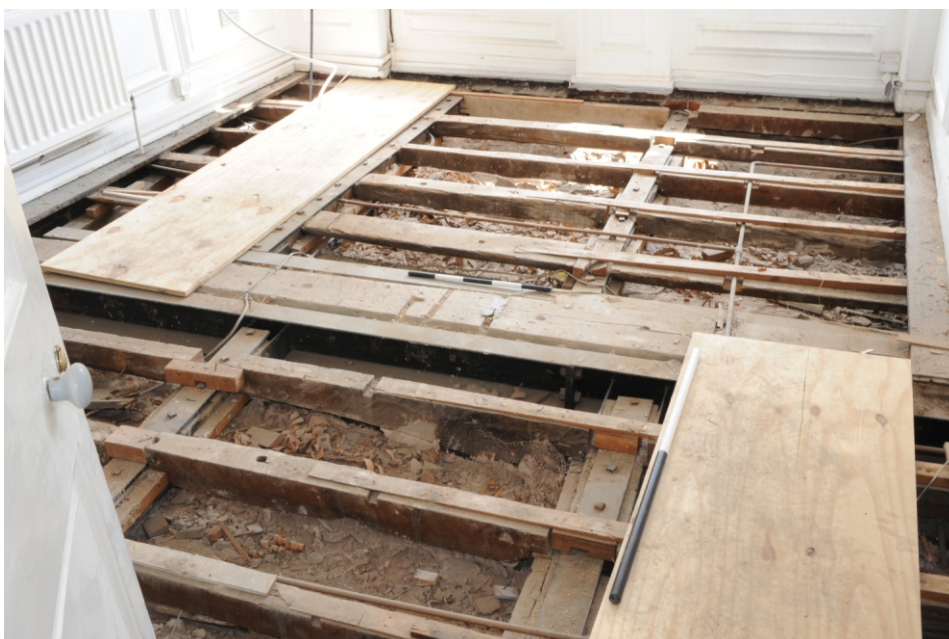
Appendix 3.26: Room F3 after removal of floor boards revealing floor structure, main floor beam continues from that in F2. E
