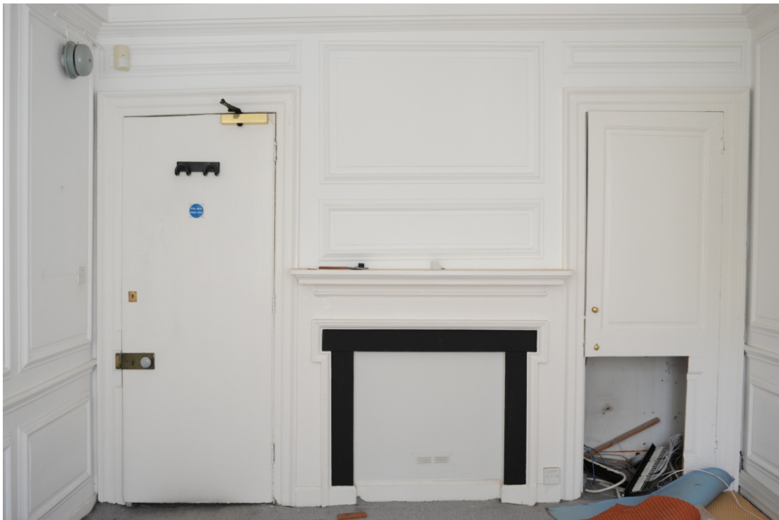
Appendix 3.10 (below): F3 blocked fireplace, door to right into cupboard. W
