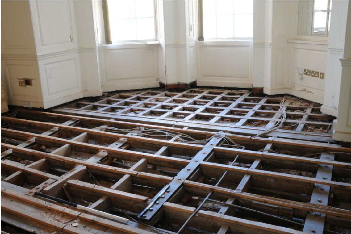
Appendix 3.27: Room F5, looking towards rear canted bay after removal of floor boards. SW
