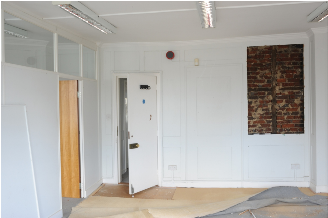
Appendix 3.15: Room S5, wall with exposed fabric, blocked doorway embedded within the panelling left of the opening. E
