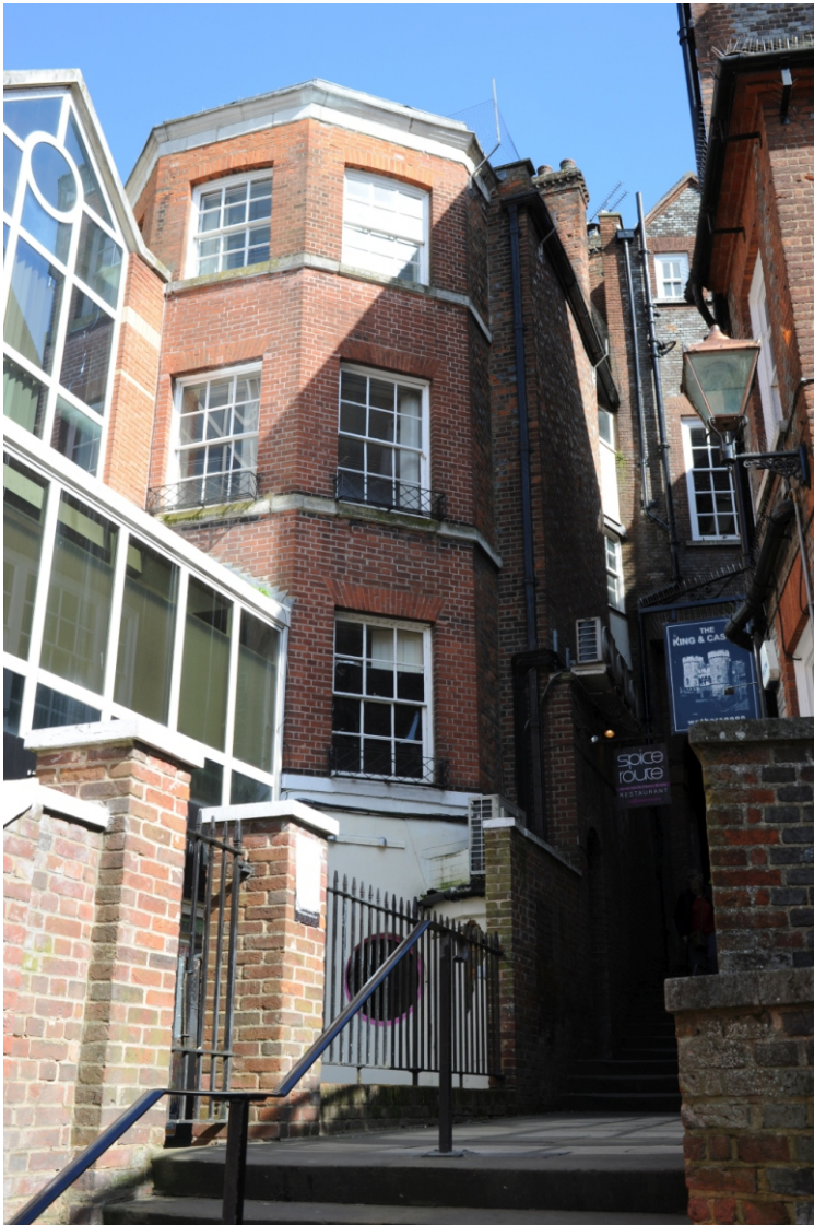
Appendix 3.2 (left): Rear elevation with canted bay representing the primary historic fabric. The late 20th century Cavendish House with glazed link is visible abutting the historic structure on the left of the picture. E
