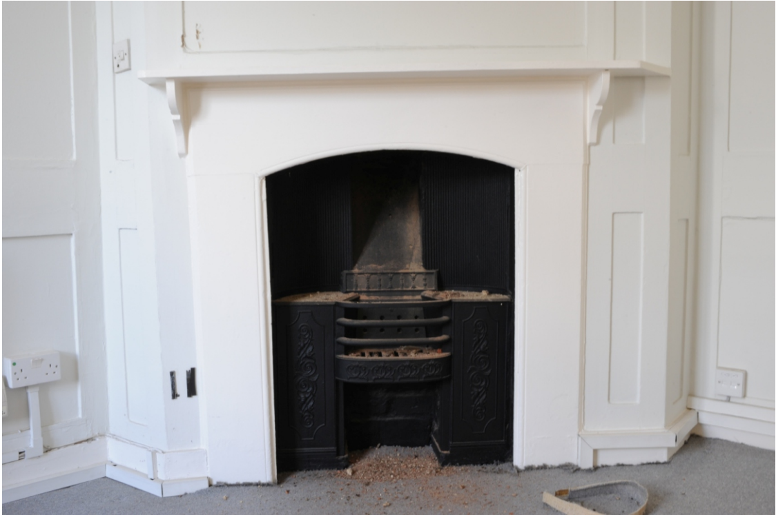
Appendix 3.14: Room S5, angled stack with grate. SE
