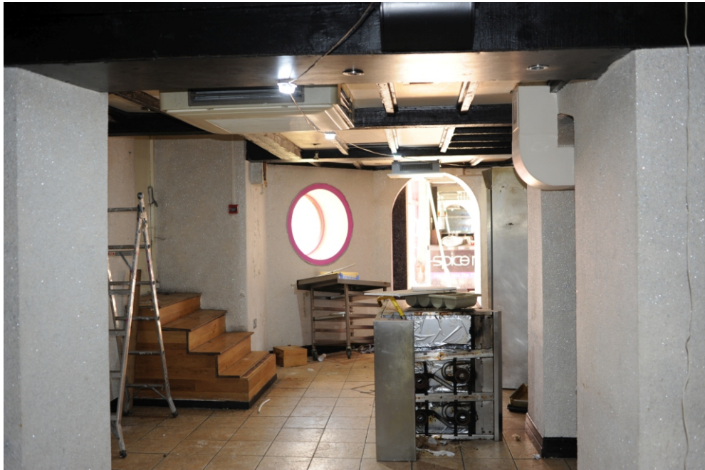
Appendix 3.4: Basement/Lower ground floor room1 looking towards the rear of the property. Steps on left lead to the alley S of the building. W
