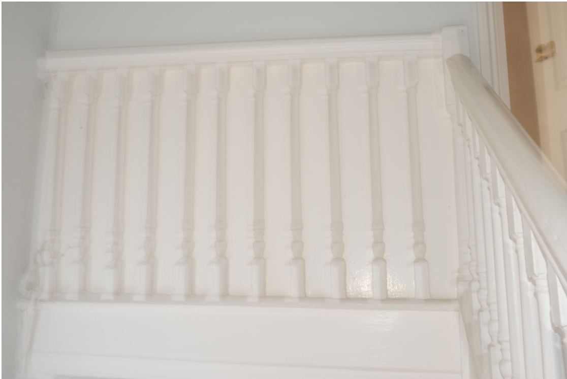
Appendix 3.16: Stair balustrade embedded within later fire partition. Th1. N
