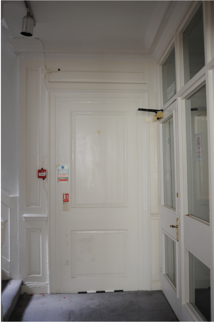
Appendix 3.9 (left): F1, blocked doorway formerly from stair into F5. Within F5 this doorway is panelled over. W
