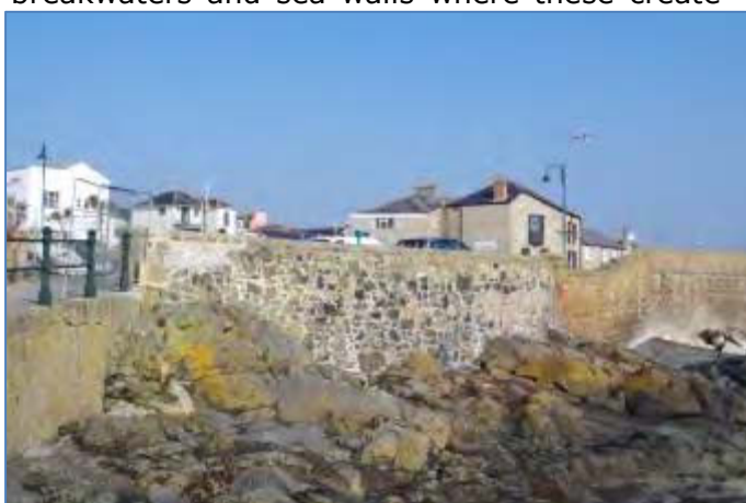
Fig 14 Historic phases of sea wall construction adjoining the South Pier, Penzance Harbour.
