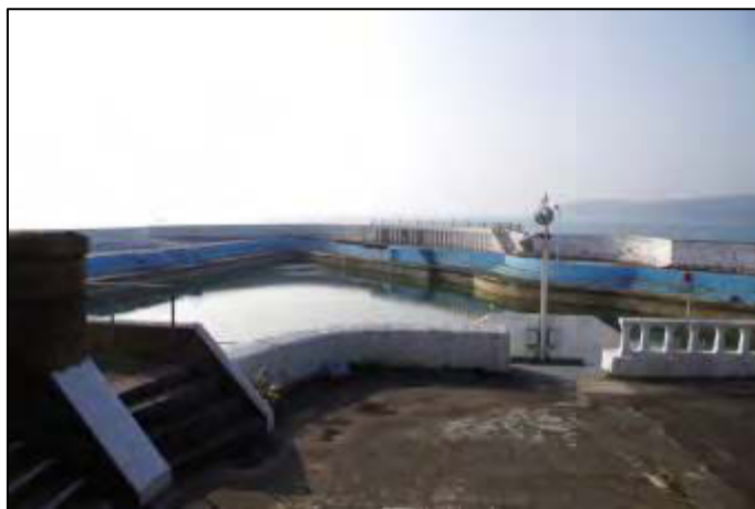
Fig 12 The Jubilee Pool lido, Penzance, built in 1935 on the foreshore of a small cove to the west of the main harbour. The lido incorporates the early 19 th century Battens Wharf.
