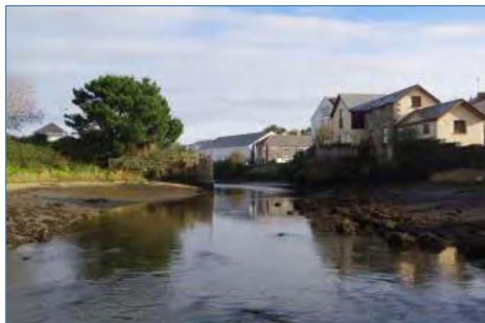
Fig 8 Copperhouse Dock, Hayle has been substantially encroached upon by modern redevelopment, resulting in substantial loss of historic setting.
