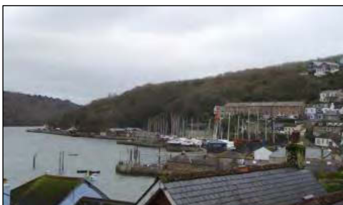
Fig 11 Late 19 th and early 20 th century shipyards extend along the shoreline to the north of Polruan, infilling between earlier quays and fish cellars.
