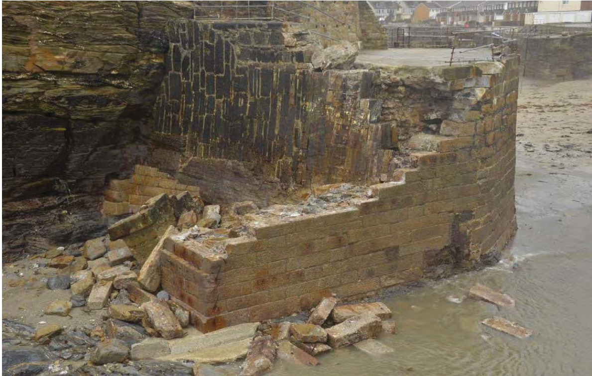
Fig 24 Storm damage to the eastern breakwater in February 2014 (photo: Ainsley Cocks).
