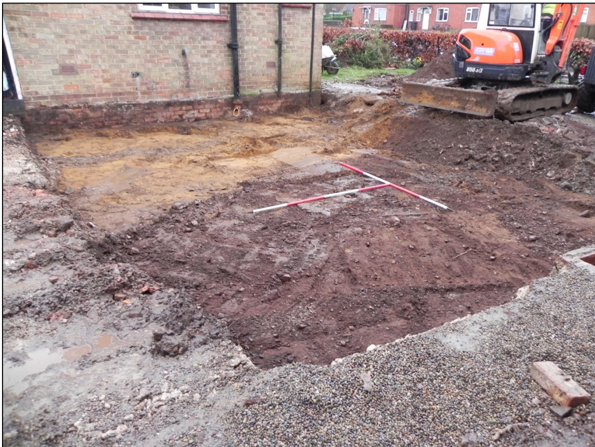
Figure 5: the site after the initial strip down to foundation level
