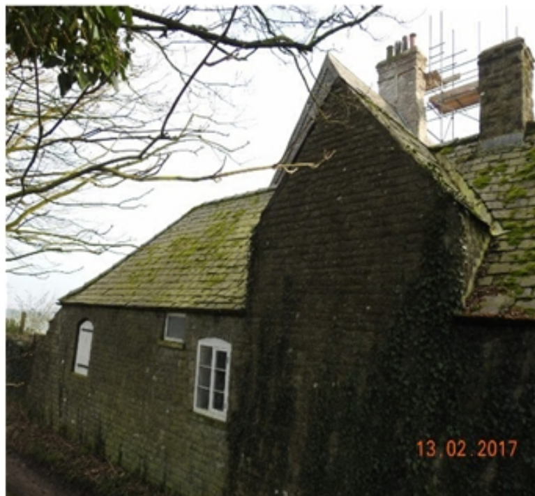
Plate 58 : Stables north facing roof from Carr Lane....13.02.17.
