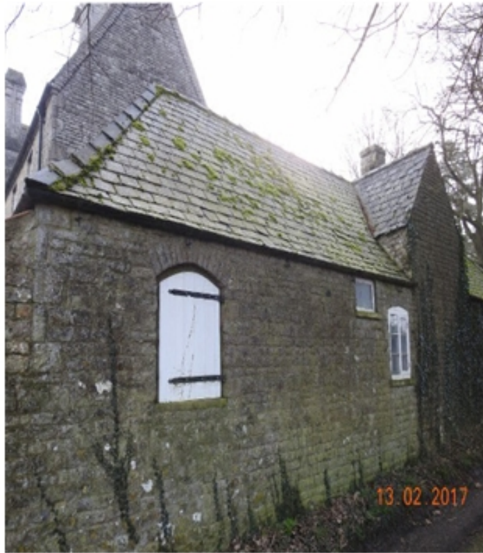
Plate 74 showing the north side adjacent to Carr lane loading flap door... 13.02.17.
