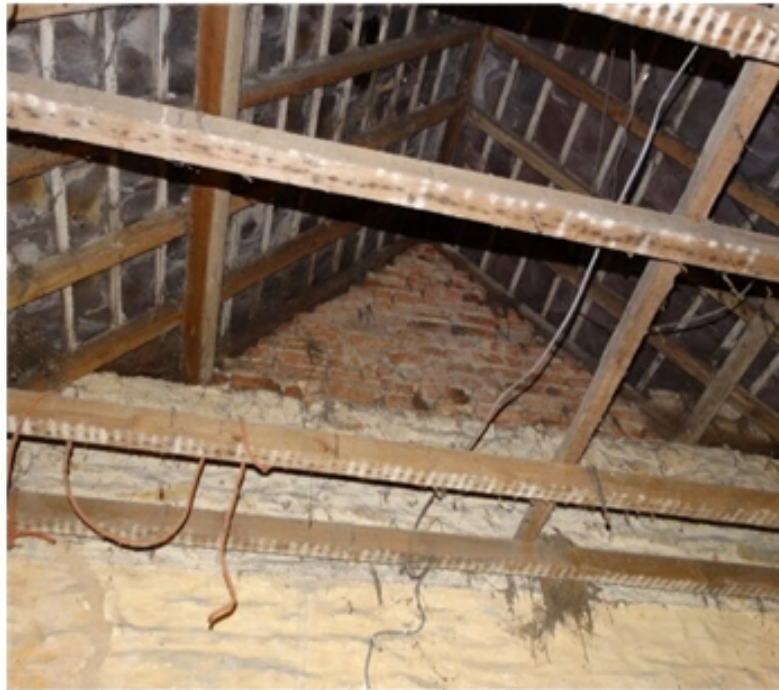
Plate 48 inside the Stables showing the east internal dividing wall and roof timbers looking towards the hayloft
