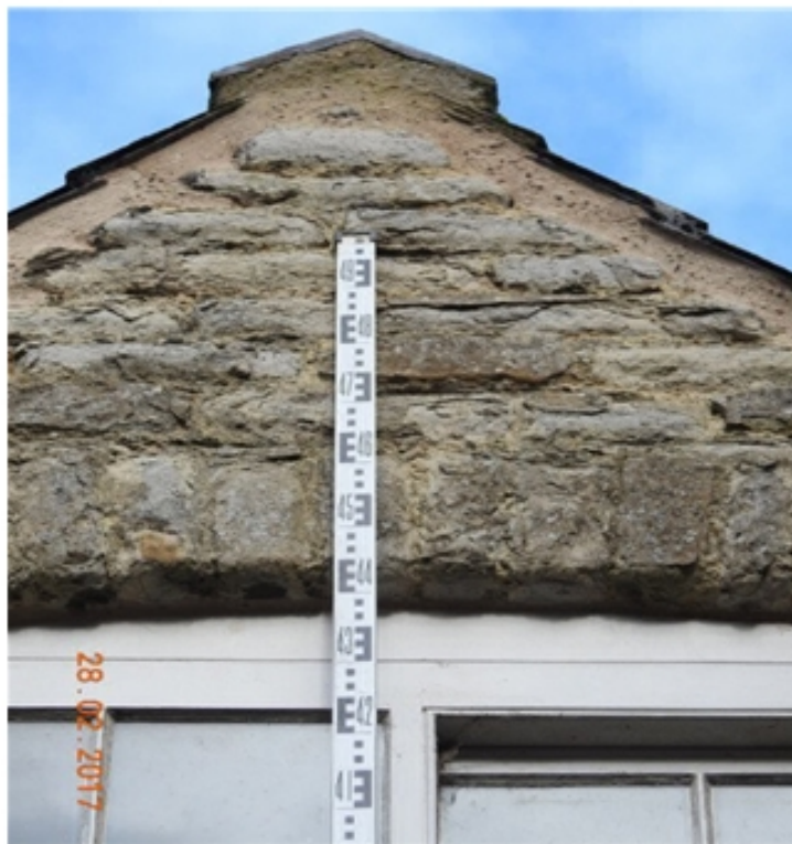
Plate 39 :Height of Hayloft south - facing window above ground level = 4.45 metres : 28.02.17
