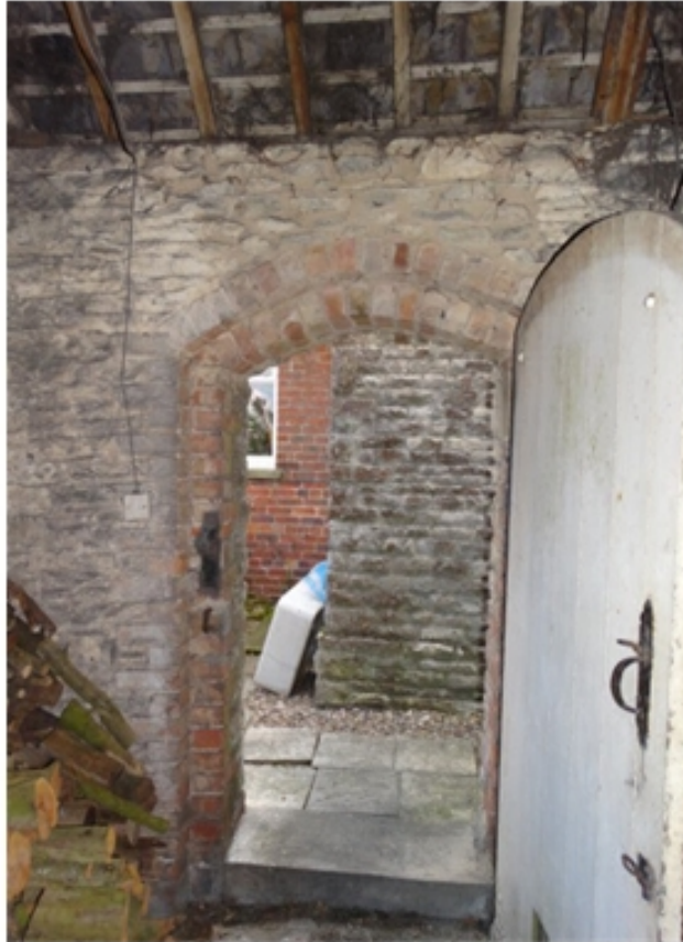
Plate 64 : Inside the Coal House looking south at the entrance door brick rebate...01.08.16.
