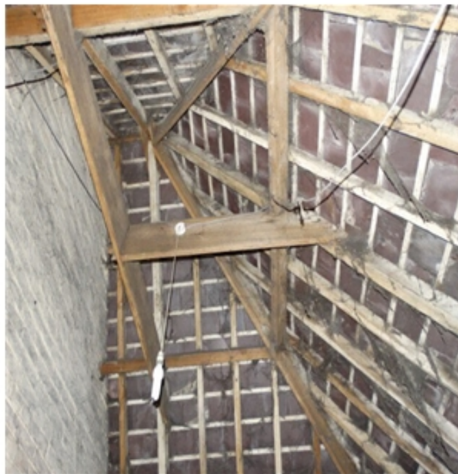
Plate 63 : Inside the Coal House looking at the roof timbers...01.08.16.
