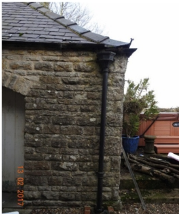
Plate 67 :south east corner of the Coalhouse : cast-iron rainwater downpipe ...13.02.17.
