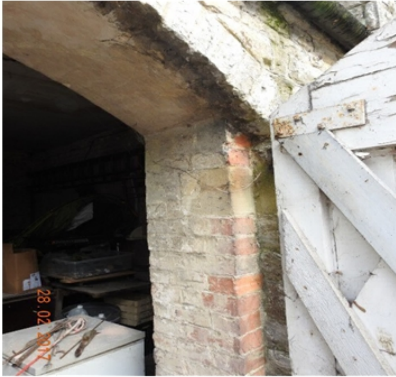
Plate 9 : Outside the Coach House double doors r.h. side rebate...28.02.17.
