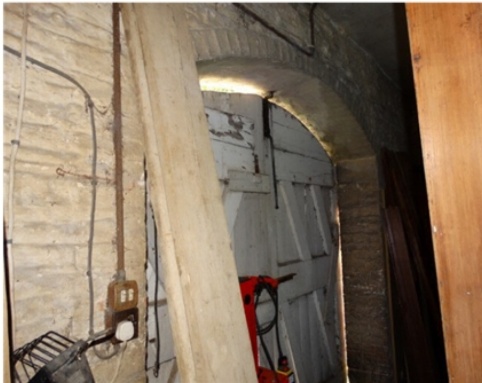
Plate 4 : Inside Coach House Double Doors (south wall) : 01.08.16.
