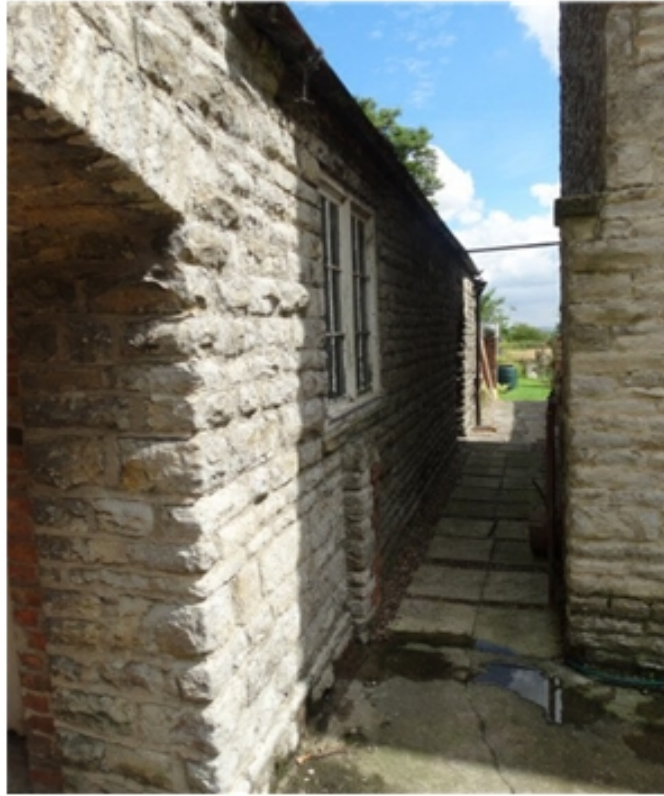
Plate 41 : South side wall of the Stables showing window and path leading to Coalhouse
