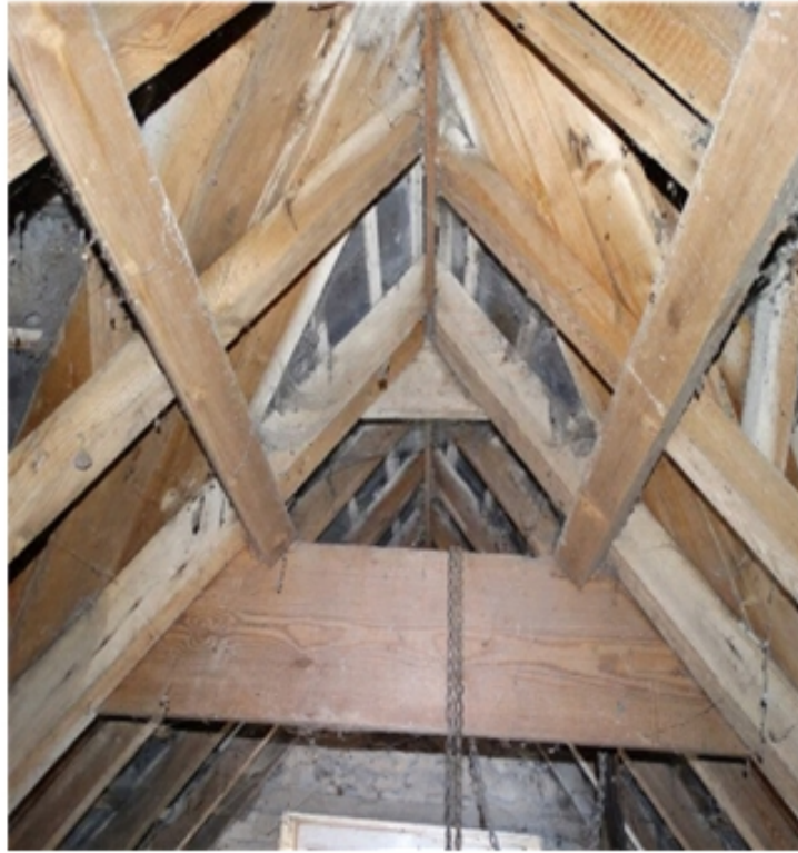
Plate 34 : Inside the Hayloft looking south, showing the valley boards and main ties : 24.08.16.
