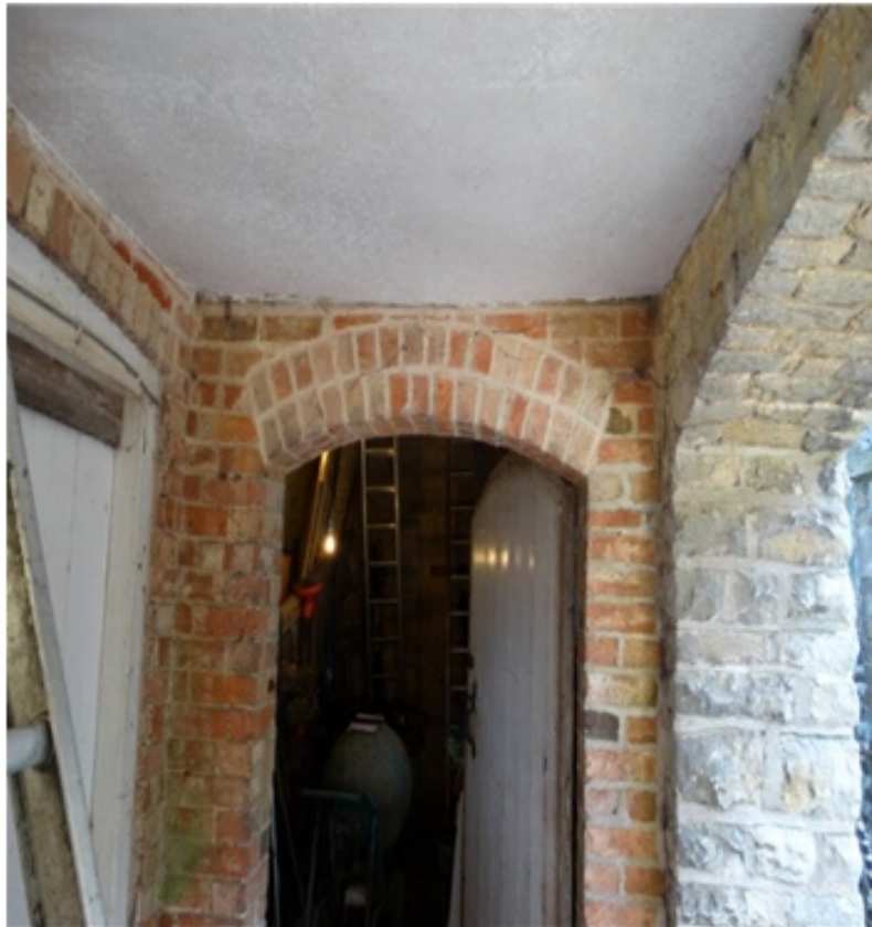
Plate 51 showing the entrance door to the Stables from the lobby...24.08.16.
