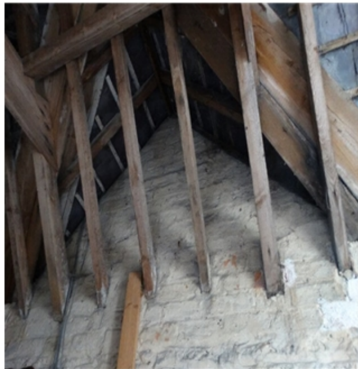
Plate 35 : inside the Hayloft showing the east facing wall roof timbers : 24.08.16.
