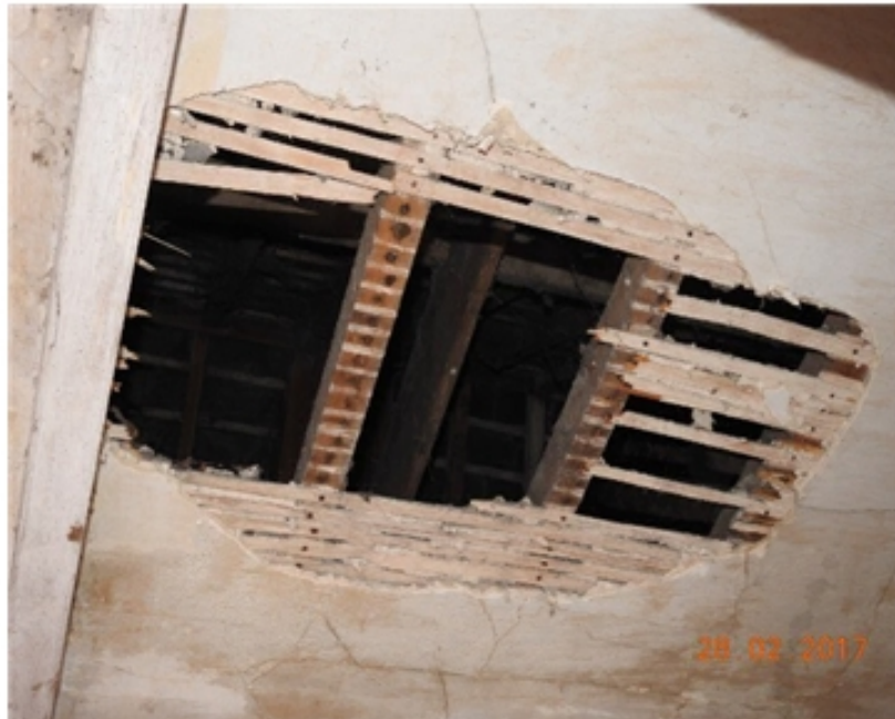
Plate 8 : Inside the Coach House : lath and plaster ceiling near roof beam...28.02.17.
