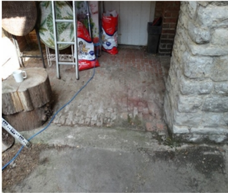
Plate 22 : Lobby/Entrance to Saddlery : outside south side : 24.08.16.
