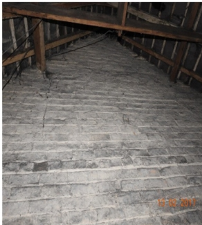
Plate 69 :inside the coalhouse looking at the division wall and roof next to the Stables...13.02.17.
