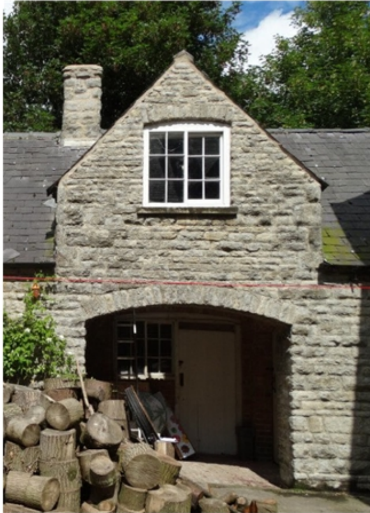
Plate 18 : Saddlery entrance and lobby : south side under Hayloft...01.08.16.
