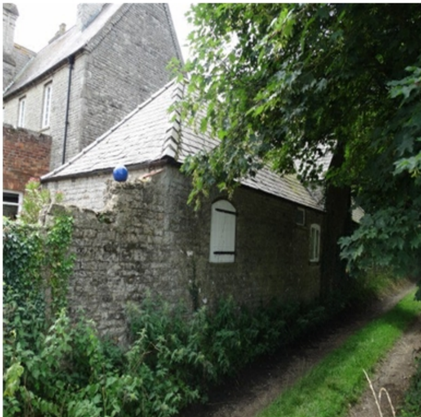
Plate 65 : north east corner of the Coal House adjacent to Carr Lane...01.08.16.
