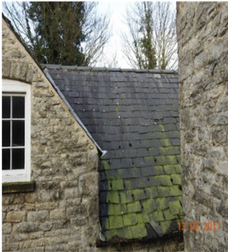
Plate 57 : Stables Roof at junction with Hayloft.....13.02.17
