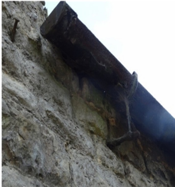
Plate 53 outside the south wall of the Stables showing the cast-iron gutter and brackets...24.08.16.
