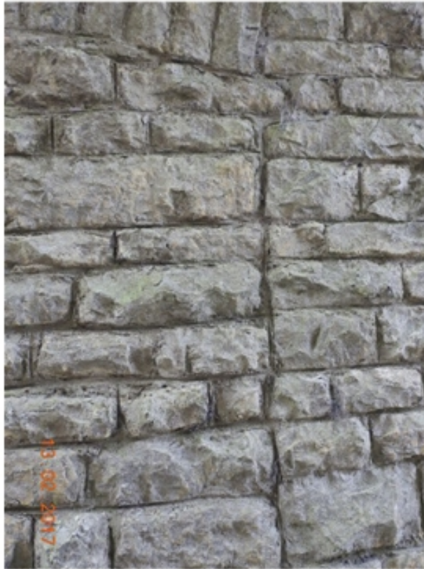
Plate 55 Outside the Stables showing former window opening in south wall...13.02.17.
