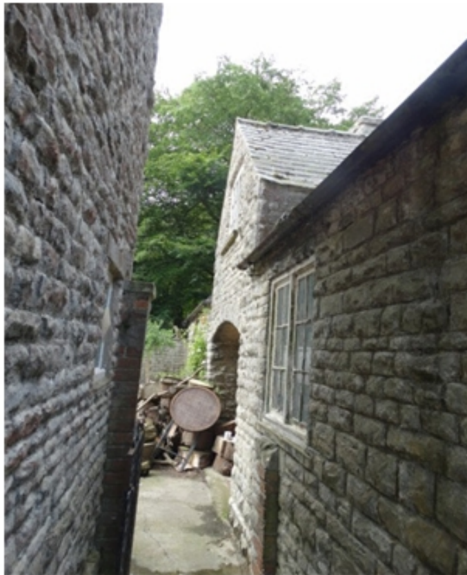
Plate 42 showing south wall of Stables looking west at window...01.08.16.
