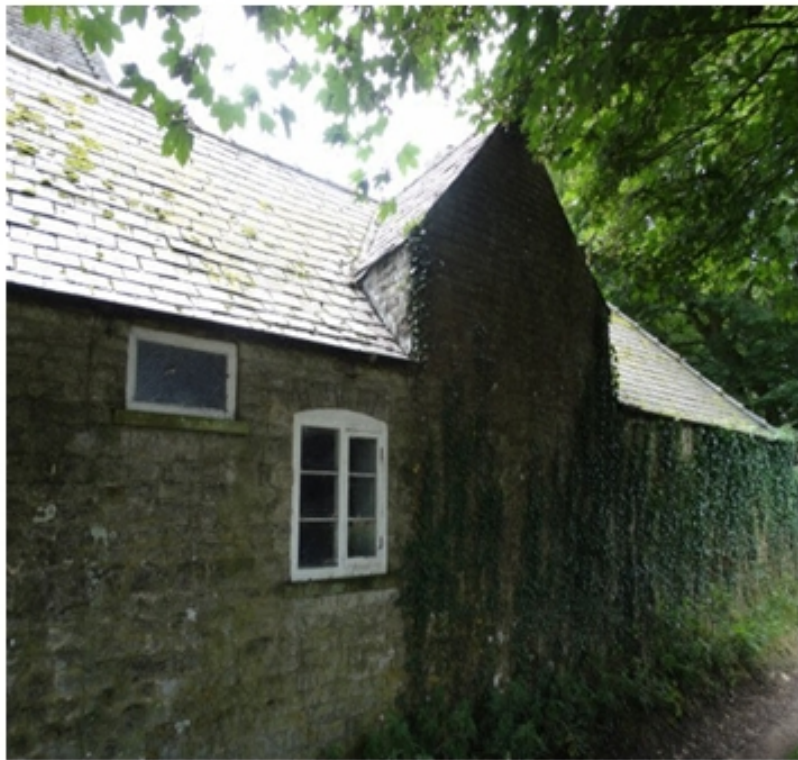
Plate 21 : Outside the Saddlery north-facing wall...01.08.16.
