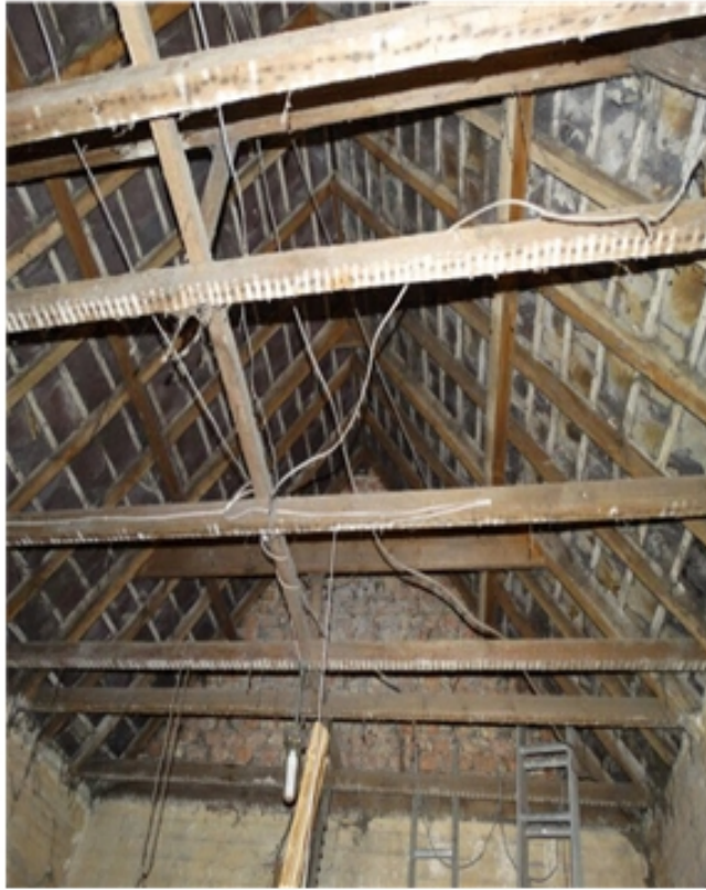
Plate 43 showing the Stables roof timbers looking east towards the Coalhouse :01.08.16.
