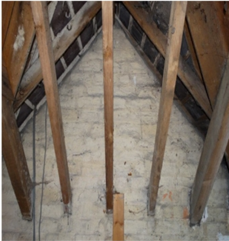
Plate 32 : Inside the Hayloft : west facing wall roof timbers : 24.08.16.
