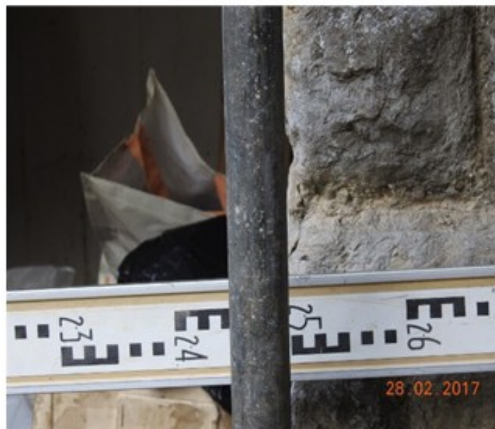
Plate 25 : width on outside of opening at entrance to lobby to Saddlery : 28.02.17.
