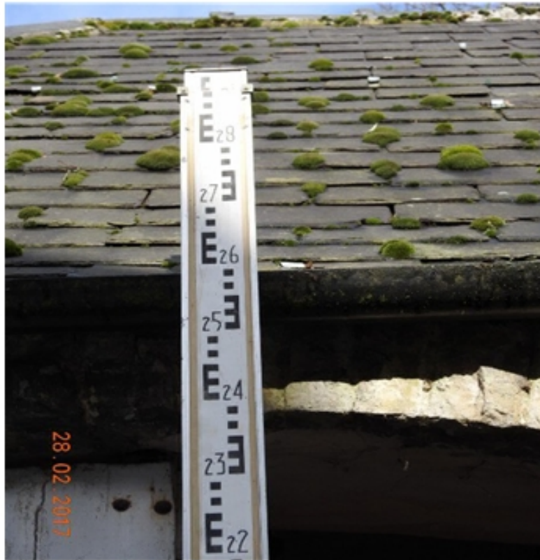
Plate 13 : Coach House eaves height on centre-line of double doors : 2.6 metres...28.02.17.
