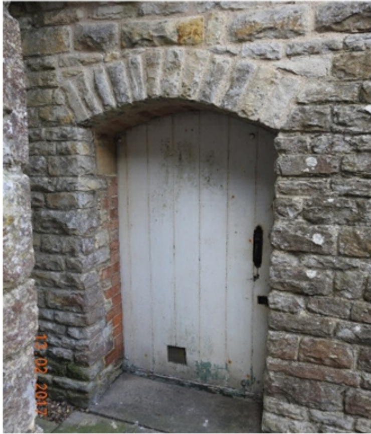
Plate 66 : outside the Coalhouse Entrance door (south wall)...13.02.17.
