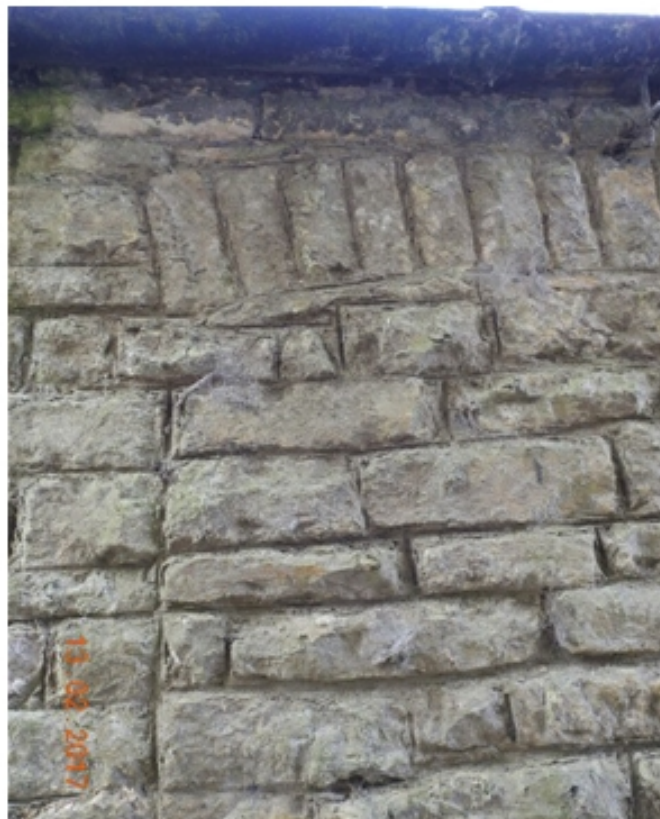
Plate 54 outside Stables south wall showing former window opening and arched lintel...13.02.17.
