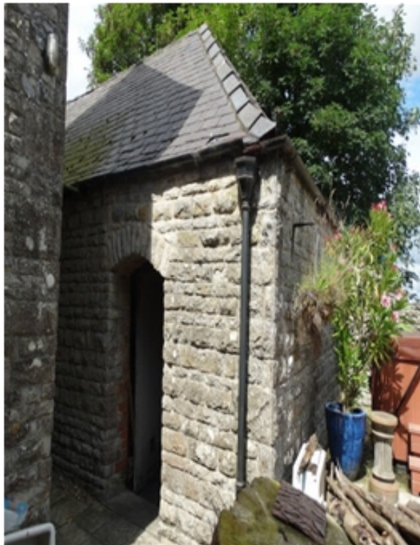
Plate 61 : Entrance to Coalhouse at the south -east corner ...01.08.16.
