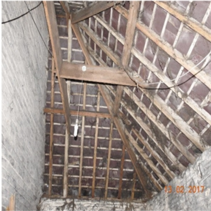
Plate 70 :inside the Coalhouse looking at the roof hipped end timbers....13.02.17.
