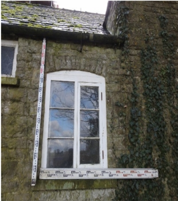
Plate 59 : Outside the north side of the Stables showing the main window....28.02.17.
