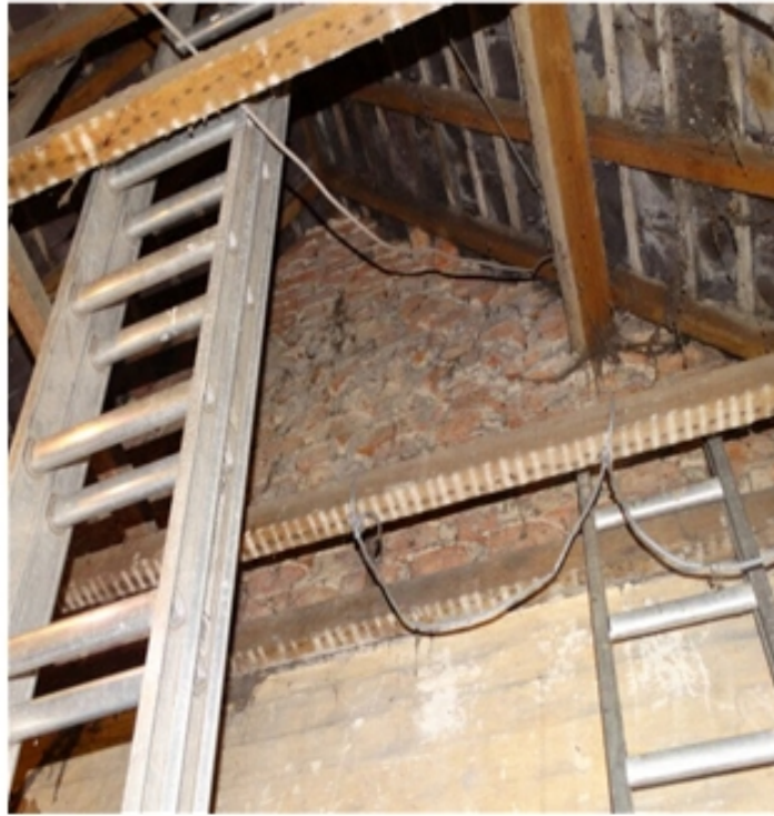
Plate 49 inside the Stables looking at the east division wall with the Coalhouse...24.08.16.
