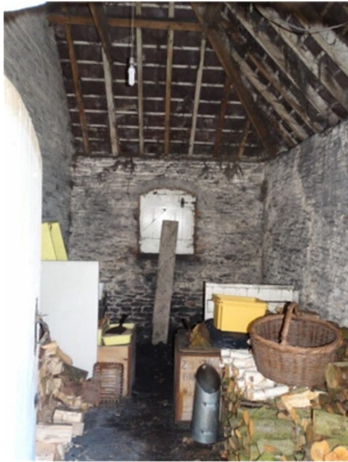
Plate 62 :Inside the Coal House looking at the north facing wall
