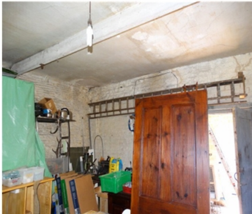
Plate 6 : Inside the Coach House : east wall hand door and roof beam...01.08.16.
