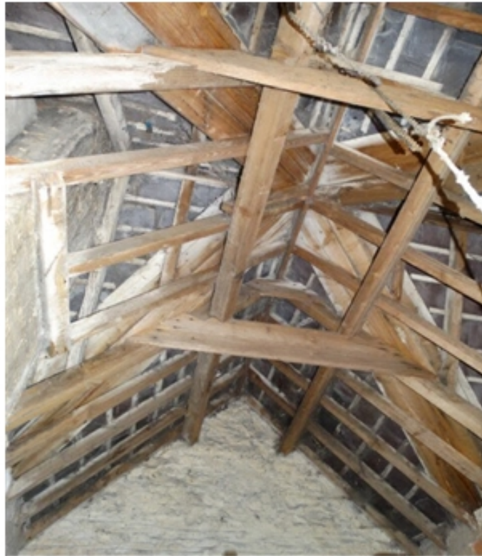
Plate 28 : Inside Hayloft looking north at valley boards at coach house (left) and stable roof (right) abutment : 01.08.16.
