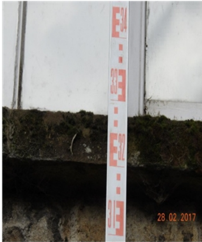
Plate 38 : Outside height of stone cill to Hayloft south facing window : 3.2metres aboveground level...28.02.17.
