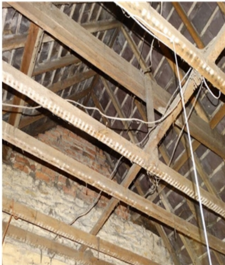
Plate 50 inside the Stables looking at the roof timbers and west side division wall..24.08.16.
