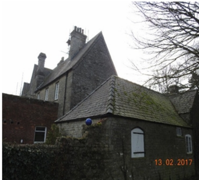
Plate 75 : north east corner of the Coalhouse adjacent to Carr Lane..13.02.17.
