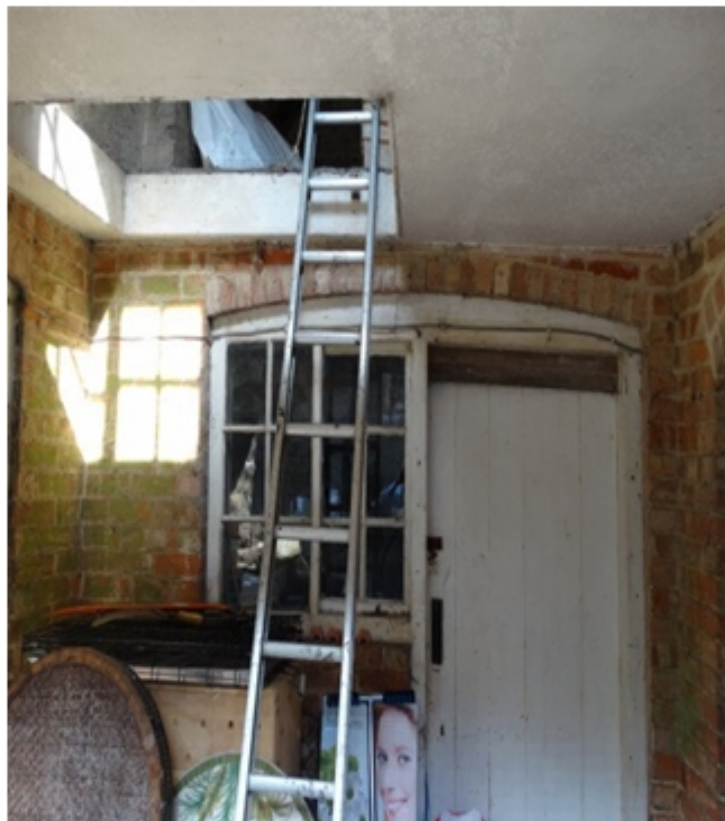
Plate 27 : Outside the south side of the Saddlery Entrance screen : 24.08.16.
