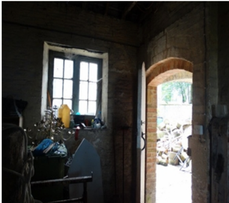
Plate 46 inside the Stables looking south : showing the entrance door and window : 01.08.16.
