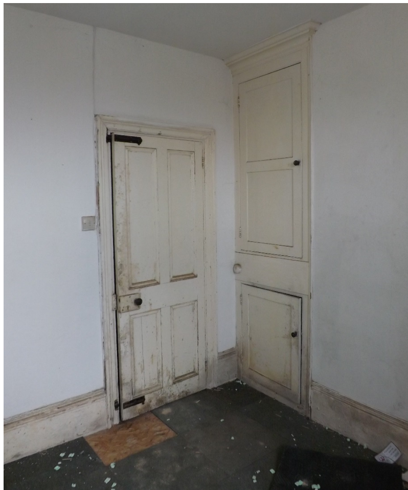
Fig 15: Room G2, typical four-panelled door and floor-to-ceiling cupboards
