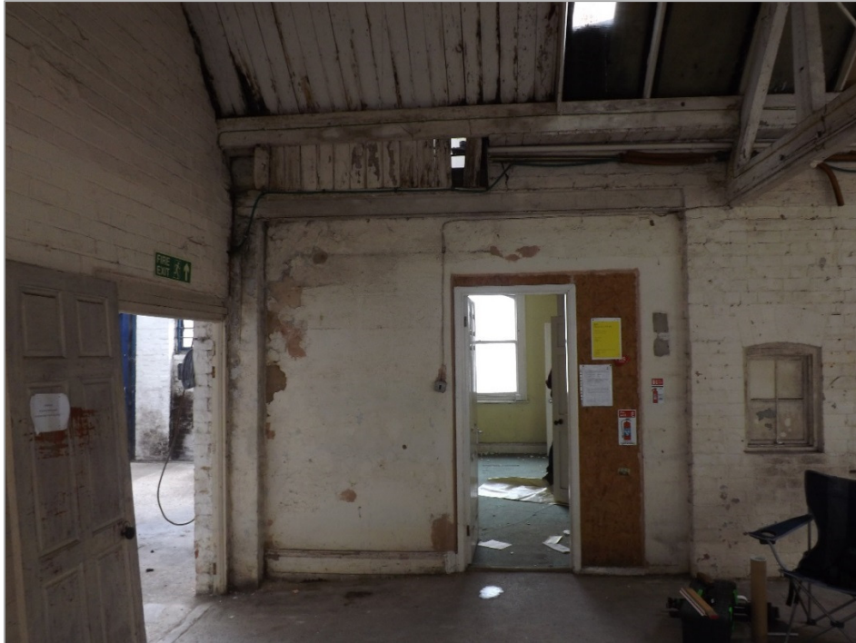
Fig 12: Entrance from factory into G1; note the RSJ above and small painted-up window on right.
