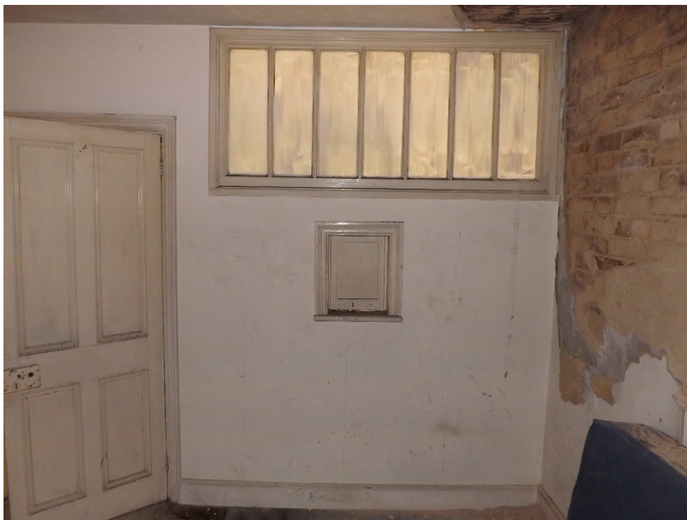
Fig 20: Borrowed light window and hatch, room F3; room F2 beyond
