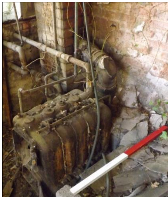
Fig 25: The Robin Hood boiler serving Building 9 (Greenhouse); scale 1m
