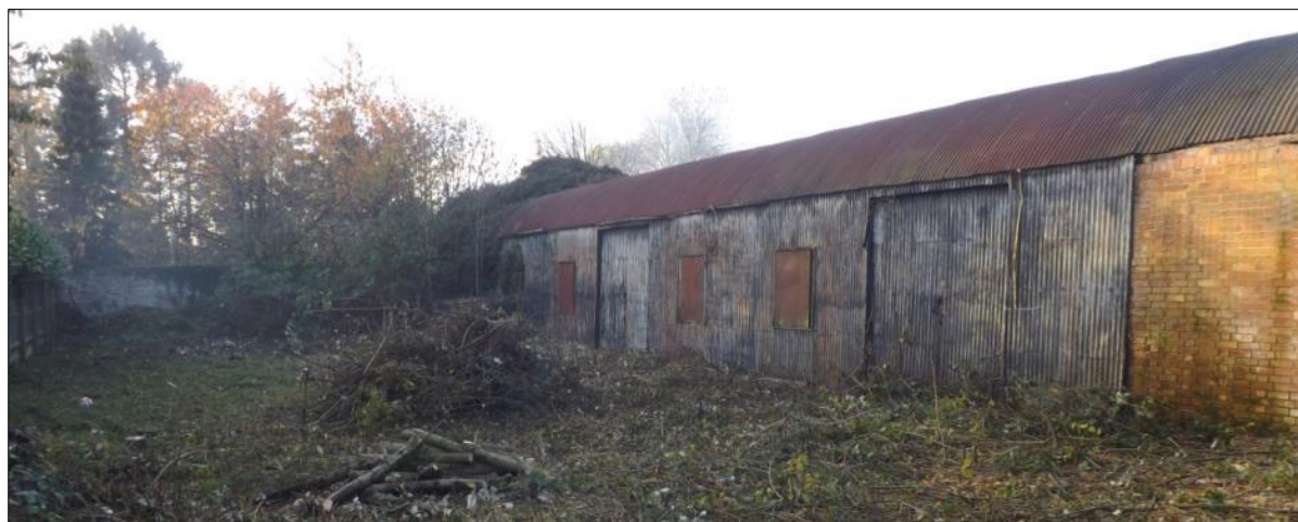
Fig 22: The southern, corrugated tin wall of Building 8; the brick bay on the right (east) is an extension.
