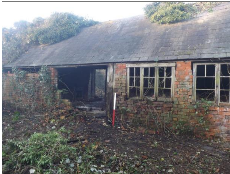
Fig 14: Building 2, south wall. Left half brick in-filled for pigs, leaving a ventilation slot; right half re-adapted for potting; scale 1m
