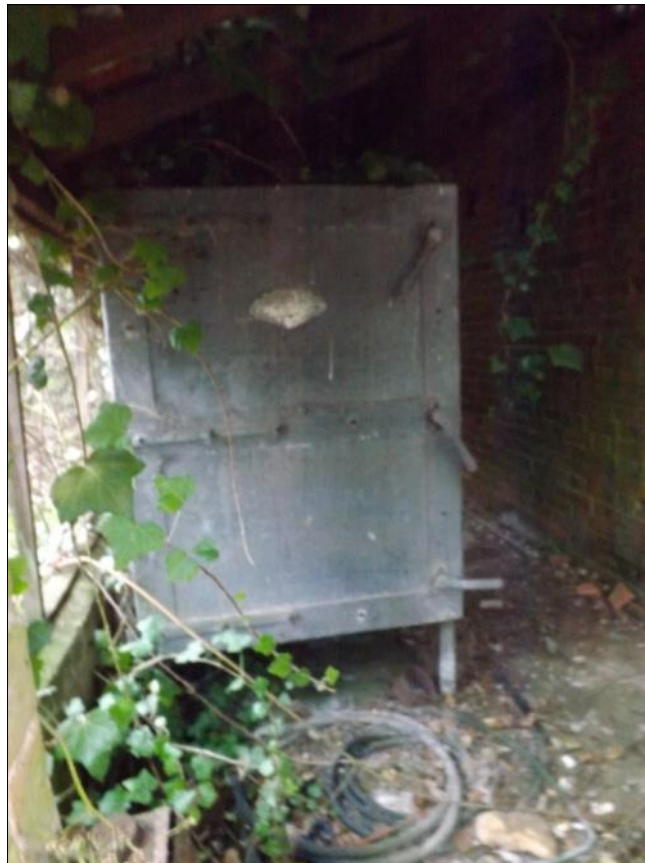
Fig 26: A galvanised steel seed-safe taking up most of Building 10's centre bay
