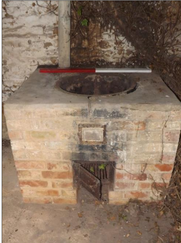
Fig 15: Building 2, the inserted copper; scale 1m
