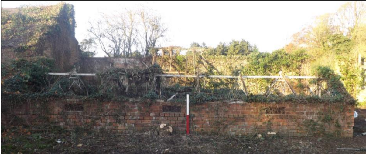
Fig 18: Building 3, Cucumber House, south side. Note the cast-iron trusses and steady iron ridge-pole; scale 1m
