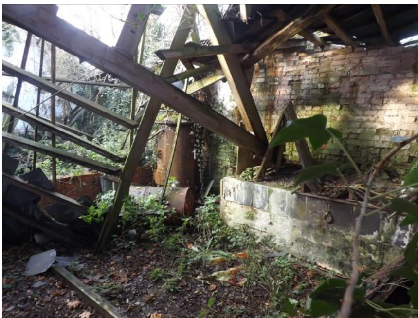
Fig 12: The eastern half of Building 1 in a state of collapse; the boiler in the background is named 'Perkins Jubilee 1935 Derby England', and is Jubilee no 04944/2.
