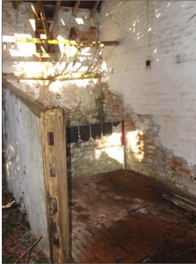
Fig 10: Building 1, surviving stall with trough and hayrack; ventilator above
