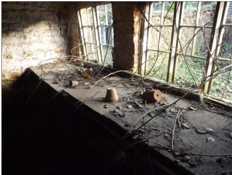
Fig 16: Building 2 interior, as abandoned potting shed; old doors formed the staging
