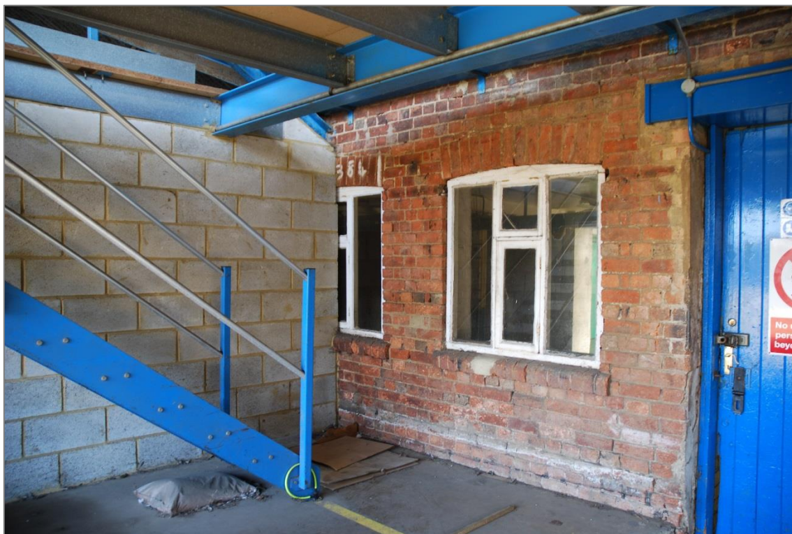
Fig 33: The possible 1879 range, with inserted loading bay doors and modern steel and breezeblock extension adjoining
