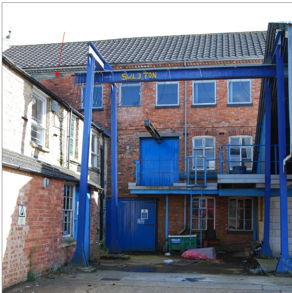
Fig 31: North-western elevation of factory, looking south-east, showing change in brick colour
