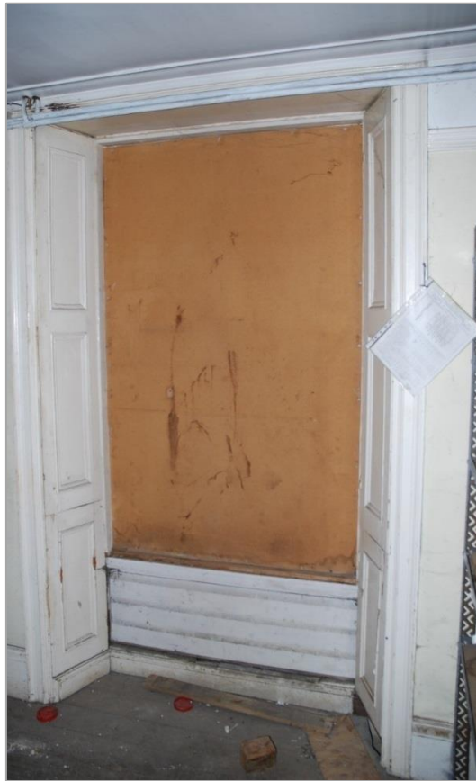
Fig 26: Splayed window with nailed-up shutter boxes, room G12
