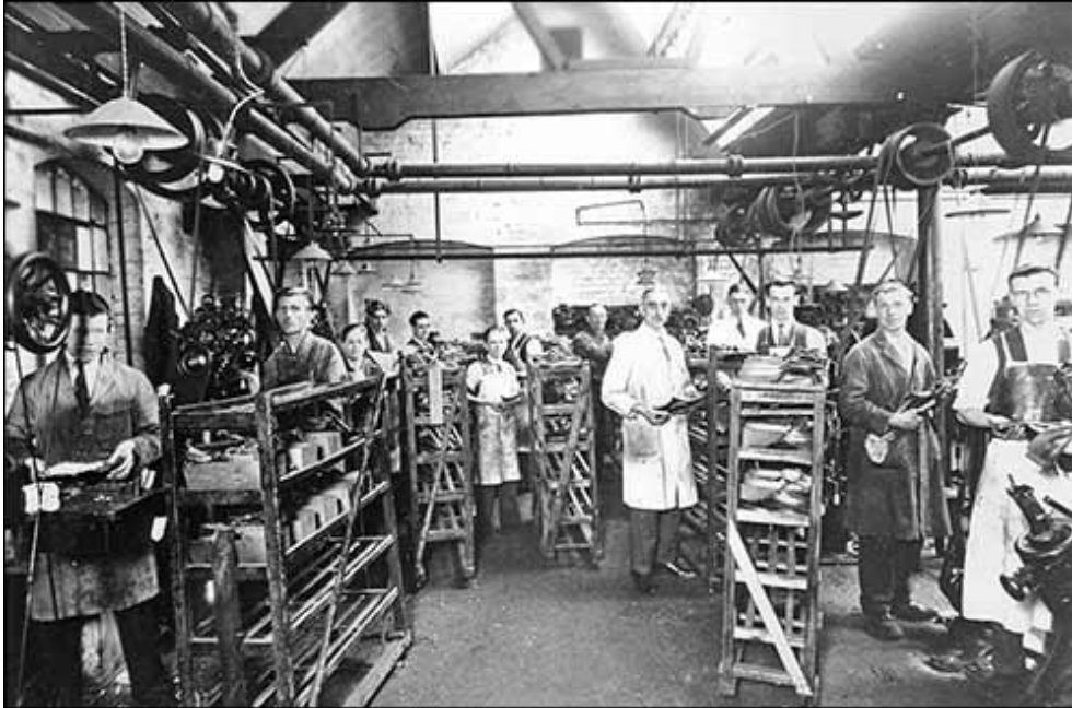
Fig 12: Interior of the north-light sheds (G3), with overhead belt drives ( rushdenheritage.co.uk )
