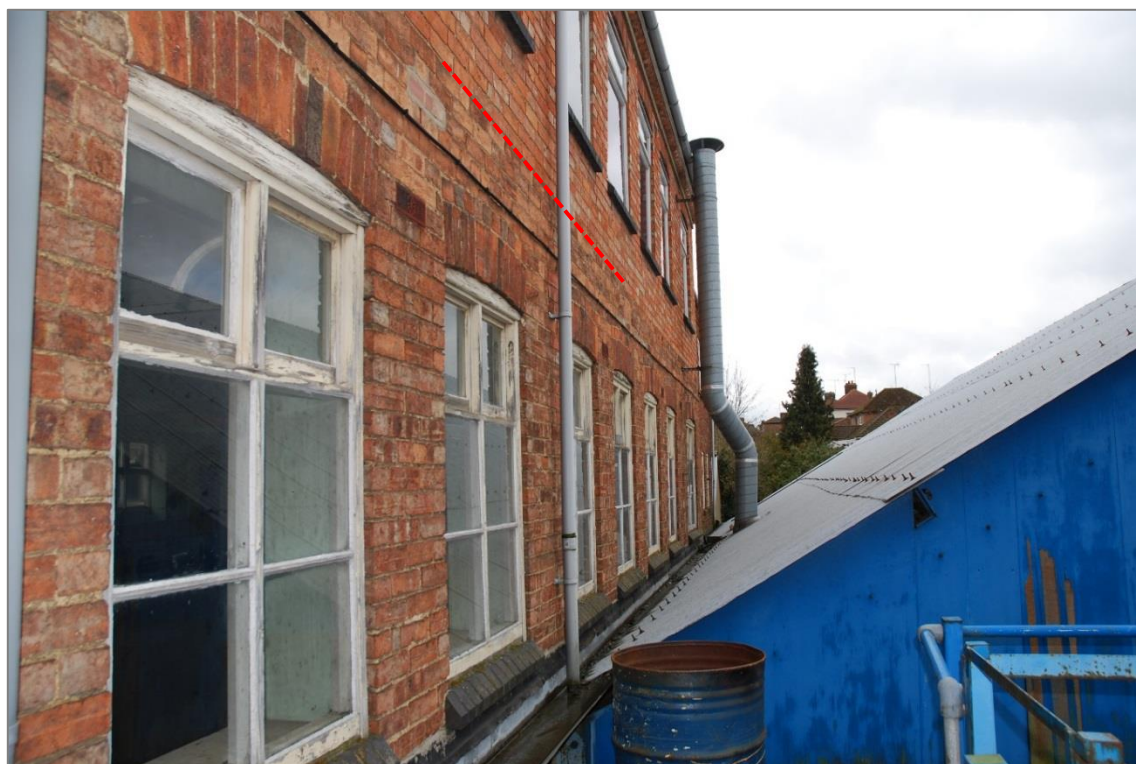
Fig 30: The north-western elevation of the 1889 range, showing change in brickwork from first to second storeys, looking south-west
