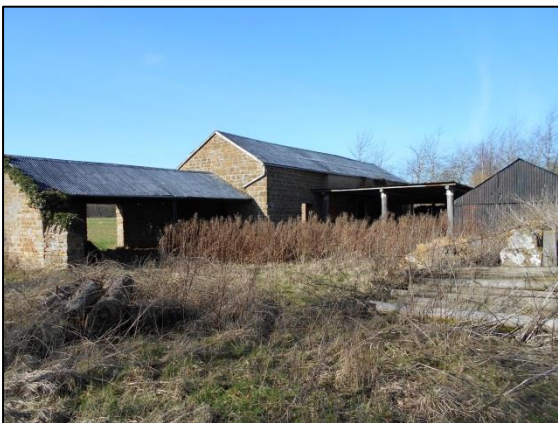
Fig 5: The barn, viewed from the south-east
