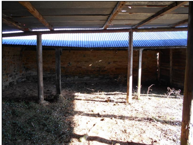
Fig 23: Cattle shelter, looking east from Barn A
