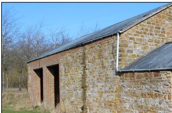
Fig 8: Barn A/B; modern west wall exterior
