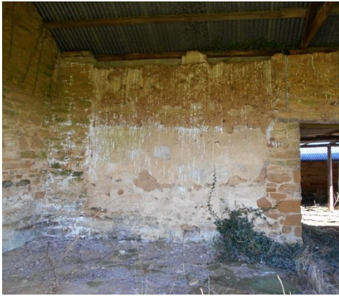
Fig 10: Left (north) cob panel in east wall
