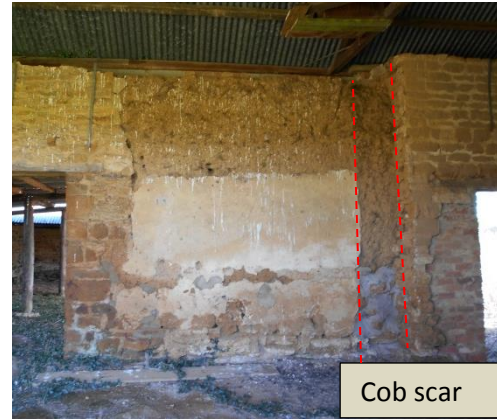
Fig 11: Right (south) cob panel in east wall
