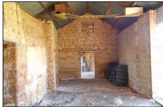
Fig 9: Barn A/B; modern west wall to right
