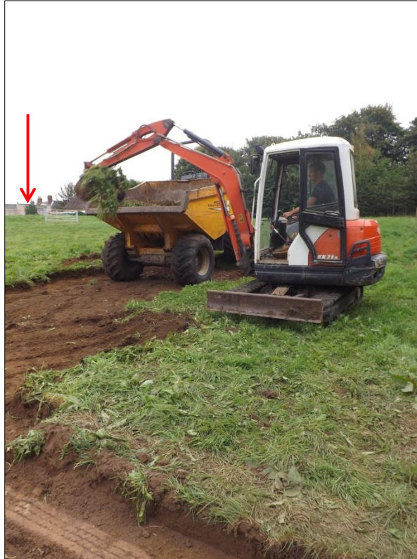
Fig 4: Stripping the turning-head. The new stable location is in the background at the top of the rise (arrowed)
