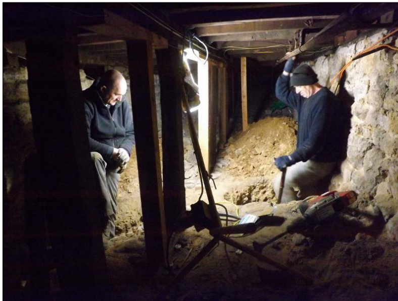
Fig 9: The sub-floor environment during digging of Test Pits B5 and B6
