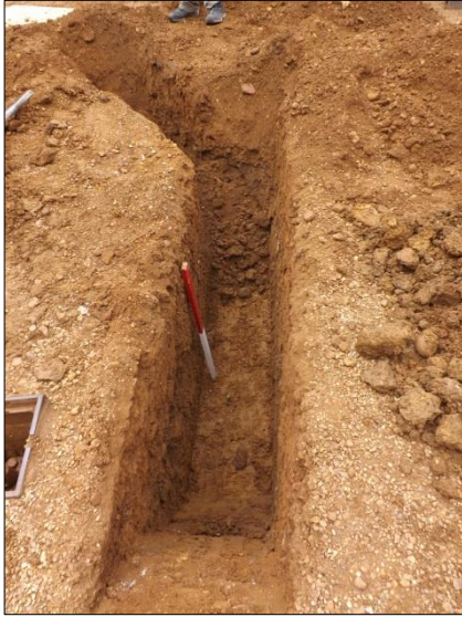
Test Pit G1, looking west
