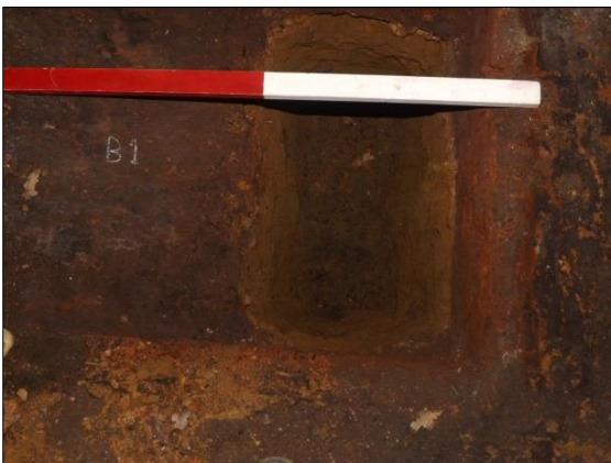
Test Pit B1: Concrete directly onto natural clay
