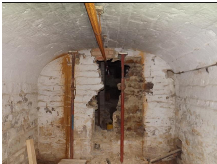
Fig 4: One of the new doorways during cutting works, vaulted cellar, looking west
