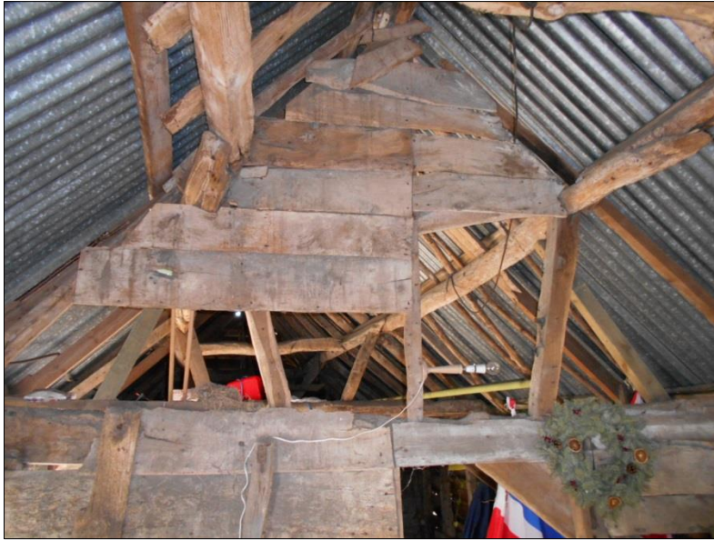
Fig 8: the weatherboarding right up to the ridge, dividing Bay 1 from Bay 2; looking south
