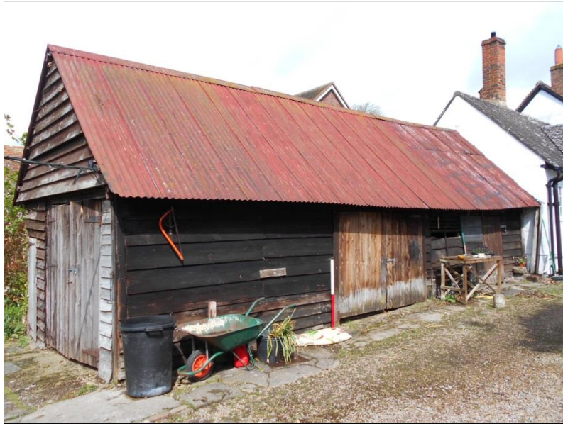
Fig 3: The outbuilding from the south-east; scale 1m
