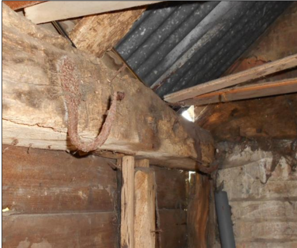
Fig 6: Bay 1 West side, butcher's hooks on wall-plate
