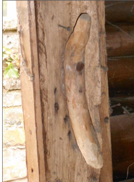
Fig 7: Bay 1 West side, rustic cleat for fixing a hoisted weight
