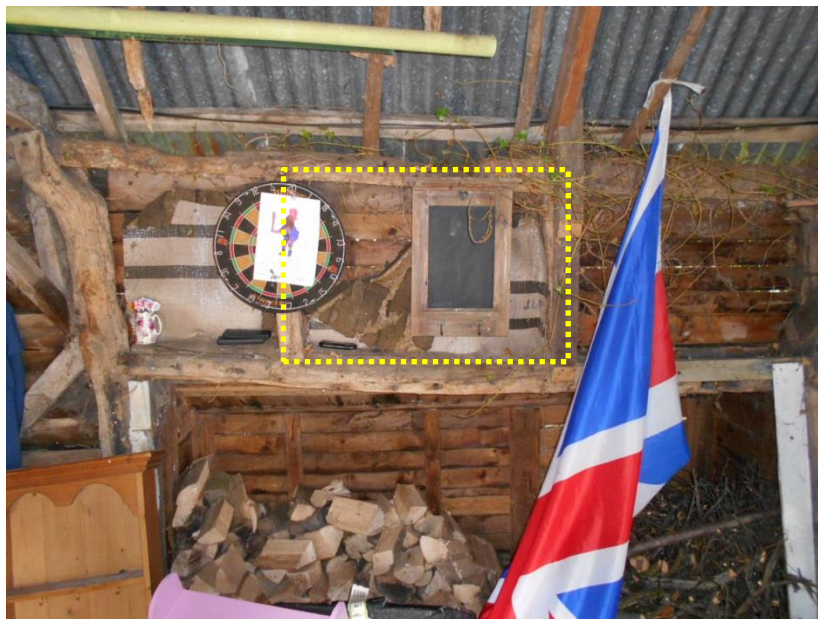
Fig 9: Possible former window; outshut below; the midrail is sagging where its supporting upright has been taken out – the empty mortise remains in the soffit
