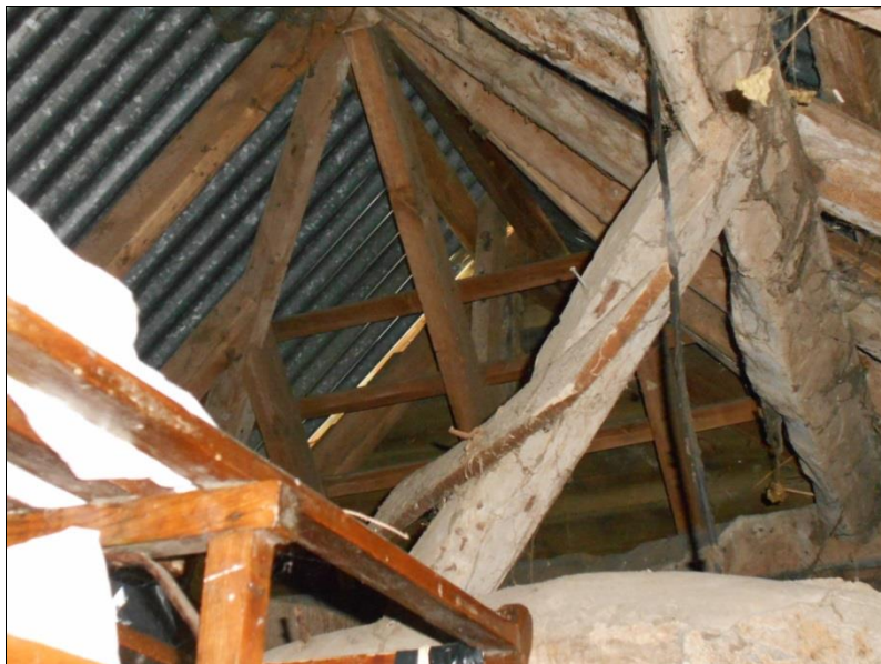
Fig 4: The angled frame which once supported the thatched hip of the south gable
