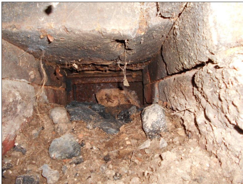
Fig 11: View through the flue within the wall, showing the buried cast-iron door on the exterior of the orangery. It is littered with unburnt coal and coke fragments.
