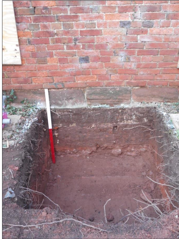
Fig 3: One of the foundation trenches for the angled buttresses; scale 1m
