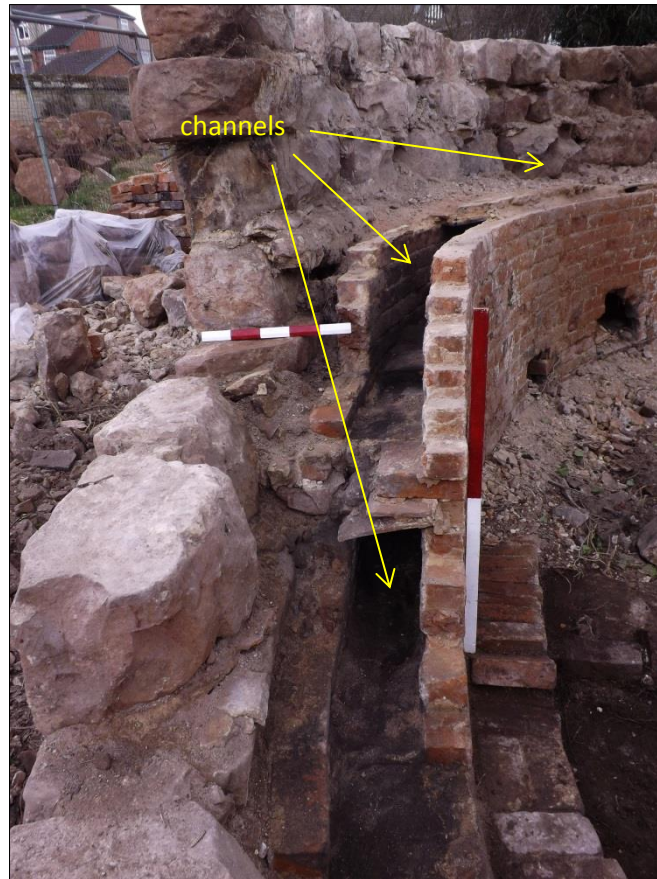
Fig 4: The orangery wall at the point of maximum dismantling; scales 1m and 50cm
