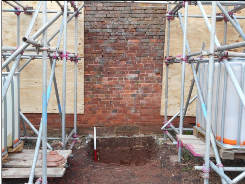
Fig 2: Buttress foundation hole between two temporary weighted wall-supports
