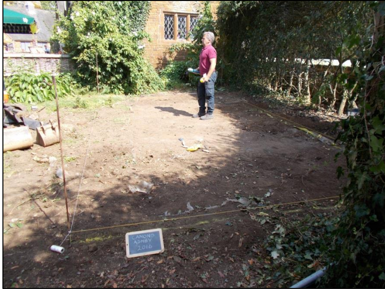
Fig 2: Setting out the building relative to the holly hedge and the roadside wall beyond (right)
