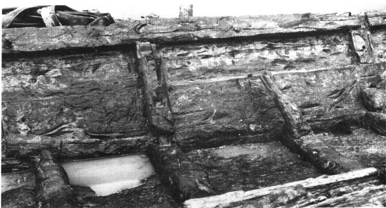
Fig 21 Barge Zwammerdam 2: starboard side. Fork-ended ribs are placed in alternate positions; the uprights are slotted into the smooth ends of these ribs (photo IPP: F Gijbels)
