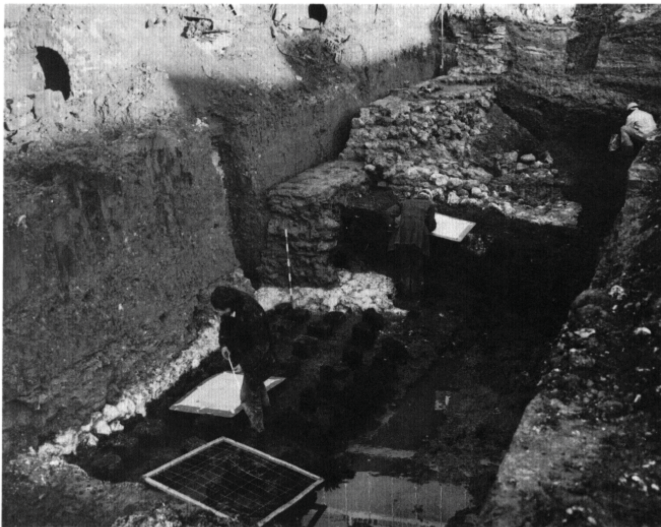
Fig 72 London: lower part of the riverside defensive wall, as excavated at Blackfriars in 1975. The ragstone superstructure lay upon a foundation of oak piles and chalk blocks. The date of this part of the wall is disputed, but it may be of the 3rd or early 4th century (Photo: T Hurst)
