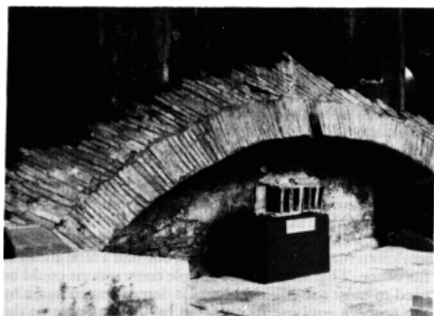
Fig 29 Brick rib from the vault of the Great Bath at Bath (Photo: author)
