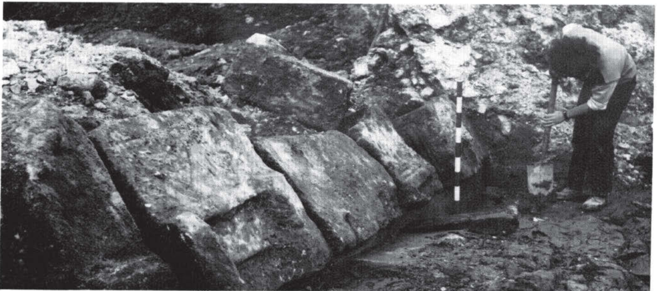
Fig 73 London: at Blackfriars and in the Tower of London have been found parts of late Roman riverside defences which contain reused stones, as in this portion of collapsed wall at Blackfriars. This seems to be of different construction, and of a different building phase, from the wall shown in Fig 72, and may date from the late 4th or early 5th century (Photo: J Maloney)
