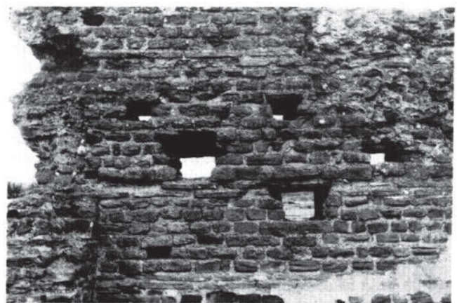
Fig 36 The 'Old Work' at Wroxeter, showing petit appareil with tile bonding-courses and putlog holes passing right through the wall. Some of the holes perhaps served for the construction of centering for the vault, not simply for scaffolding (Photo: author)
