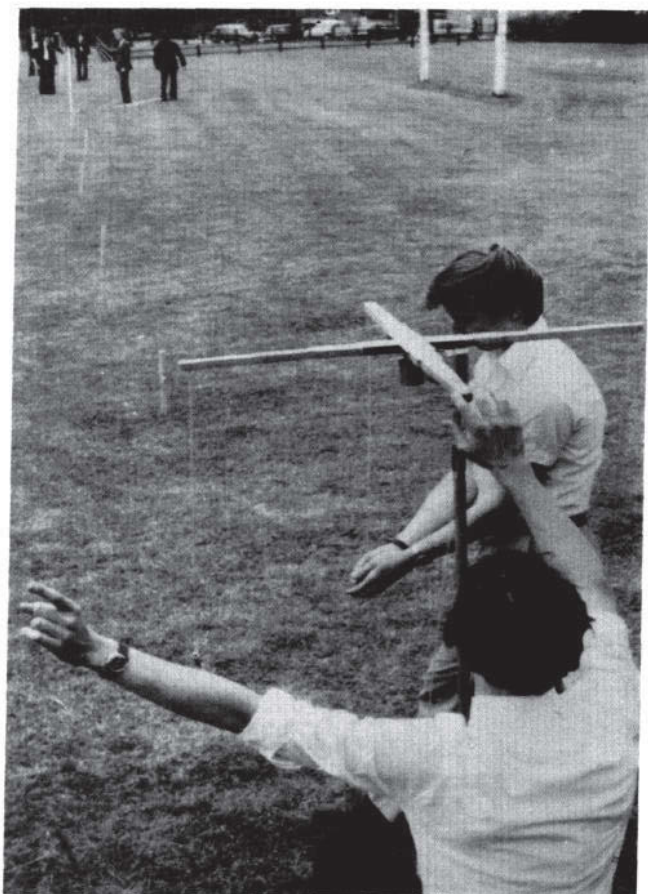
Fig 11 Boys of Silcoates School, near Wakefield, using a model groma made by the Wakefield Schools Museum Service. It is a copy of the groma found in the workshop of Verus at Pompeii, and the exercise demonstrated its reliability, except in strong winds
