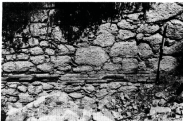
Fig 28 Mortared rubble work with tile bonding-courses in a bath building at Oenoanda in Lycia (Photo: author)
