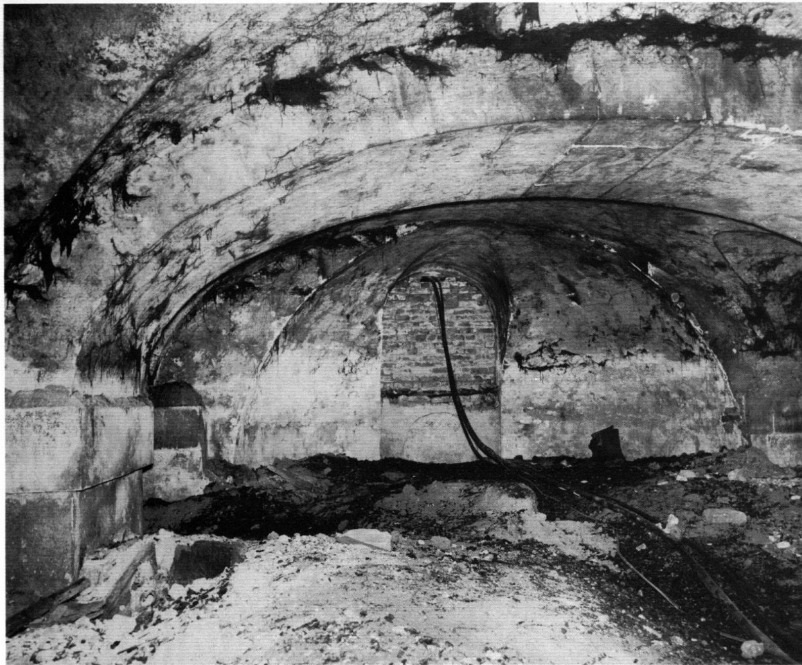
Figure 1.8 Apse at west end of parochial vault showing where the body of the church abuts the tower
