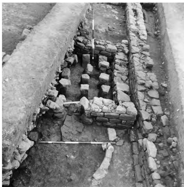
Plate 59 Catterick Bypass (Site 433) – Building VI.4b. Hypocausted Room 2 inserted in Phase 6b with praefurnium within Room 1 in foreground. View south. Scales 6ft
