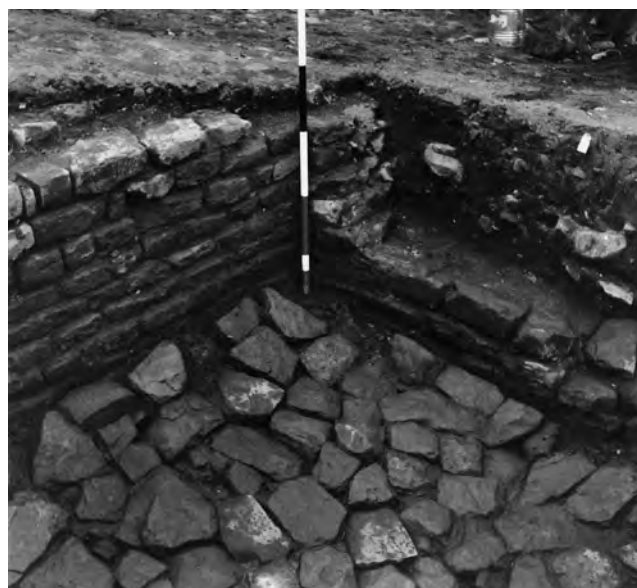
Plate 52 Catterick Bypass (Site 433) – Building III.5c. Phase 6a occupation surface within Room 3. View north-west. Scale divisions 1ft.
