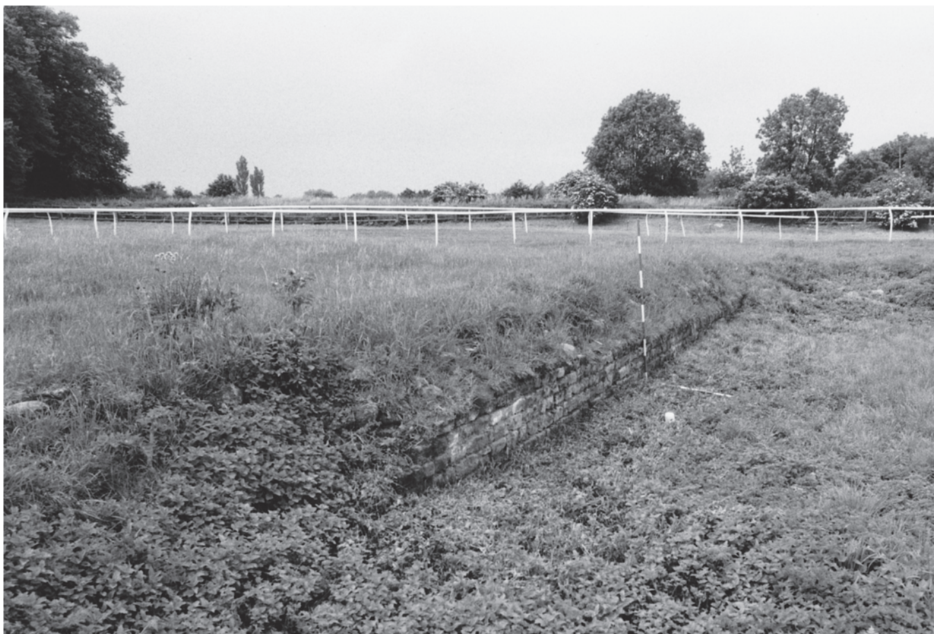
Plate 11 The east wall of the Roman town as restored by Sir William Lawson in the 19th century. View north-west
