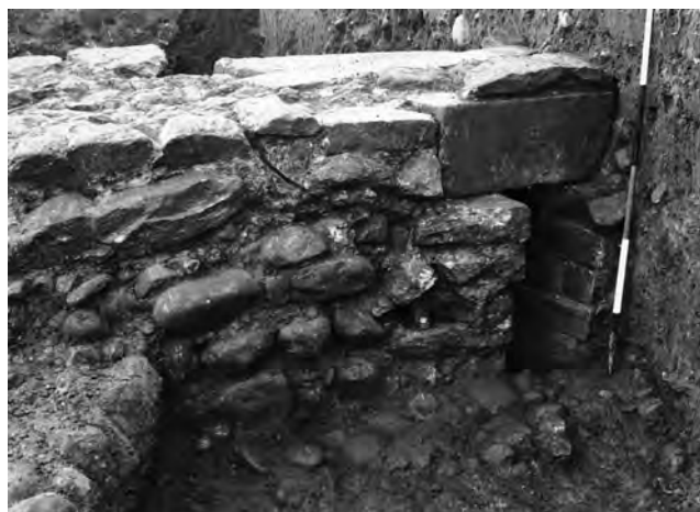
Plate 47 Catterick Bypass (Site 433) – drain through town wall in Area A showing cobble ‘raft’ foundation extending under drain on inside of the wall. View west. Scale divisions 1ft. (Photograph R H Hayes)
