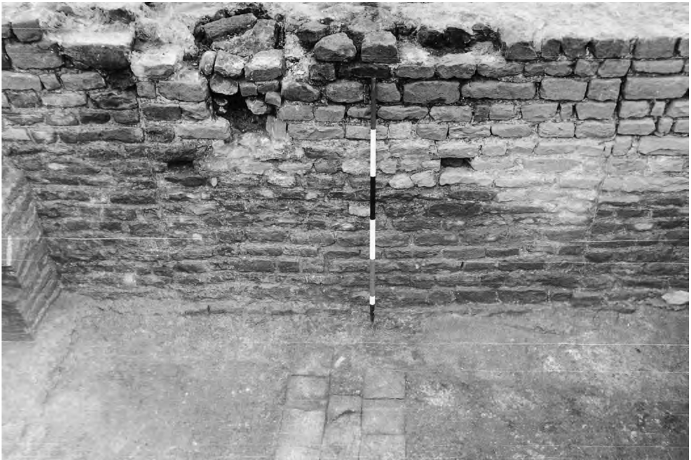
Plate 37 Catterick Bypass (Site 433) – Building III.5c. Coursed blockwork filling the gap between the two stub walls within Wall 5 on the west side of Room 2. View west. Scale 6ft
