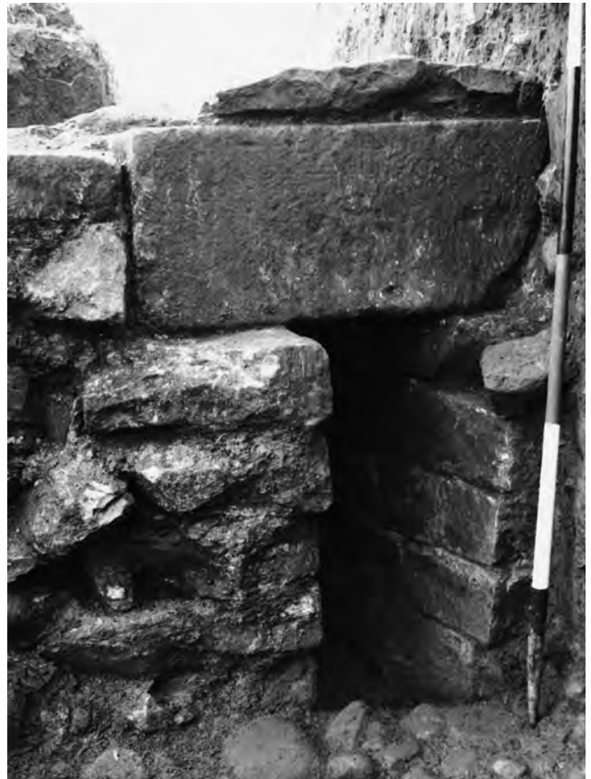
Plate 49 Catterick Bypass (Site 433) – town wall in Area A. Detail of the drain through the wall showing construction on the inner face. View west. Scale divisions 1ft. (Photograph R H Hayes)
