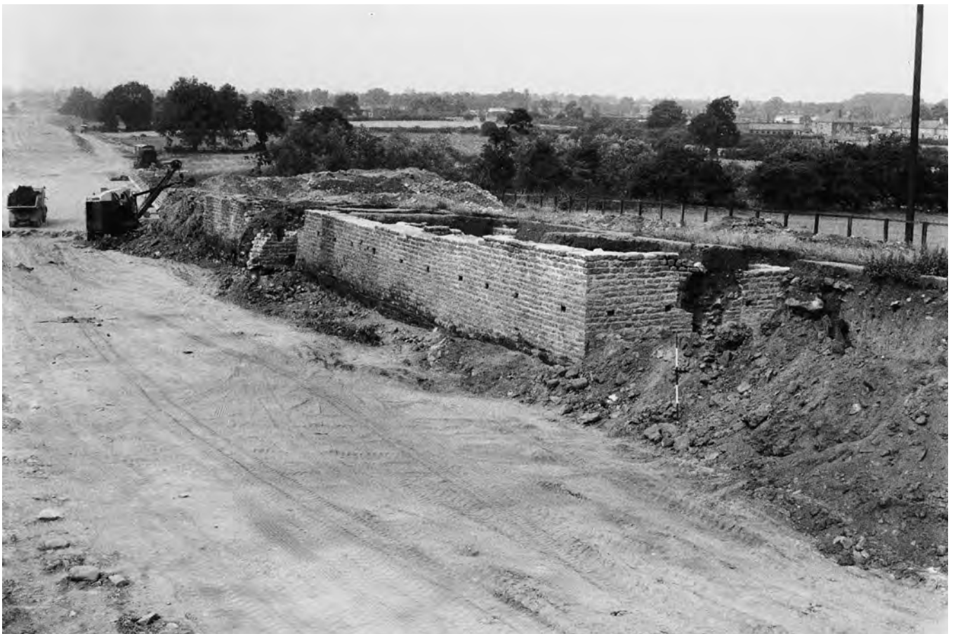
Plate 35 Catterick Bypass (Site 433) – Building III.5c after the removal of the hillside into which it had been terraced showing putlog holes. View north-east. Scale 6ft. (Photograph A McWhirr)
