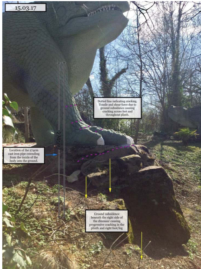
Plates 73 and 74 – Analysis of structural deterioration – Front Plinth 62
