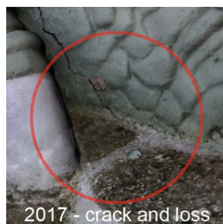
Plates 37,38,39 –Images of the digital model comparing data from 2016 and 2017, red circles identifying concrete loss. 37
