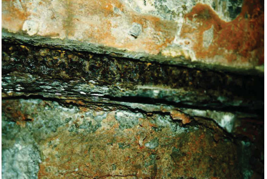
Plate 9. Corroded Iron hooping in the Iguanodon. Removed 2001 10 .
