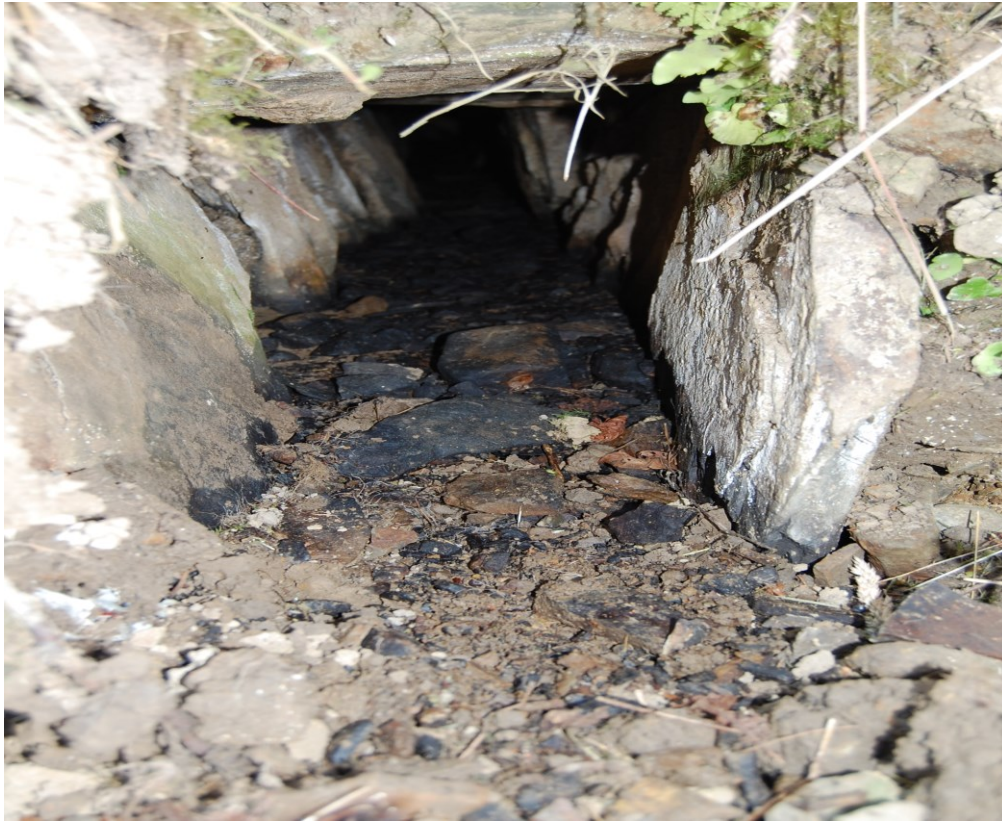
Figure 19: Close up of Stone Lined Drain in South West Corner of Garage Area.
