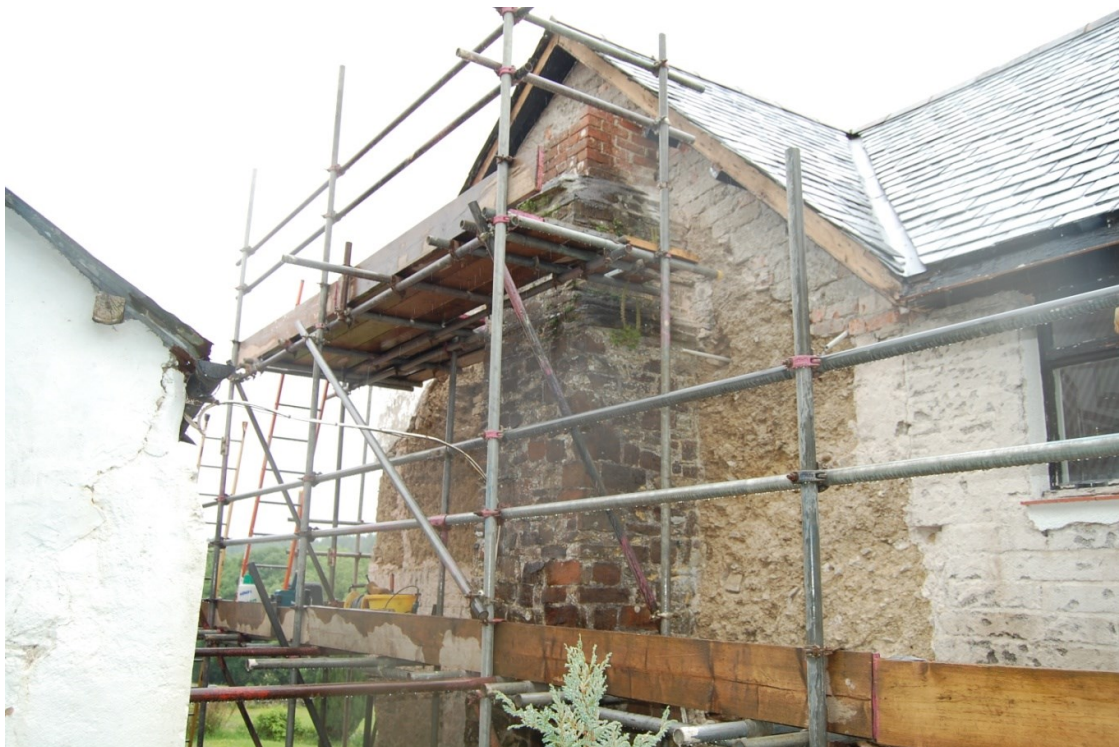
Figure 5: West Gable End Showing How the Breeze Blocks Have Been Added Above Cob
