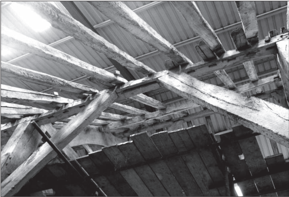
Fig. 7. Underside of the Phase 1 wall plate, showing stave-holes and the redundant mortice for braces.
