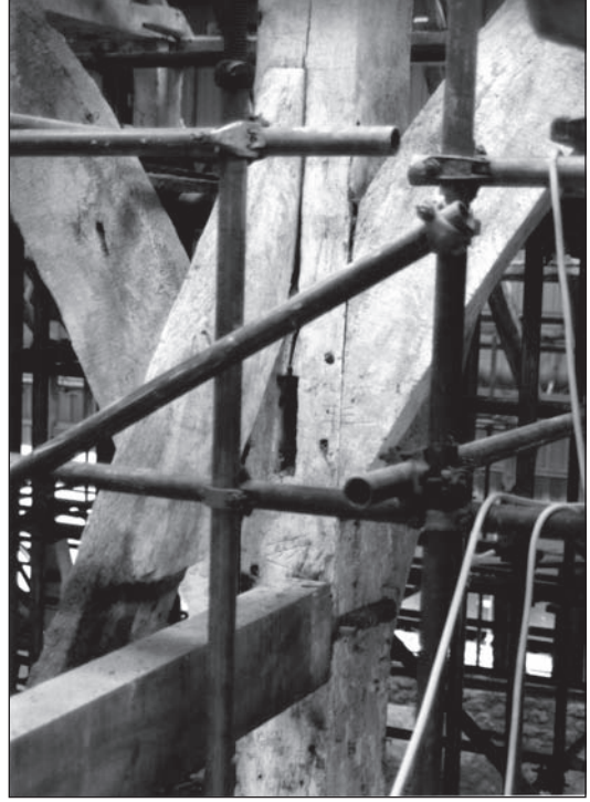
Fig. 22. Redundant mortice for the wall plate on the south side of the east porch, on the post at the east end of Truss 6.
