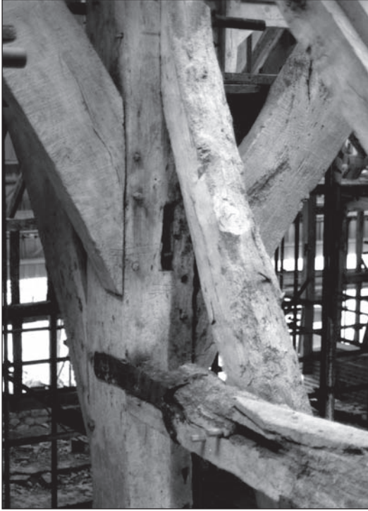
Fig. 21. Redundant mortice for the wall plate on the north side of the east porch, on the post at the east end of Truss 5. Note the remains of a peg which appear to indicate that it had been used.
