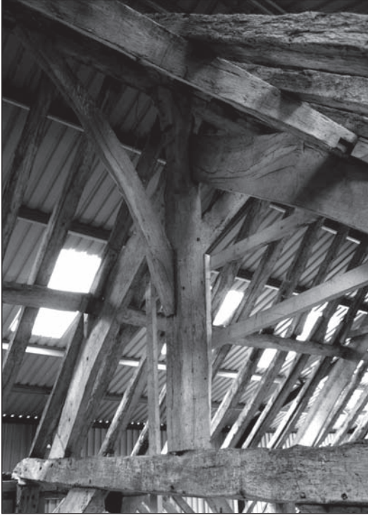
Fig. 16. Kingpost and brace assembly on Truss 4. Note the different levels at which the braces from the ridge plate attach to the kingpost, that to the left (south) is part of the Phase-1 structure, whilst that to the right (north) is part of the Phase-2 extension.
