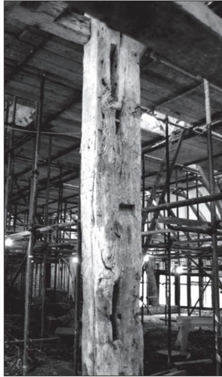
Fig. 6. The main post at the east end of Truss 5, north face, showing the redundant mortices for rail and braces, and a shoring notch.
