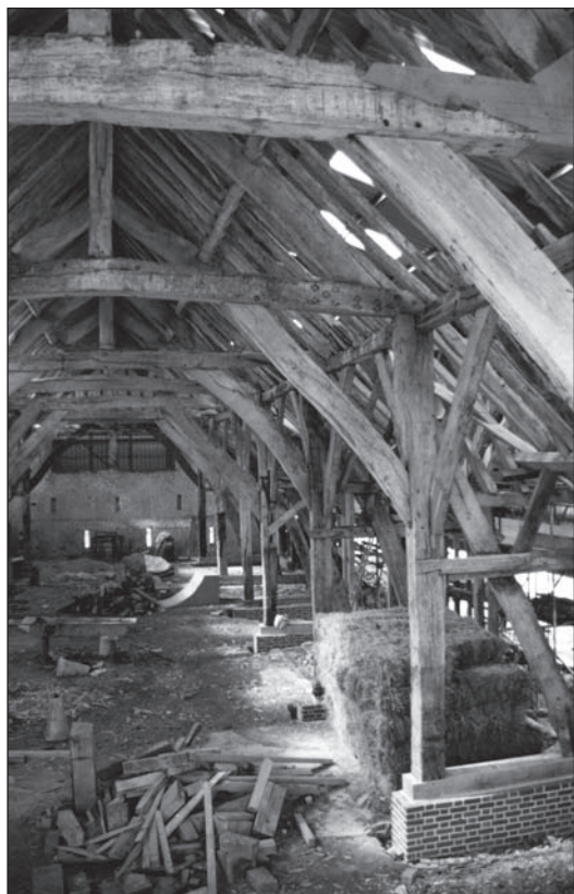
Fig. 3. Interior of the barn during repairs in 1994, looking south, with the west end of Truss 3 in the foreground.
