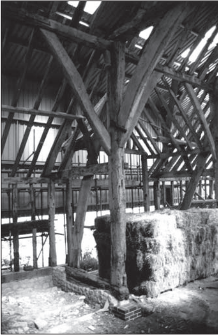
Fig. 5. The main post at the west end of Truss 4, looking northwest. Note the redundant mortices for the soleplate, rail, and braces.
