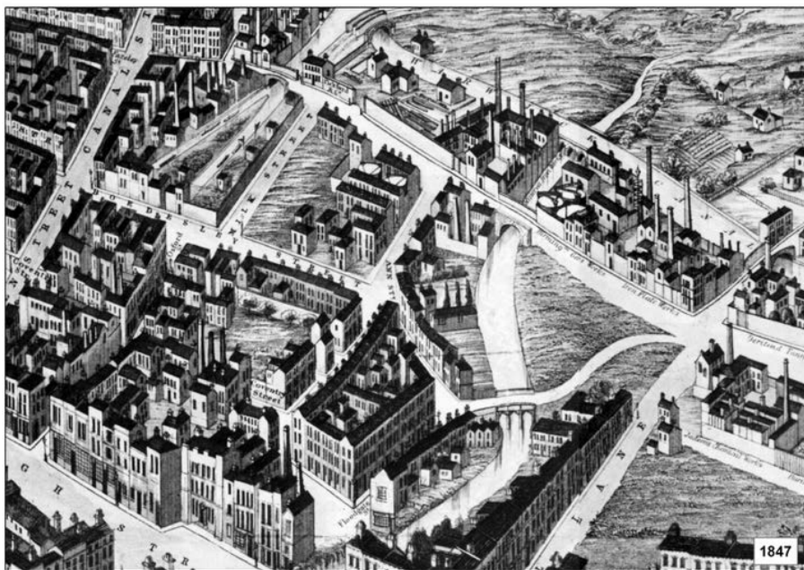
Figure 3.32 Buildings and Structures adjacent to the canal (in the vicinity of 59), Ackermans Panoramic 1847
