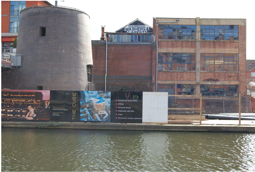
Figure 5.11. Recent regeneration works along the canal near the Mailbox.
