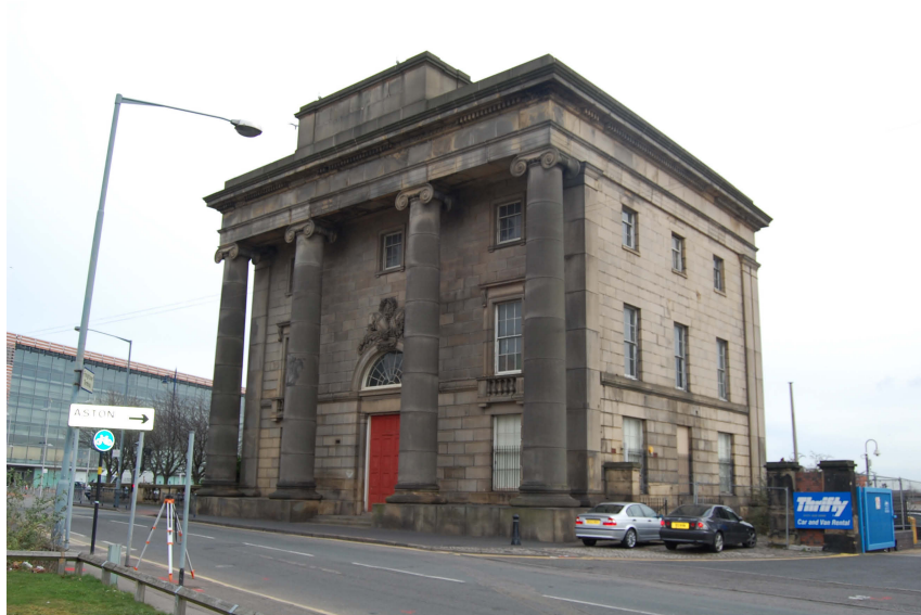
Figure 5.13. Curzon Street Station with Millennium Point in the background, 2007.
