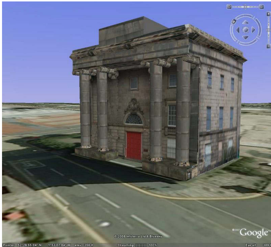
Figure 3.37 Curzon Street station, generated from a 3D laser scan undertaken by Birmingham Archaeology and shown in Google Earth
