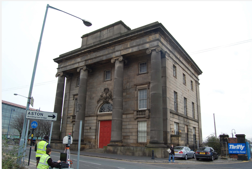
Figure 5.16. Laser Scanning Curzon Street Station
