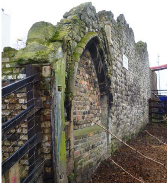
Photo 17 North wall of New Meeting House, Congregational Church
