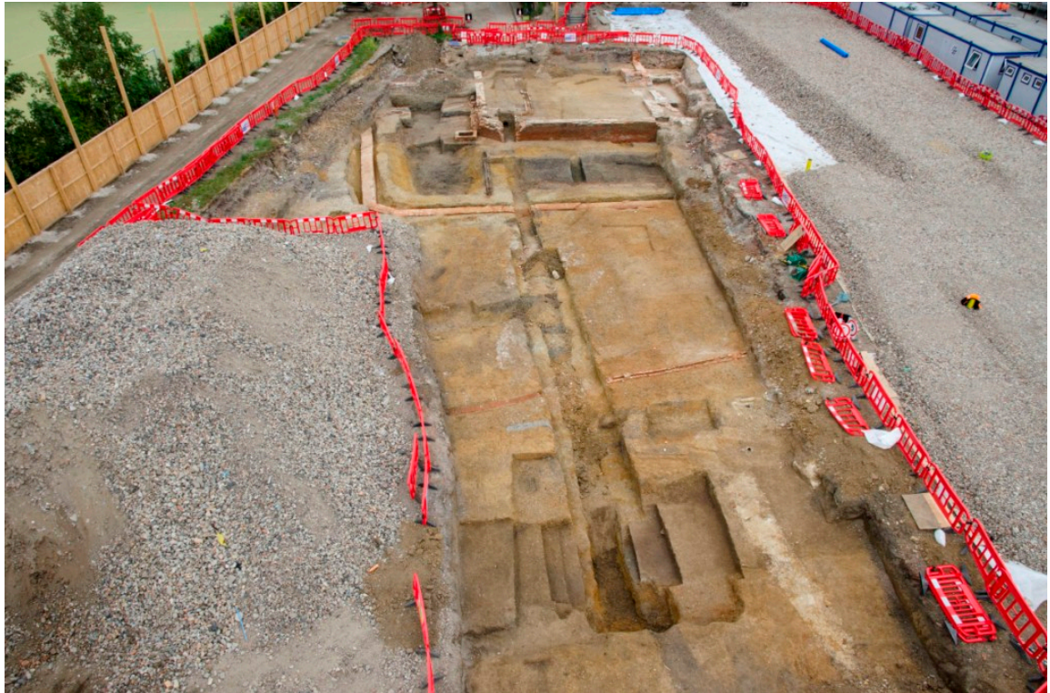
Photo 27 Main shaft excavation with southern arm of L-shaped ditch [284] near, and moated house with bridge baseplate to rear
