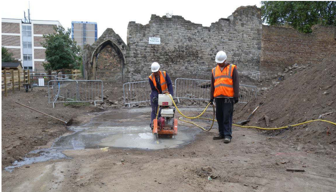
Cutting concrete, Stepney City Farm, looking south
