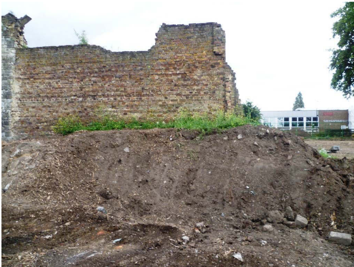
Photo 7 Removal of first metre of modern fill
